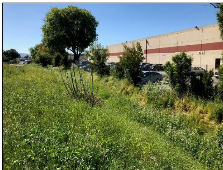
Photo 2. A drainage ditch in the southeastern part of the site.
