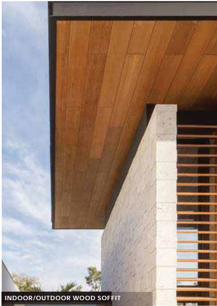
INDOOR/OUTDOOR WOOD SOFFIT
