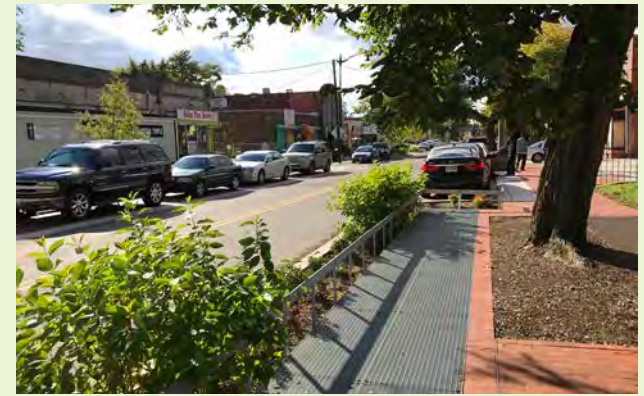
▲ This stormwater curb extension allowed for both a gentle transition in grade and an ADA accessible metal grate to be placed over the landscape to accommodate better pedestrian circulation around the tree.
