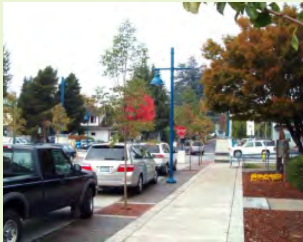
▲ EXAMPLE: A combination of pervious paving and stormwater trees adjacent to the parking lane maximize both space efficiency and stormwater management.
