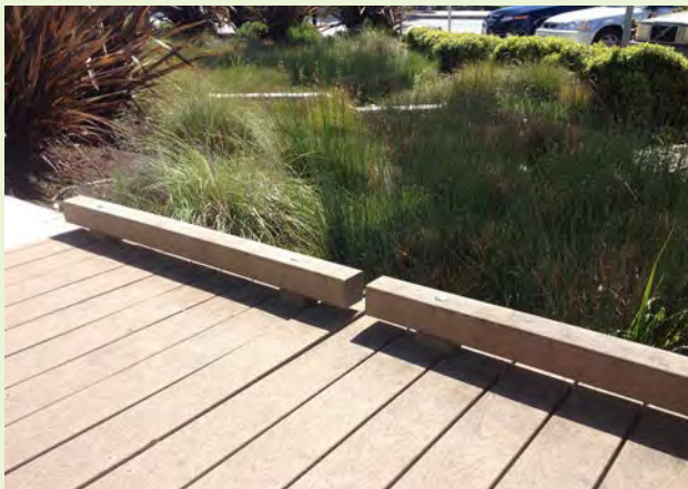
▲ Boardwalks are effective to suspend pedestrian travel over landscaped-based stormwater facilities.
