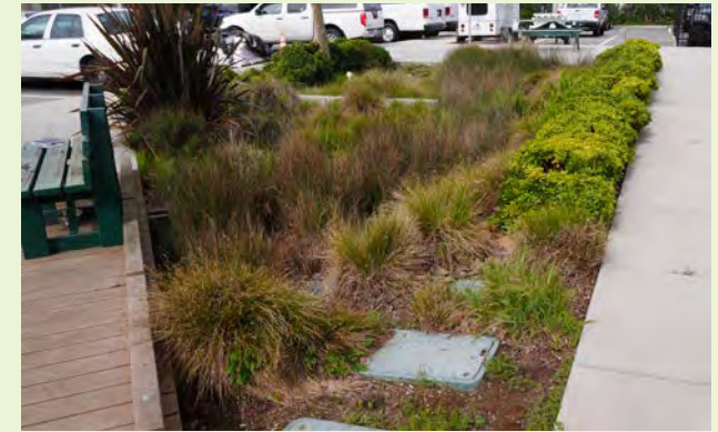
▲ This rain garden has about 70% plant coverage which is considered the minimum for functionality.
