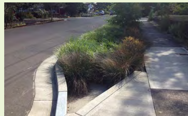
▲ This stormwater curb extension has a concrete forebay that captures sediment that is removed regularly.
