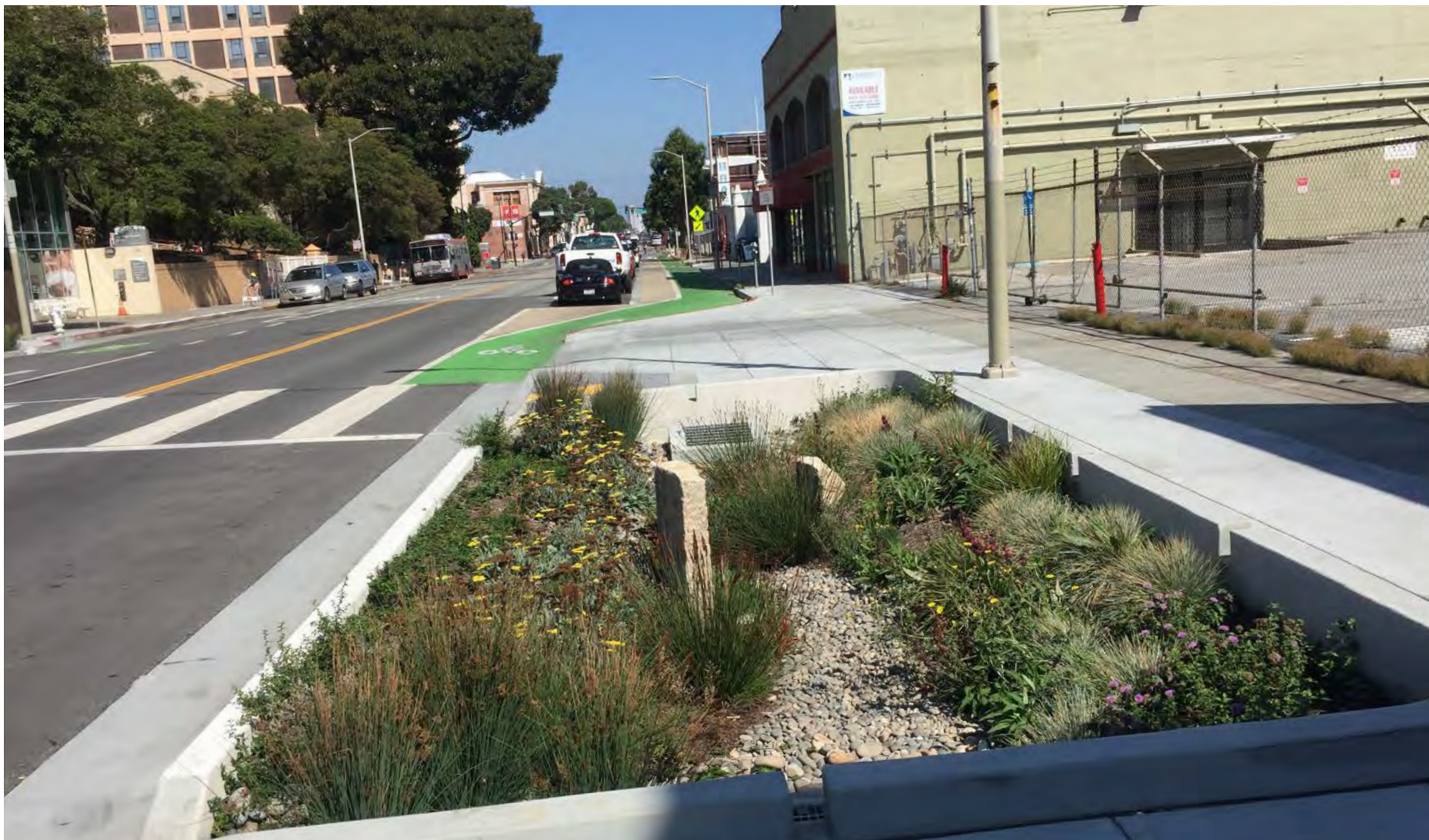
▲ A sustainable street in San Francisco that integrates stormwater planters and stormwater curb extensions with improved pedestrian and bicycle facilities.
