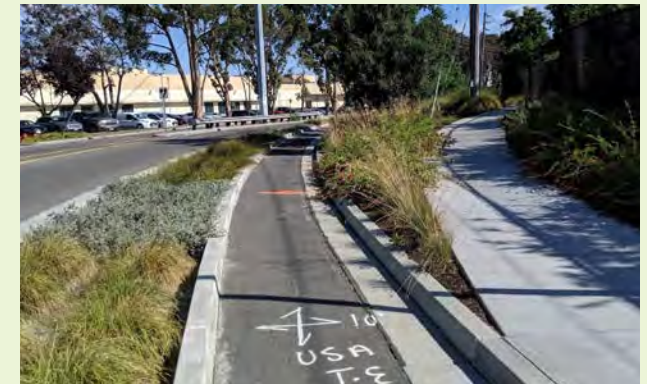
▲ Stormwater planters located between the vehicle travel lane and cycle track provide a buffer between the different transportation models, enhancing bicyclist safety and riding comfort.
