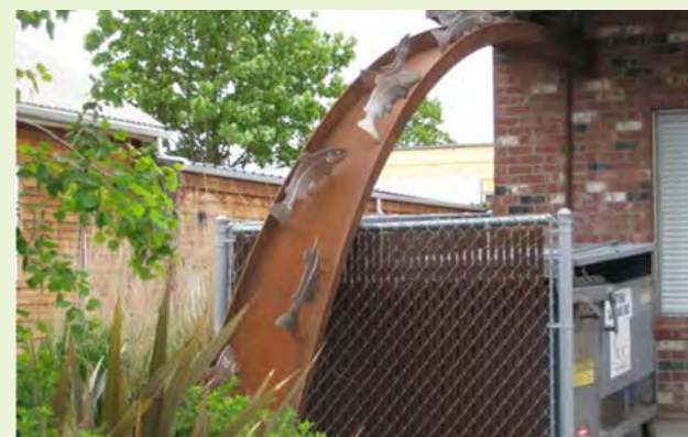
▲ A “fish ladder” conveys roof runoff into a stormwater landscape avoiding the trash receptacle area.
