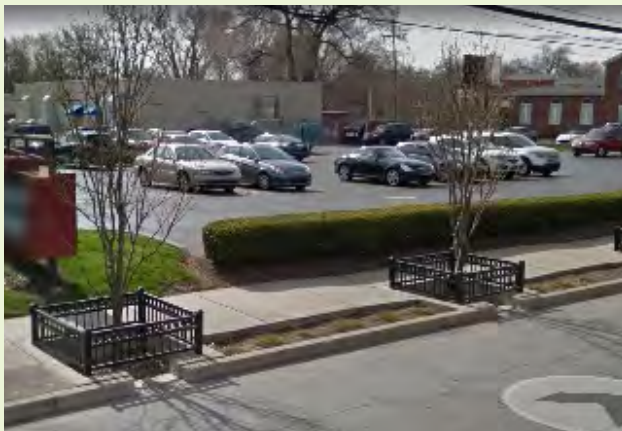
▲ EXAMPLE: This street uses tree well filters linked with pervious paving or landscape areas.
