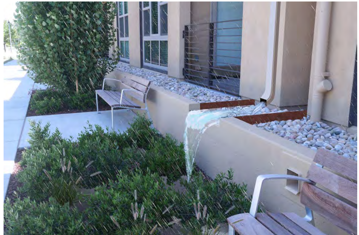
▲ RETROFIT OPPORTUNITY: The same high-density residential yard that disconnects roof downspouts and converts existing landscape areas into a stormwater planter with drought-tolerant landscaping.
