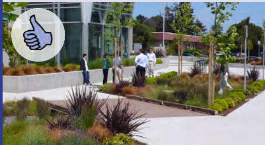
Good, Continue Maintenance Routine
