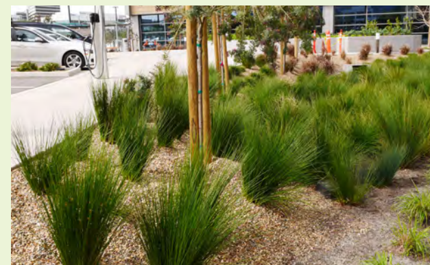
▲ Pea gravel mulch used on both the side slopes and wetted area of a vegetated swale prevents erosion.
