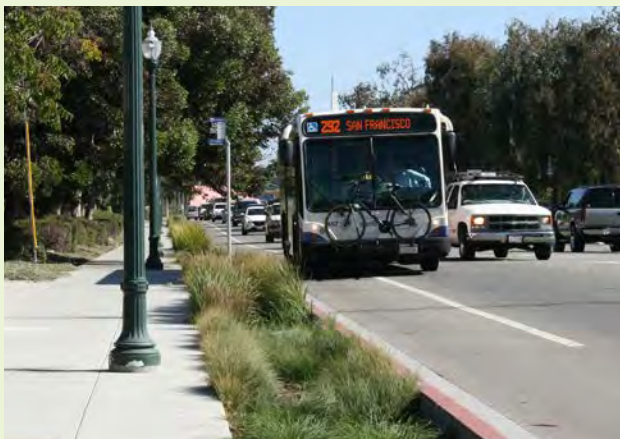
▲ Stormwater planters provide a landscaped buffer between pedestrians and the roadway. Bike lanes provide a designated space for bicyclists, providing a more comfortable cycling experience.
