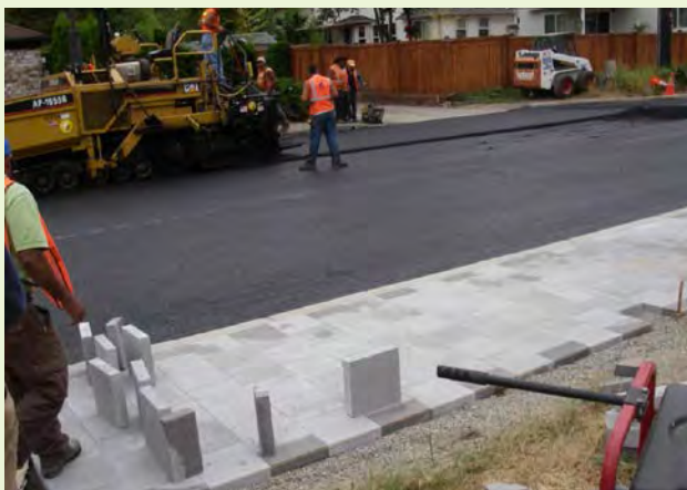
▲ Pervious asphalt and pervious paver sidewalk retrofit.
