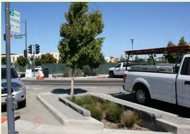
▲ Stormwater planters integrated into diagonal parking planter bays. Step out areas along planter bay edges allow comfortable access to enter and exit vehicles.
