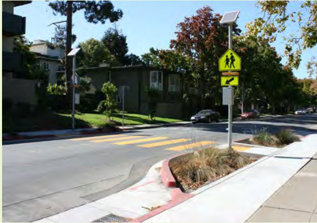
▲ Mid-block stormwater curb extension along this suburban neighborhood connector street with on-demand flashing pedestrian crossing provides a more comfortable and welcoming place to cross.
