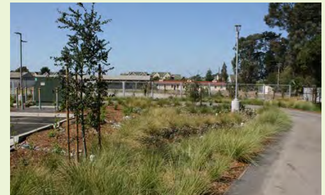
▲ Rain gardens allow for the collection and treatment of larger runoff quantities of stormwater runoff. Runoff from a commercial parking lot and a neighborhood multi-use path flow into this rain garden.
