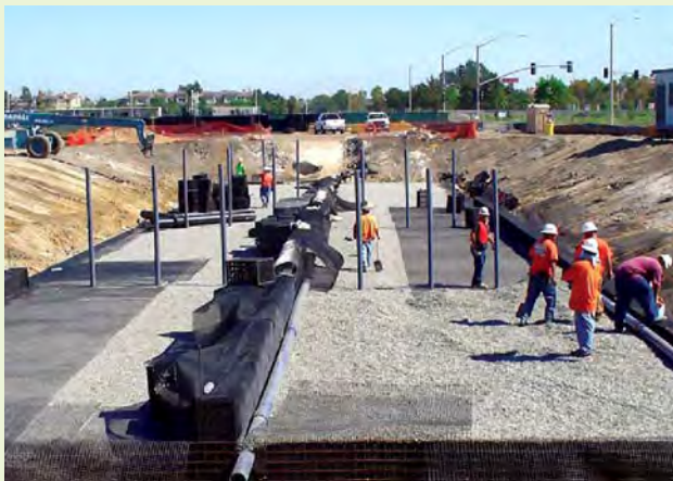
▲ Subsurface infiltration system being placed under a future park.
