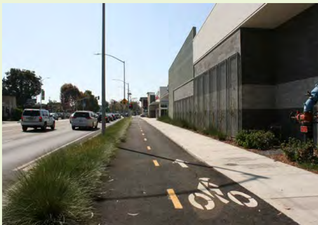
▲ A narrow landscape planter buffers two-way cycle track and a sidewalk from vehicle traffic in this retrofit project along a suburban mixed use thoroughway corridor.
