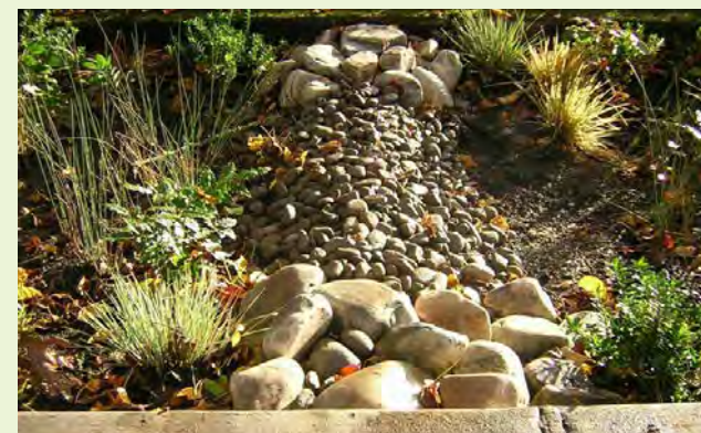
▲ Simple checkdams made of stacked rocks or gravel can be used on gently sloped stormwater facilities.
