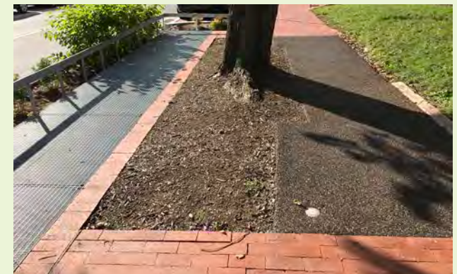
▲ To preserve an existing street tree and provide space for a stormwater curb extension, a metal grate extends the walkway over the new landscape area.
