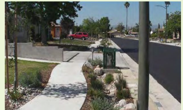
▲ AFTER: The Elmer Avenue Neighborhood is retrofitted with stormwater planters that collect and pass stormwater through a catch basin and infiltration gallery. The addition of street trees, sidewalks, and street lighting enhance neighborhood safety and connectivity.
