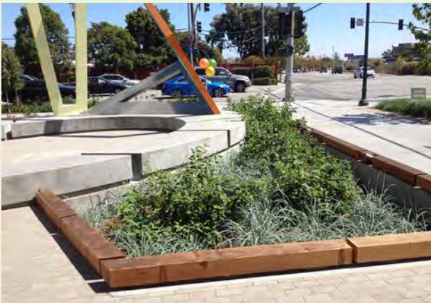
▲ This urban rain garden at a street corner features a well-integrated raised timber edge treatment for detecting a drop in grade.
