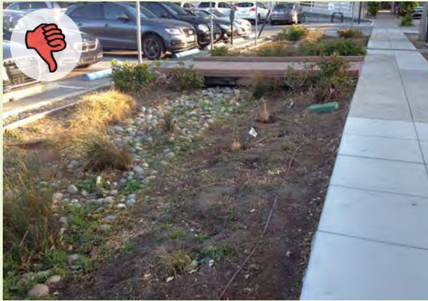
▲ This vegetated swale contains less than 70% coverage of plant material and needs additional plant material added.
