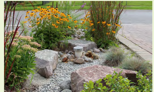
▲ Infiltration trench with plantings located in a low density residential setting.
