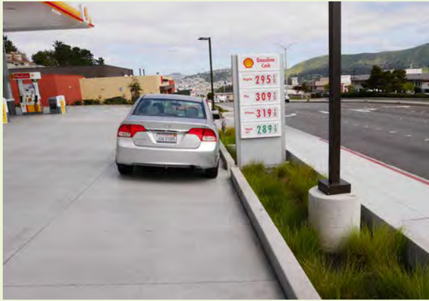
▲ This gas station parking lot in San Mateo County provides a stormwater planter within a confined space used for capturing runoff.
