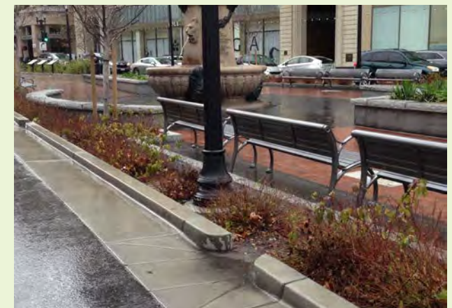
▲ While this plaza retrofit project was not required to provide green infrastructure, curb cuts were designed into the project to allow street runoff to enter depressed landscape areas to provide some water quality treatment and debris catchment.
