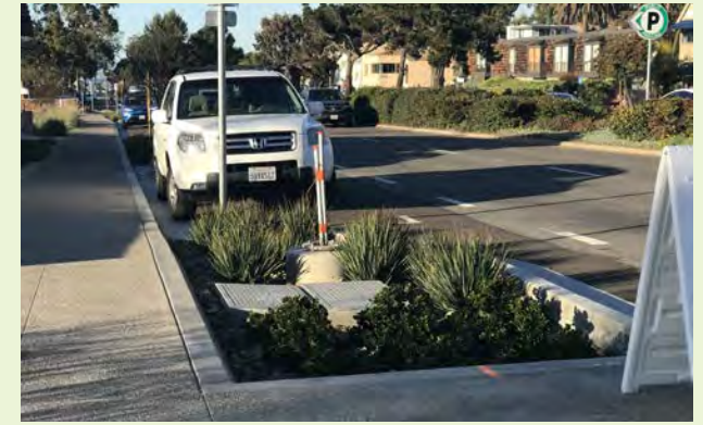
▲ These stormwater curb extensions have been designed to have street lights and their electrical boxes within the planters. Even though this was a retrofit project the sidewalk, curb, and gutter are new and the utility boxes could have been moved into the sidewalk.
