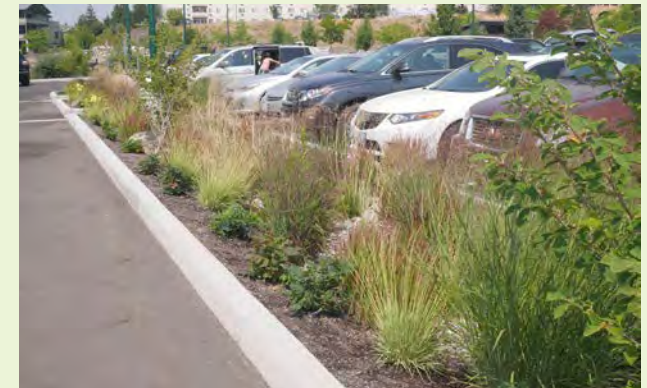
▲ Parking lot vegetated swales, like this example in Coeur d'Alene, Idaho provide a visual buffer between parked cars.
