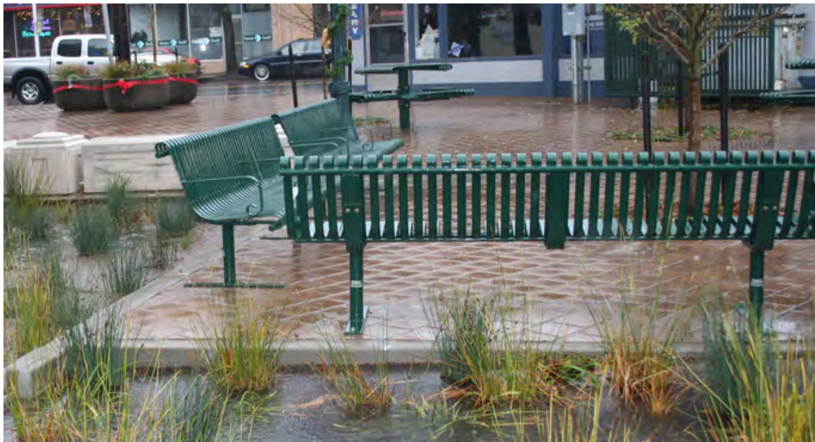
▲ Sheet flow of stormwater runoff enters a stormwater planter from a public plaza space.
