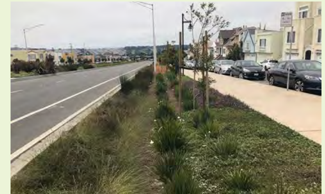
▲ Stormwater planters can be retrofitted into street projects to meet multiple community goals including climate resiliency and adaptation, and integration of multimodal facilities.
