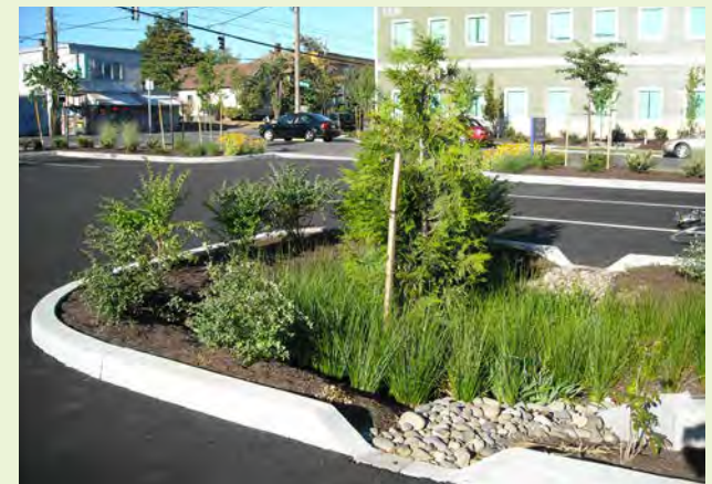
▲ EXAMPLE: This parking lot treats its stormwater runoff within multiple stormwater swales throughout the site.
