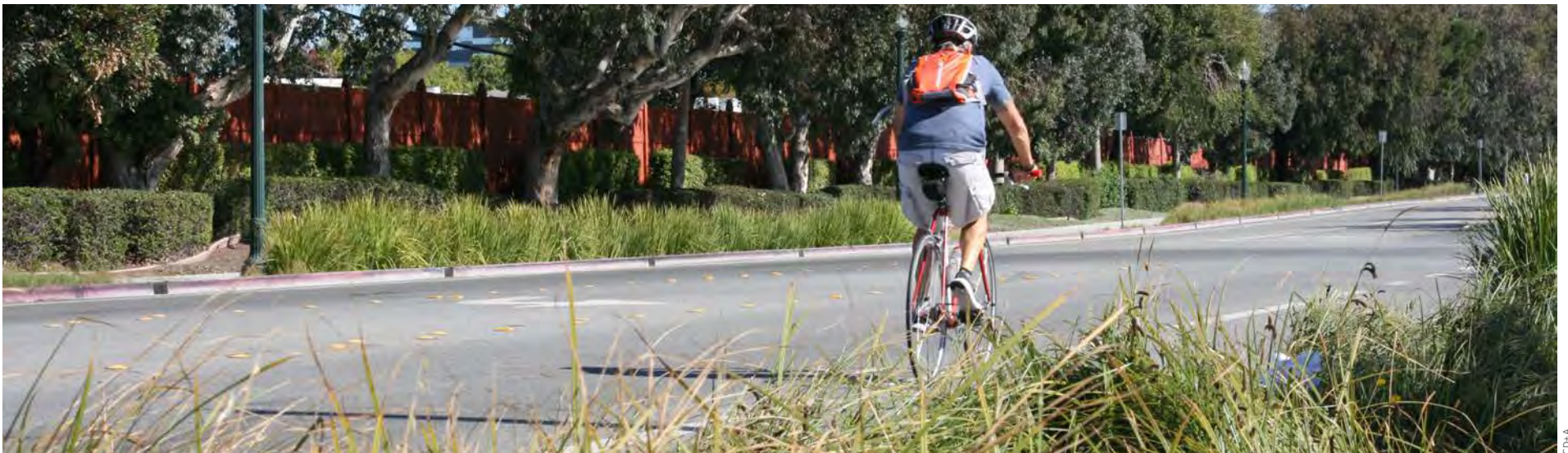
▲ A sustainable street retrofit project along Humboldt Street in the City of San Mateo includes bike lanes and stormwater planters along a commercial and residential corridor.
