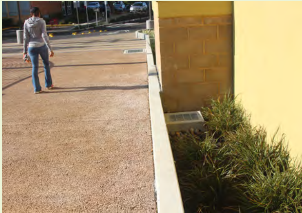
▲ This multi-family project uses porous asphalt in this pedestrian walkway that doubles as a fire lane, and complements the adjacent stormwater planter that treats building rooftop runoff.
