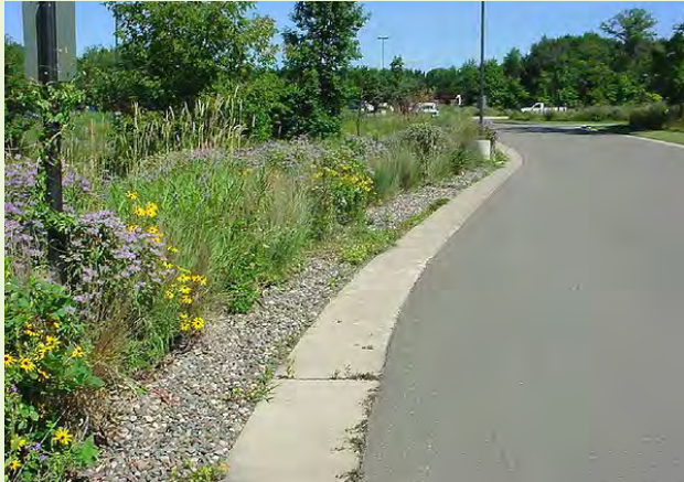
▲ Infiltration trench along curbless street which allows sheet flow to enter the facility.
