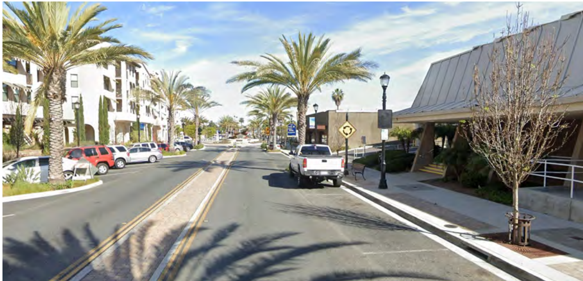
▲ This is a retrofit project in which the street was redesigned to drain to the center permeable paver median and to the curbs with tree wells designed with a modular suspended pavement system.
