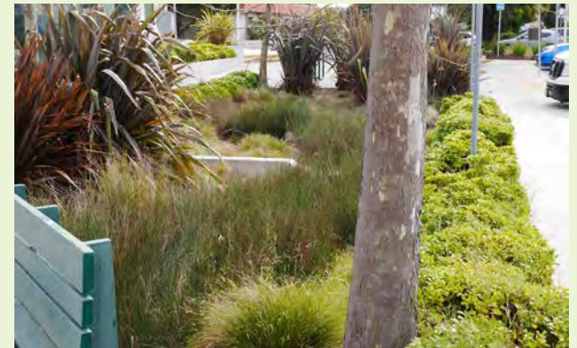
▲ This parking lot rain garden in San Mateo County utilizes the “Condition 3” cross section. The soil is very clayey but does have an underdrain and storage layer, hence the cross section retains 6 to 8 inches of runoff.
