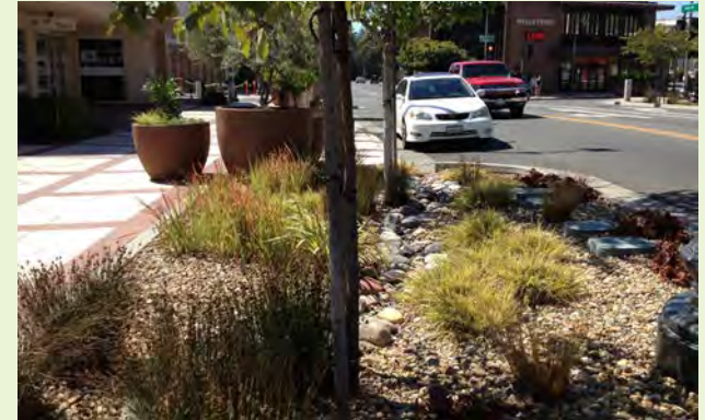
▲ Conversely, this stormwater curb extension features street trees located in the center of the landscape area and flush with the facility bottom. There is no mounding of the rootball area.
