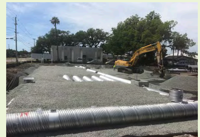
▲ Subsurface infiltration system being placed under future parking lot.
