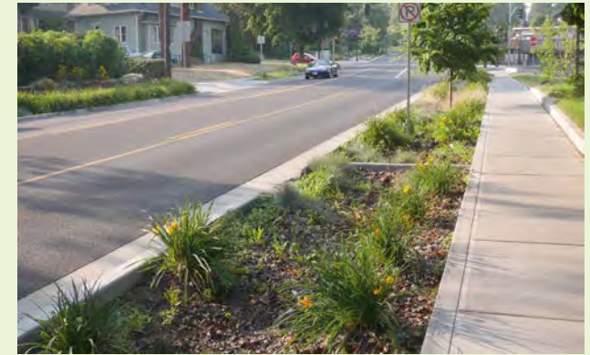
▲ A beautiful vegetated swale adds significant greening and character to a residential street.
