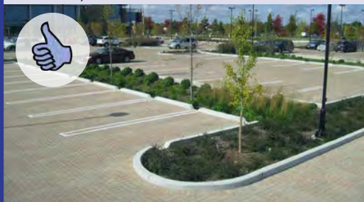
Good, Continue Maintenance Routine
