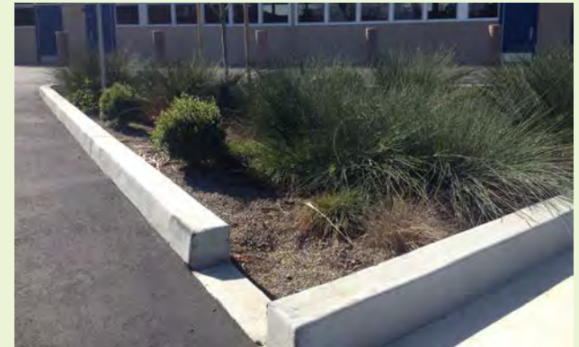
▲ This parking lot rain garden in San Mateo County utilizes the “Condition 2” cross section. The soil is very clayey with no underdrain; hence the cross section is quite shallow.
