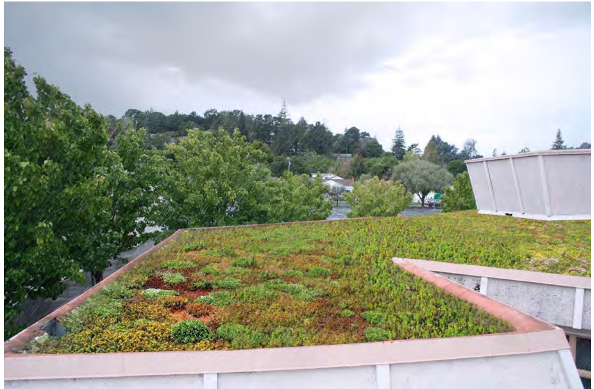
▲ RETROFIT OPPORTUNITY: The same school rooftop retrofitted with an extension green roof system.
