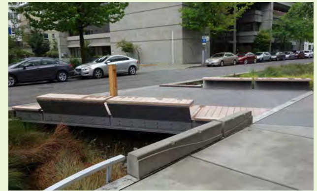
▲ Bridges over green infrastructure, such as this one connecting the street to the sidewalk and multi-family project entry, can be designed to be significant gateways and gathering places for people within the public realm.
