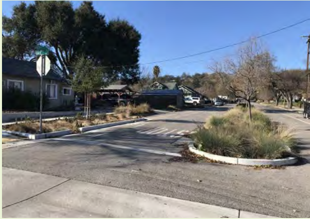
▲ Stormwater curb extensions and a median stormwater planter along with striped bike lanes have been retrofitted into this semi-rural neighborhood.
