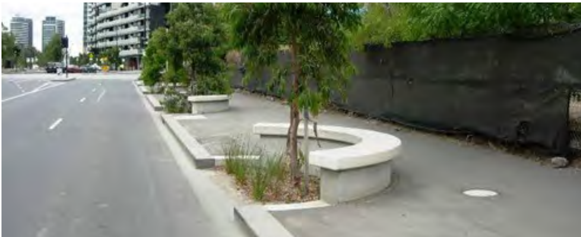
▲ These stormwater trees are flanked by seating areas. A metal capped inlet should be provided across the face of the planter to prevent vehicles from entering the planters.
