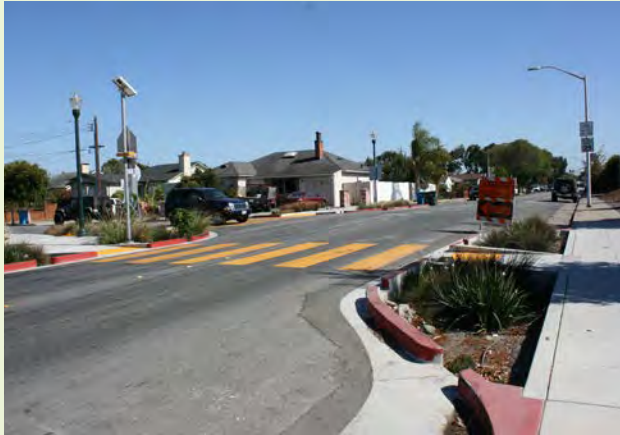
▲ Corner and mid-block curb extensions create a safer and more attractive pedestrian crossing. On-demand flashing lights and a high visibility crosswalk provide additional complete street techniques, while stormwater curb extensions add a green infrastructure component.
