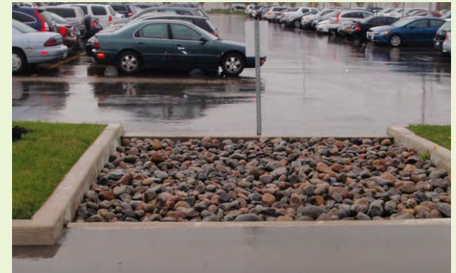
▲ This infiltration trench absorbs runoff from the parking lot.
