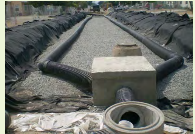
▲ Subsurface catch basin and infiltration gallery infrastructure installed under Elmer Avenue.
