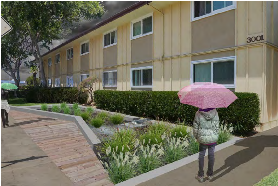
▲ RETROFIT OPPORTUNITY: The same high-density apartment complex that converts perimeter grass and landscape areas into a rain garden with drought-tolerant landscaping. Roof downspouts direct water into the rain garden.
