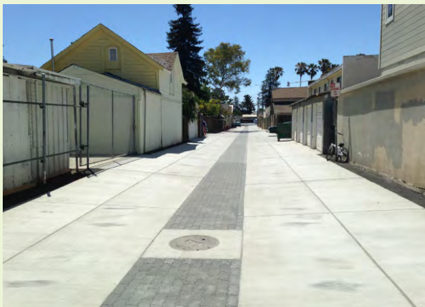
▲ EXAMPLE: The Martha Gardens neighborhood in San Jose was retrofitted with three green alleys. Runoff flows to a central panel of pervious pavers over an infiltration trench to reduce localized flooding and improve water quality.
