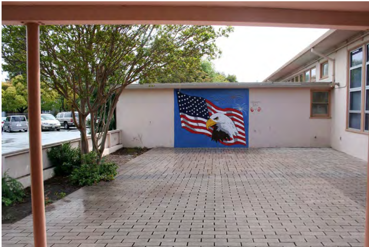
▲ RETROFIT OPPORTUNITY: The same school courtyard using pervious pavers to allow for rainfall to soak into the ground.
