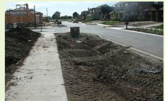
▲ Compost should be cultivated into native soil as recommended by the soil laboratory analysis report.
