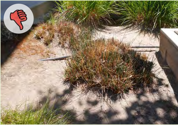
▲ A rain garden with compacted soils cannot maintain long term function.
