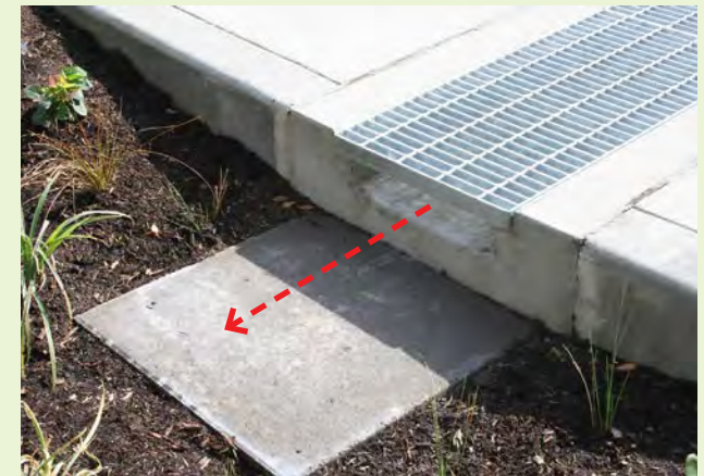
▲ A concrete unit paver is placed at the exit point of this trench drain. The pad helps prevent erosion by dissipating water velocity as water drops from the trench drain to the finish grade of the stormwater facility.
