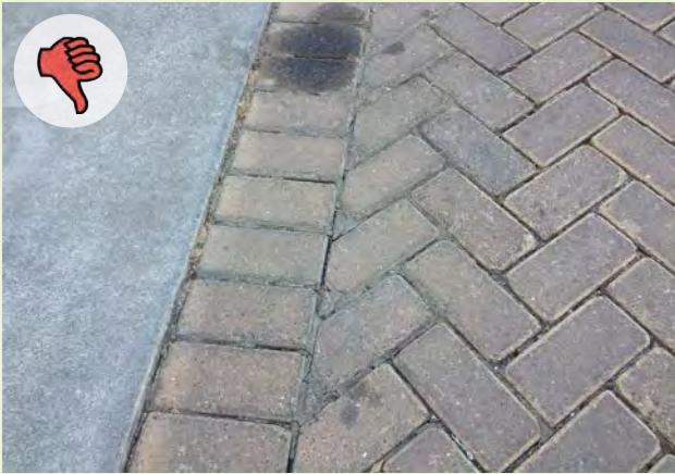
▲ Sediment build-up within the joints of interlocking concrete pavers.
