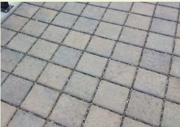
▲ The void space of pervious concrete should be free of sediment and debris by regular sweeping or blowing.
