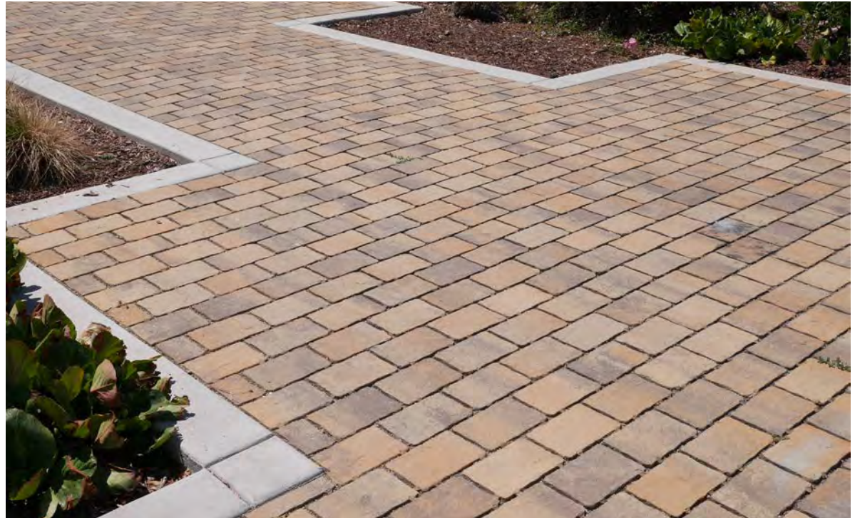
▲ An apartment complex in San Mateo uses permeable pavers throughout the walkway system.
