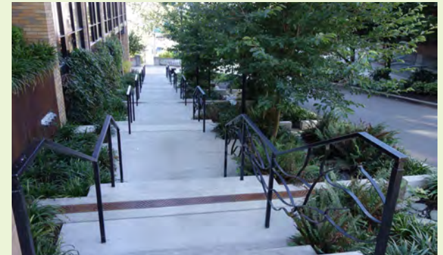
▲ In highly developed projects, rainfall captured from roofs can be directed to building adjacent stormwater planters for treatment. Weirs allow the system to step down the sloping ground plane.
