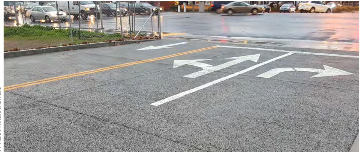
▲ This project uses pervious concrete to manage runoff from the street.
