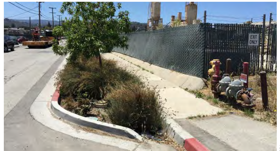
▲ This industrial street, Bransten Road in San Carlos, also underwent a street retrofit to integrate stormwater curb extensions.
