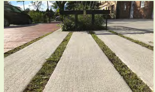
▲ Flexibility in design standards allowed this street project in Washington D.C. to design, construct, and test innovative “Landscape Infiltration Gaps (LIGs)” to capture sidewalk runoff.
