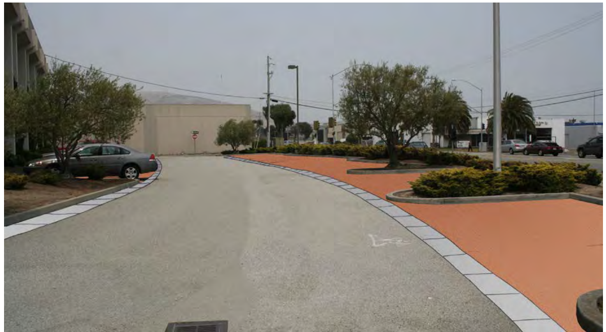
▲ RETROFIT OPPORTUNITY: The same parking lot retrofitted with pervious pavement in the parking stalls.
