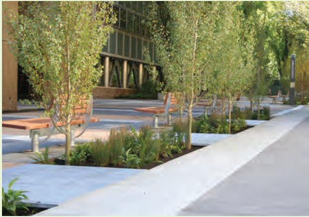
▲ This is a flow-through and lined stormwater planter in a pedestrian plaza space that still allows for street trees.
