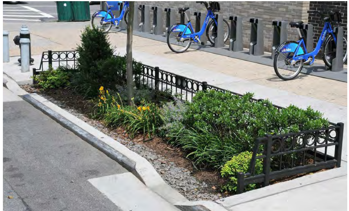
▲ Stormwater trees increase a community's urban forest while also achieving stormwater management goals.
