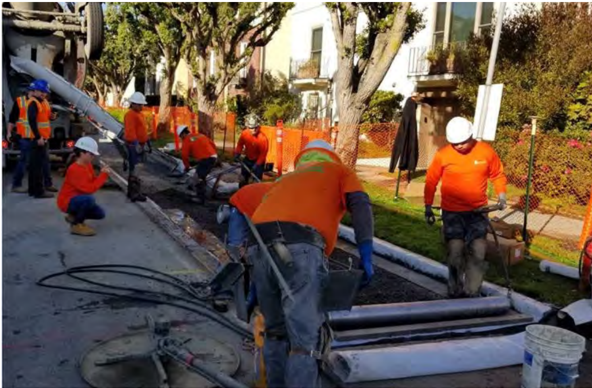
▲ The parking lane in this San Francisco residential street is being retrofitted with pervious concrete.
