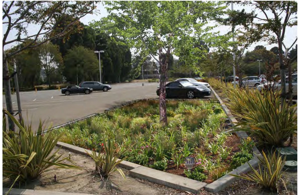
▲ RETROFIT OPPORTUNITY: The same parking lot retrofitted with a stormwater planter. Notice that this stormwater planter is located near the existing drainage inlet.
