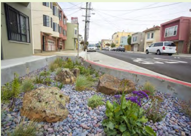
▲ The use of gravel as a mulch in this stormwater curb extension also helps control water velocity.
