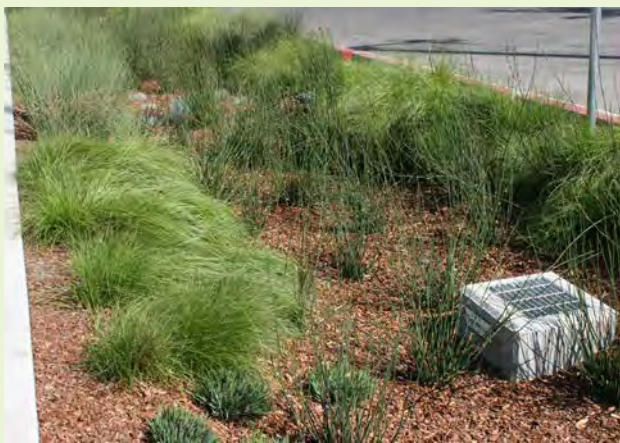
▲ Overflow structure set above ponding level, but below adjacent walkway and street.
