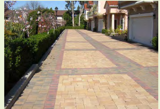
▲ Residential driveway with permeable pavers in San Mateo County.
