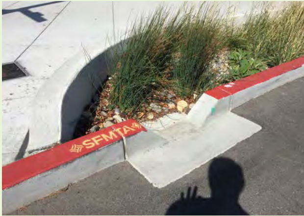
▲ A concrete splash pad to catch sediment and cobbles to dissipate runoff velocity aid in the longevity and maintenance of the facility.
