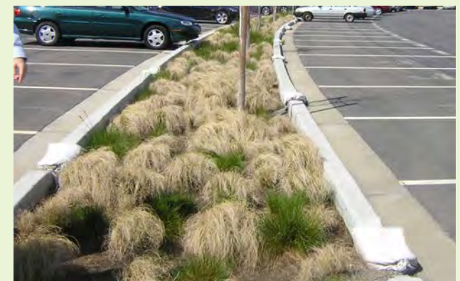
▲ Sand bags are placed in front of curb cut inlets in order to help protect soil and plant material immediately after planting.
