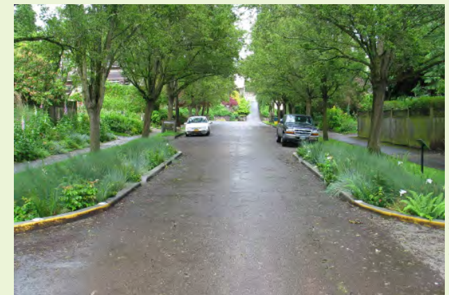
▲ EXAMPLE: A pair of stormwater curb extensions used in a residential street's parking zone. Notice that there is still plenty of on-street parking available.
