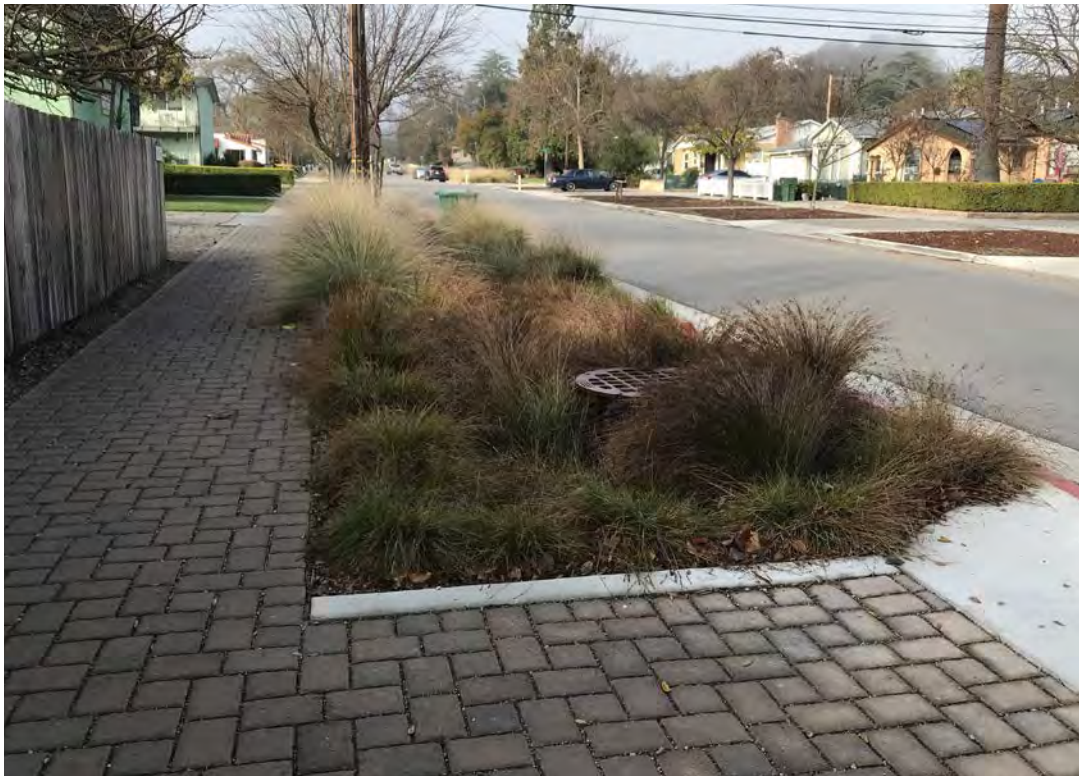
▲ Stormwater planters and permeable pavers are used in this retrofit street project that reduced the wide width of the roadway, enhances the low density residential neighborhood character, and manages runoff.
