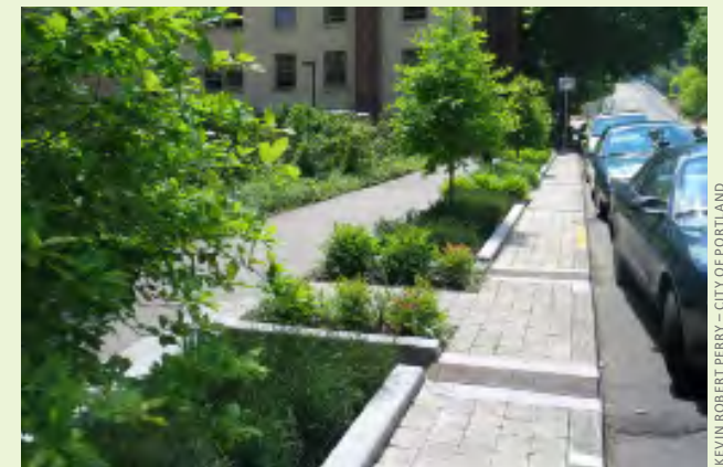
▲ EXAMPLE: Stormwater planters used along a downtown street. Notice that there is adequate space allocated for people to get in and out of their vehicles and access the sidewalk and frontage uses.
