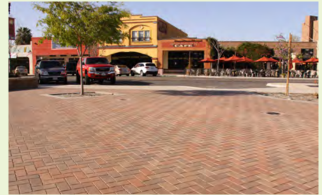
▲ This plaza is made up of permeable pavers, allowing water to infiltrate at the source.
