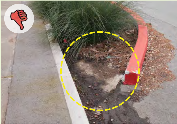
▲ A stormwater curb extension curb cut full of sediment accumulation.
