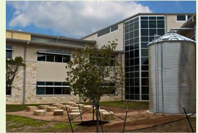
▲ EXAMPLE: A large 15,000 gallon cistern at Lake Travis Middle School near Austin, Texas is used for landscape irrigation.
