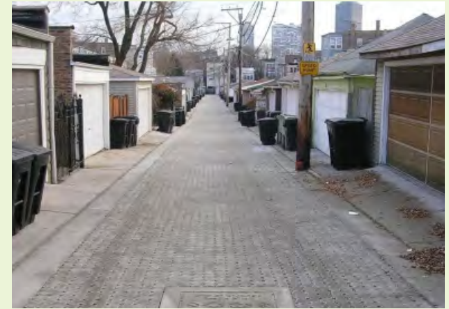
▲ EXAMPLE: This neighborhood alley uses pervious pavers across the entire alley to manage and treat stormwater.
