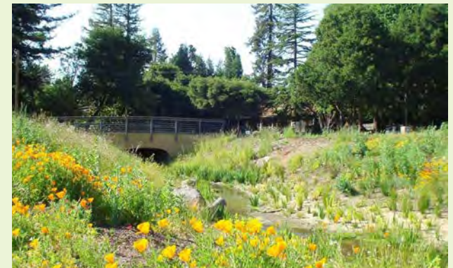
▲ A portion of Sausal Creek was daylighted with the Portola Valley Town Center project. The restored creek design slows and helps treat stormwater runoff, protecting the creekbed from erosion and sediment pollution.
