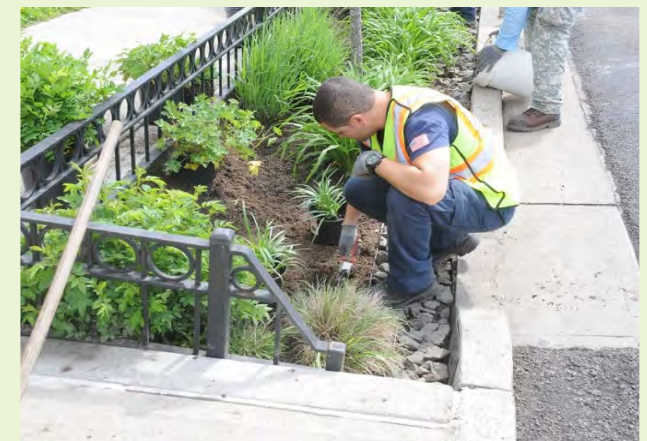
▲ As with other green infrastructure measures, stormwater tree planters will need to be maintained to remove debris and sediment and replant vegetation that declines.
