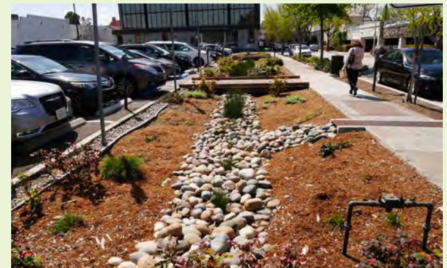
▲ Plants within this rain garden have died due to excessive drought conditions and need to be replanted.
