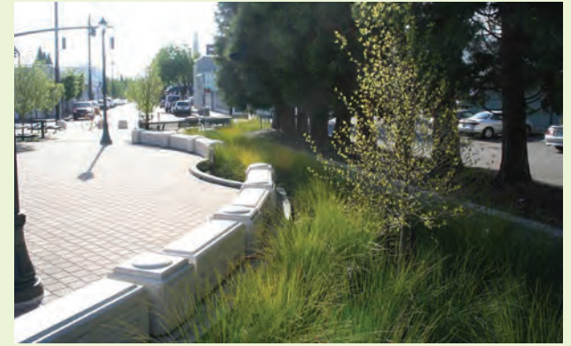
▲ This plaza rain garden in Portland, Oregon utilizes the “Condition 1” cross section. The soil is sandy loam; hence the cross section retains 6 to 8 inches of runoff without an underdrain.
