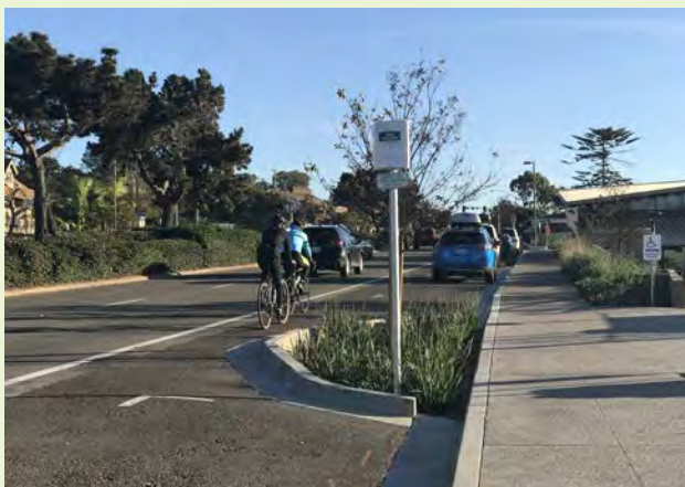
▲ A stormwater curb extension provides attractive green space at this location between on-street parking stalls. A 2-3" rock gravel mulch helps to dissipate runoff flows on this sloping street condition.
