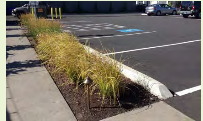
▲ This narrow green gutter has an integrated curb with frequent curb cuts to allow parking lot runoff to enter the landscape.
