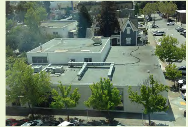
▲ EXISTING: A typical commercial/office building rooftop in San Mateo County.
