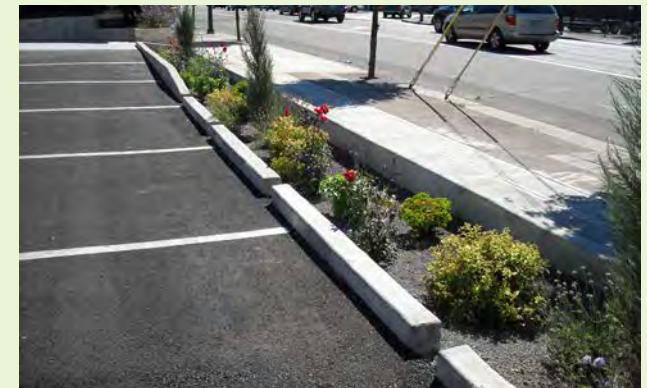
▲ A narrow stormwater planter at the edge of a parking lot.
