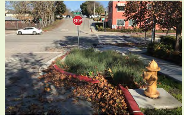
▲ A stormwater curb extension with weirs was added to this sloped residential street.
