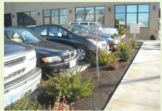
▲ EXAMPLE: A shallow green gutter accepts runoff from the adjacent parking lot surface.
