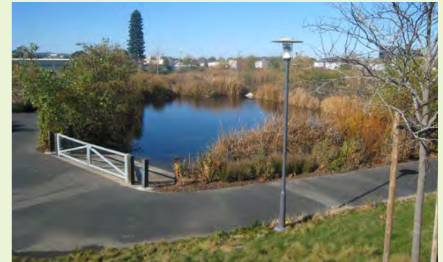
▲ A constructed wetland pond in San Mateo collects and treats stormwater from surrounding neighborhoods.
