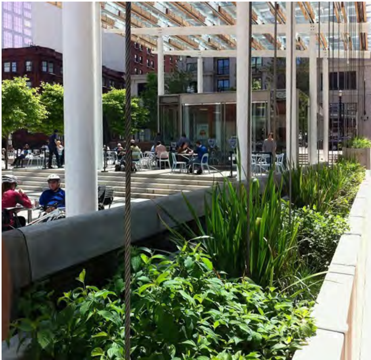
▲ This large stormwater canopy in Director's Park in Portland, Oregon directs runoff down vertical cables and into a raised stormwater planter.
