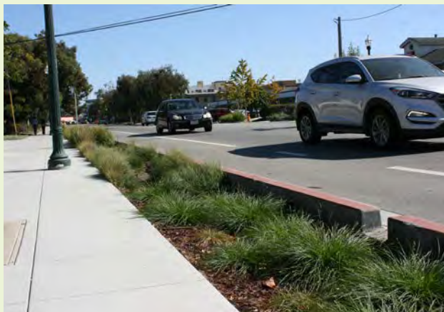
▲ This arterial street without on-street parking was retrofitted with a series of stormwater infiltration planters.
