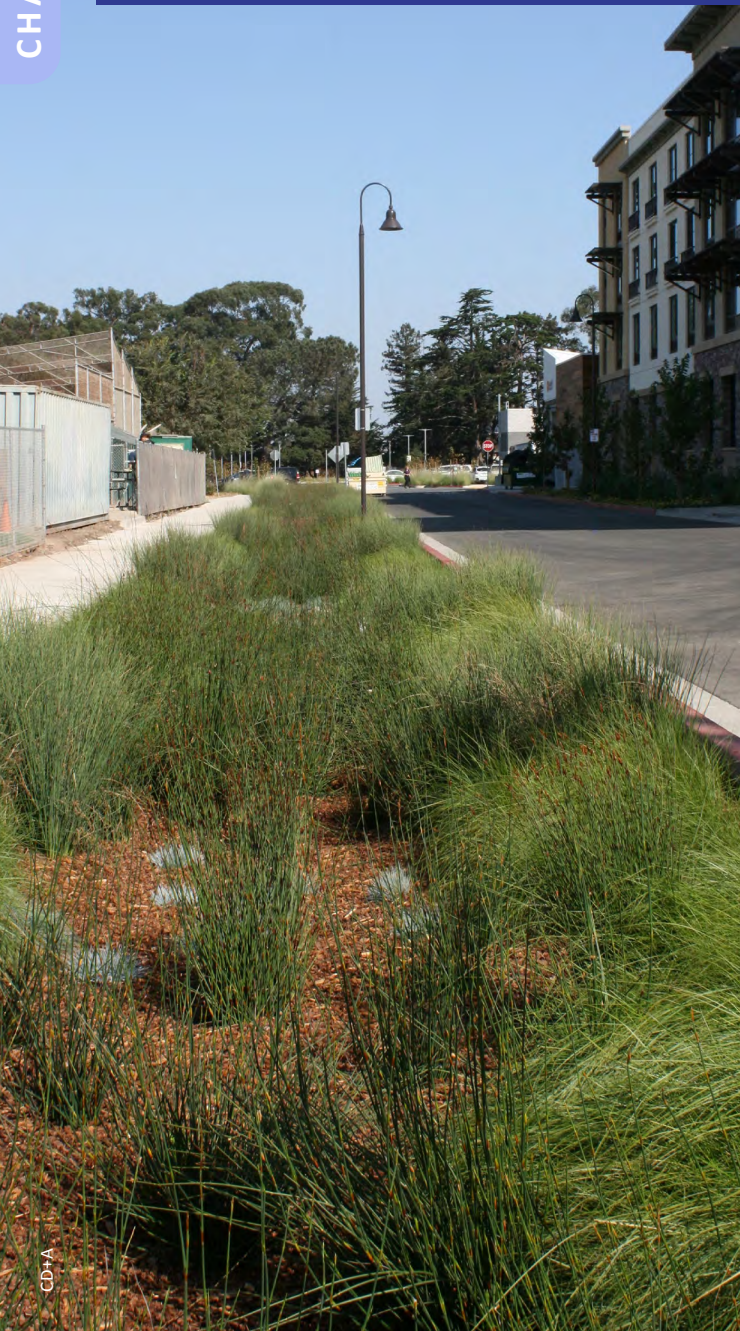
▲ Typical vegetated swale in a constrained right of way. This concept shows a design option in locations where less space is available and no step-out space is required.
