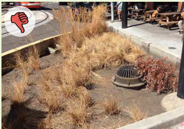
▲ Poorly performing irrigation can also quickly cause plant death from under-watering or lack of coverage.
