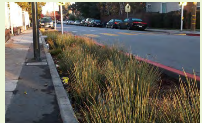
▲ This stormwater curb extension has a hybrid of both pea gravel below the flow line of water and organic mulch along the side slopes that are above the flow line of water.
