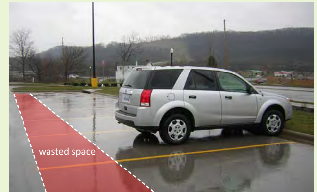
▲ By transferring this area of wasted space to the front row of parking stalls, a vegetated swale could fit without affecting the function of the parking lot.
