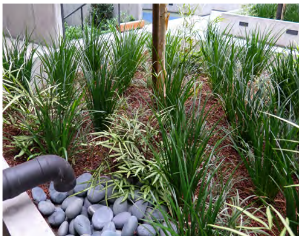
Bioretention in a plaza manages stormwater from the roof of a residential building in San Francisco. Photo: Krystal Zamora
