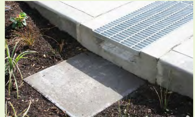
▲ A concrete forebay at the street curb cut is placed lower than the gutter grade to disperse water flow.
