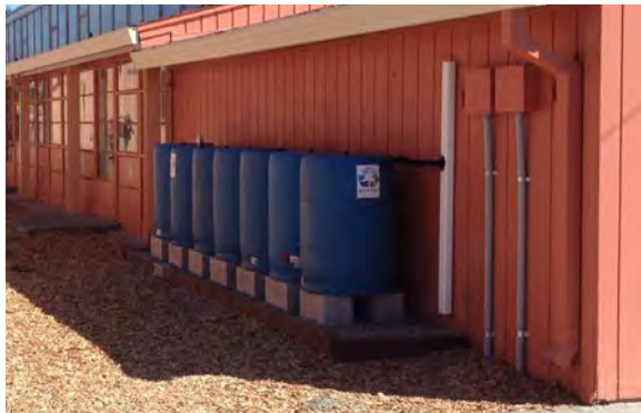
▲ A series of interconnected rain barrels captures roof runoff for reuse at an elementary school.
