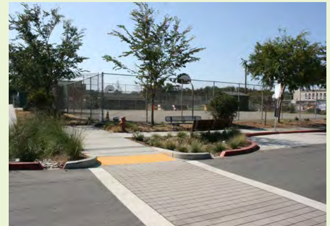
▲ While these stormwater curb extensions have been designed to be fairly deep in relation to the surrounding walkways and roadway, the vegetation is densely planted and fairly tall, which helps discourage people from entering them.
