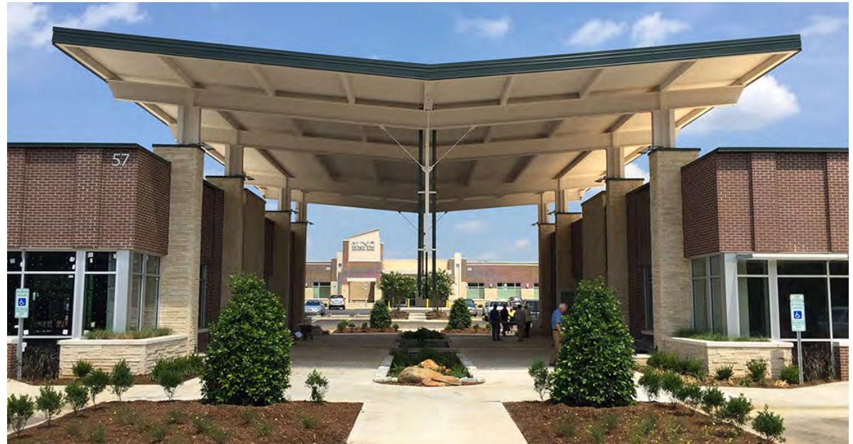
▲ This large stormwater roof canopy at the Chatham Park Medical Facility in North Carolina captures and directs runoff into the surrounding landscape.
