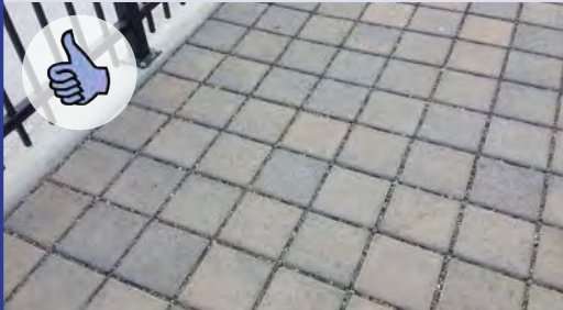
Good, Continue Maintenance Routine
