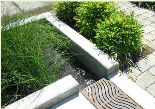
▲ Grated curb cuts conveying street runoff should be at least 12 inches wide, preferably 18 inches wide to adequately handle stormwater flow.
