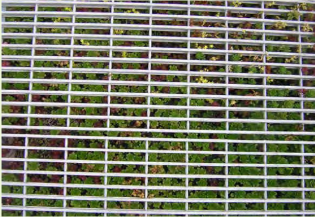
▲ This metal grate allows for pedestrian travel over a landscaped system while still allowing rainfall to pass through the void space between metal grate paving.
