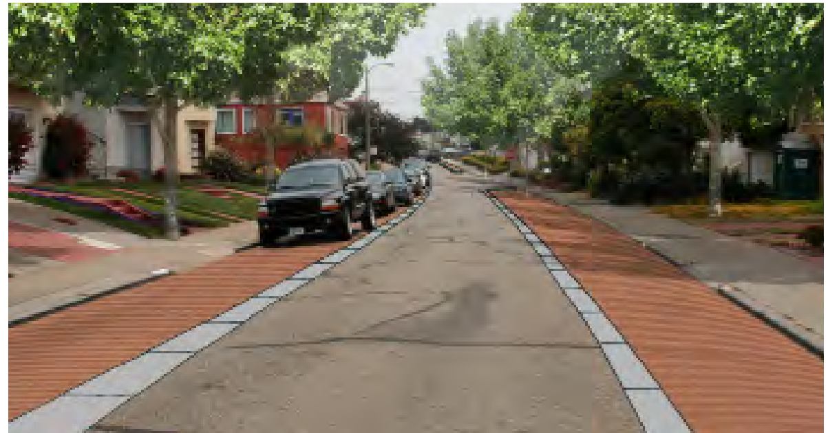
▲ RETROFIT OPPORTUNITY: The same neighborhood access street retrofitted with pervious paving in the parking lanes of the street as well as street trees within front yards.
