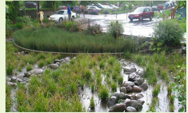
▲ This rain garden next to an elementary school collects runoff from adjacent neighborhood streets and the school's parking lot.
