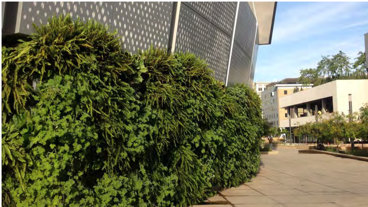
▲ A large green wall wraps around the Golden One Center in Sacramento. This green wall captures runoff from vertical surfaces and helps soften the overall feel of the space.
