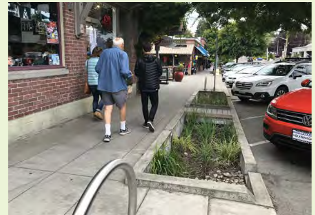
▲ Green infrastructure included in commercial retrofits treat runoff at its source and beautifies the public storefront and streetscape, creating a more inviting atmosphere for tenants and patrons.
