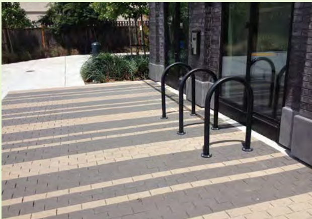
▲ EXAMPLE: A high-density residential building uses pervious pavers at bike parking zones.
