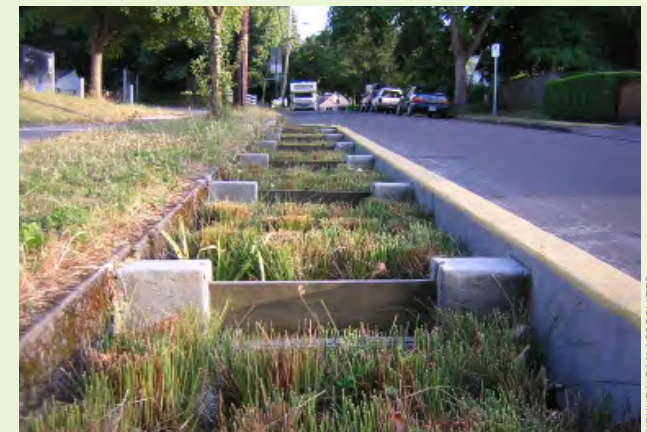
▲ EXAMPLE: This neighborhood connector incorporates a stormwater curb extension with check dams to reduce velocities on a sloping street.
