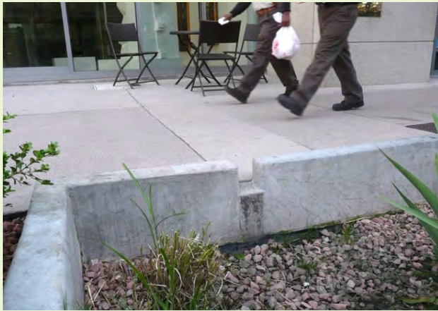
▲ Low curb edge with gaps to allow runoff to enter bioretention area.
