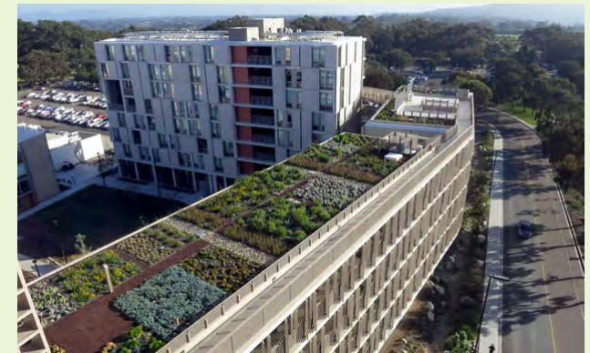
▲ This university dorm building at UC San Diego features a larger extensive green roof.
