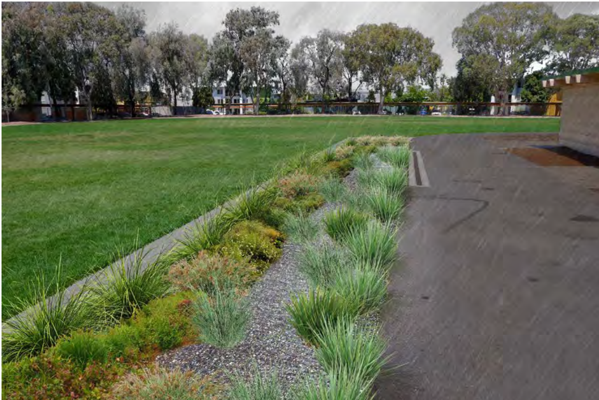
▲ RETROFIT OPPORTUNITY: The same park and walkway condition with a vegetated swale replacing a portion of the lawn space.
