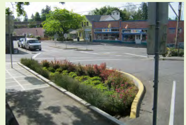
▲ EXAMPLE: This main street retrofit consolidated a few parking spaces and incorporated an angled stormwater curb extension.
