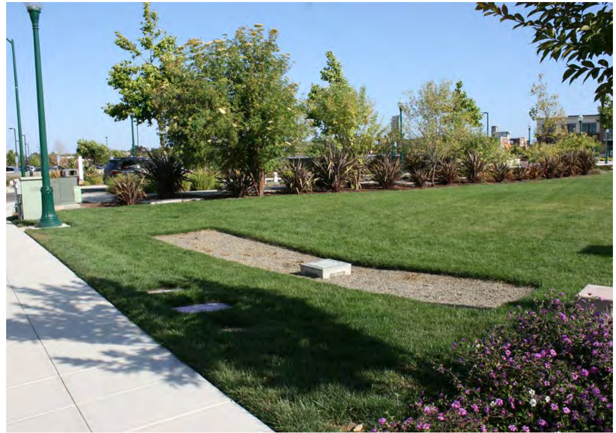
▲ Infiltration trench placed behind sidewalk within a park.
