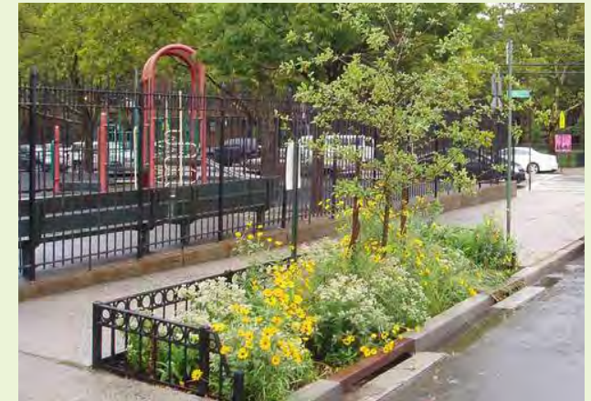
▲ Stormwater tree planters can vary in length, but are typically shorter than this example. Note that this example uses metal capped inlets to keep vehicle tires from entering the planter.
