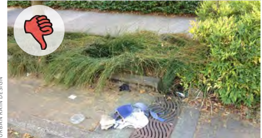
Poor, Overhaul Maintenance Routine
