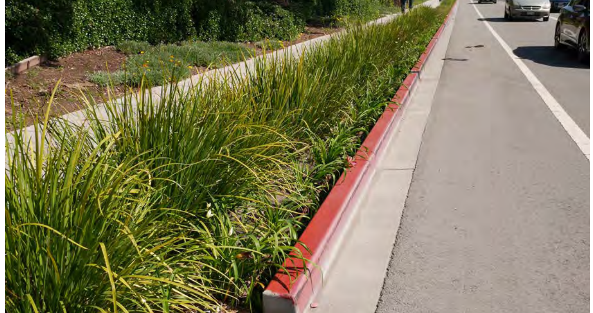
▲ This shallow vegetated swale along Delaware Avenue in San Mateo captures stormwater runoff and buffers pedestrians from vehicular traffic.
