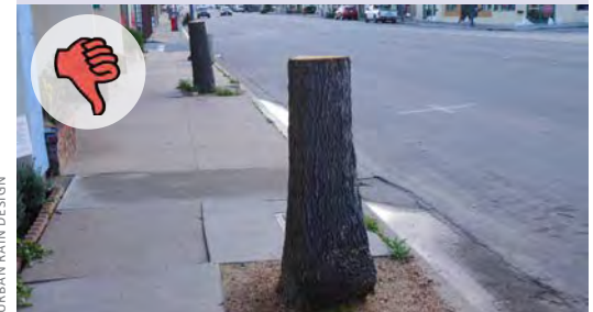
Poor, Overhaul Maintenance Routine
