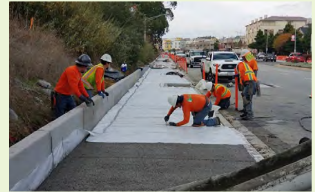
▲ This pervious concrete sidewalk is being retrofitted along El Camino Real in South San Francisco.
