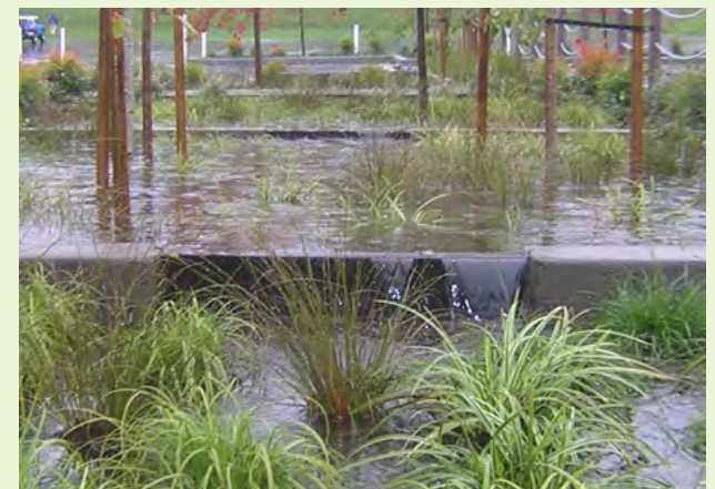
▲ Stormwater facilities slow the flow of stormwater runoff through the interaction of the water with plants and soil.
