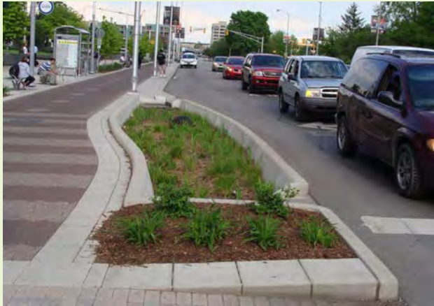
▲ A combination of pervious pavers and a stormwater curb extension manages runoff and protects riders on this cycle track and pedestrians at the intersection.
