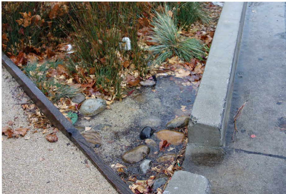
▲ Remove sediment and debris as needed to maintain the function of the green infrastructure.
