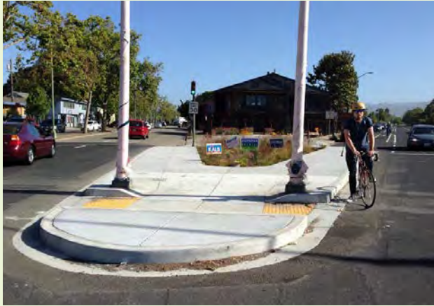
▲ This street retrofit features a rain garden, a bulbout for a protected pedestrian crossing area, and two streetlights that form a gateway feature.
