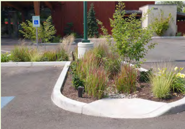
▲ This parking lot features distributed landscape spaces within the interior of the parking lot to capture stormwater runoff.
