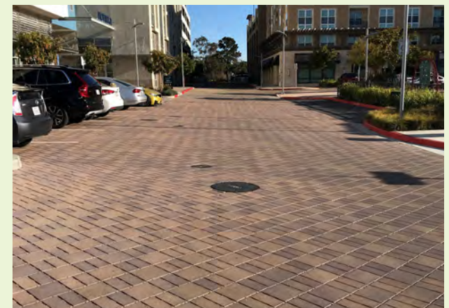
▲ Streets and parking lots cover a large percentage of the built environment. Pervious pavements such as these permeable pavers can aid in providing drivable and walkable surfaces that treat and infiltrate runoff.
