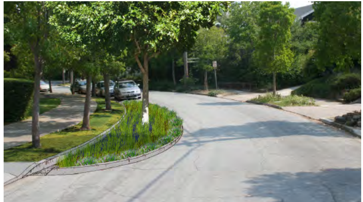
▲ RETROFIT OPPORTUNITY: The same neighborhood street retrofitted with mid-block stormwater curb extension, as well as an additional street tree.
