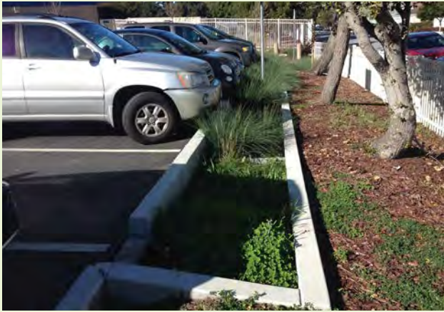
▲ This stormwater planter captures stormwater runoff at the perimeter of a parking lot.
