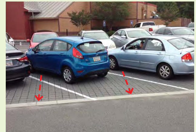
▲ This parking lot features pervious pavement within the parking stalls, however the parking stalls are graded so the pervious pavement only manages rainfall and no run-on from impervious areas.
