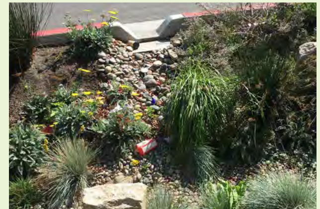
▲ Gravel or cobbles should be used in areas that may erode due to higher volumes or velocities of runoff.
