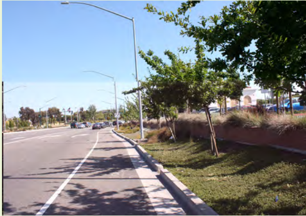
▲ The landscape area behind the curb has been designed as a gentle swale to capture, infiltrate low flows, and direct runoff off the street.
