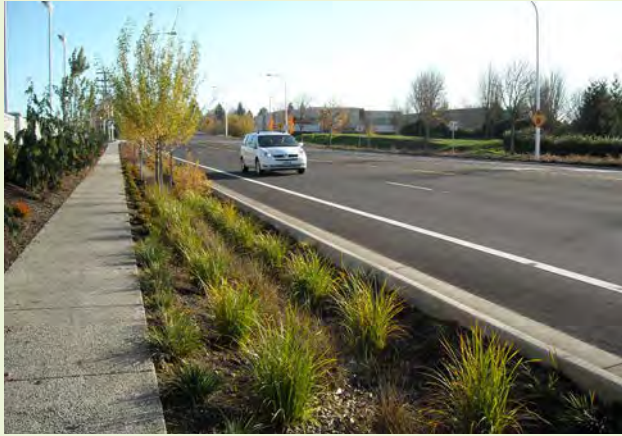
▲ This vegetated swale contextually fits well along this low-density residential arterial street and also features a pervious concrete sidewalk and new street trees.
