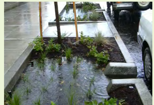
▲ Green infrastructure measures aid in collecting and filtering out pollutants before the stormwater enters the storm drain system or natural water bodies.
