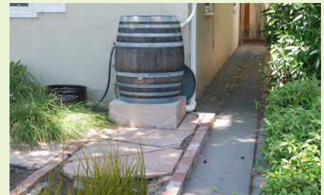
▲ This oak rain barrel at a residential property captures rainfall. Any overflow is directed to a stormwater planter.
