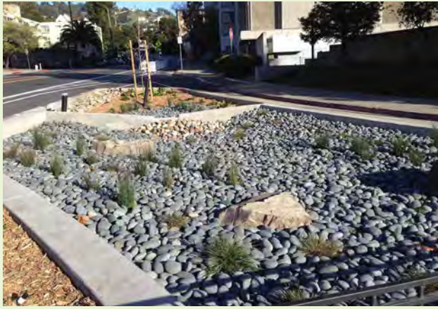
▲ Check dam slows runoff in sloped street conditions. This rain garden is also used to separate vehicle and bicycle facilities.
