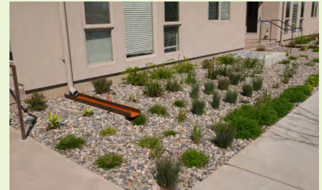
▲ This very shallow landscape strip has a large footprint to accept building rooftop runoff. Only 1 to 2 inches of runoff is retained in this facility.
