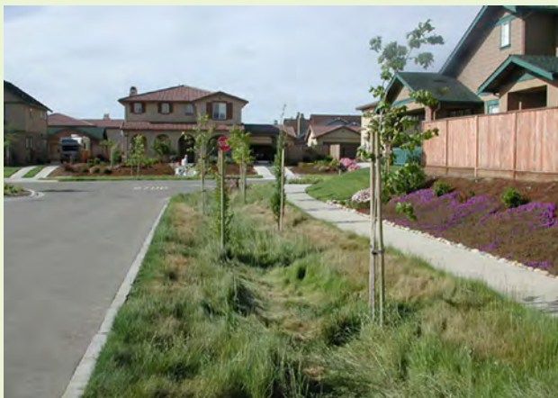
▲ Native grasses and oaks are used along a curbless street and in a vegetated swale to mimic a natural landscape.
