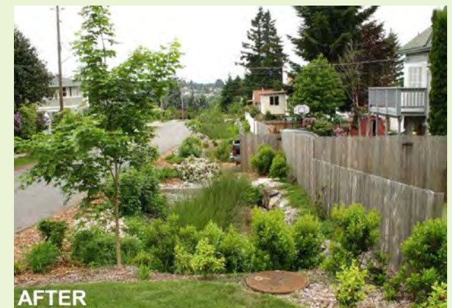
▲ AFTER: A curbless rain garden was installed to manage stormwater runoff from the road and beautify the roadway.
