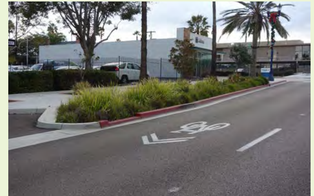
▲ Stormwater curb extensions are used at corners next to diagonal back-in street parking in this complete and green street retrofit project.
