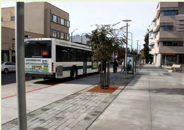
▲ Stormwater curb extensions can aid in traffic calming by visually narrowing the street and slowing vehicle traffic, while also allowing stormwater runoff to infiltrate into pervious pavement and tree well filters.
