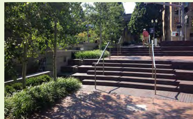
▲ A narrow stormwater planter is strategically cut into a staircase without impacting pedestrian flow.
