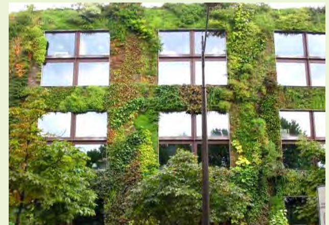
▲ Green infrastructure along building façades work to capture runoff on site, stabilize the internal temperature of the building, and reduce the heat island effect.
