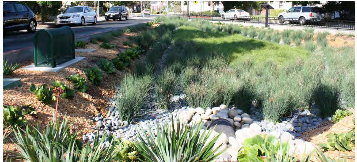
▲ This rain garden was a retrofit project specifically to implement green infrastructure, but it also helps enhance the community's character and calm traffic by installing vegetation where excess asphalt used to be.
