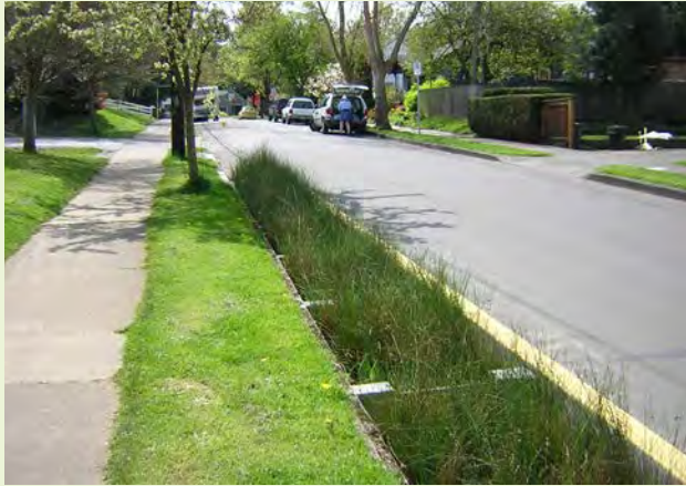
▲ Green gutter with weirs retrofitted into a residential street.
