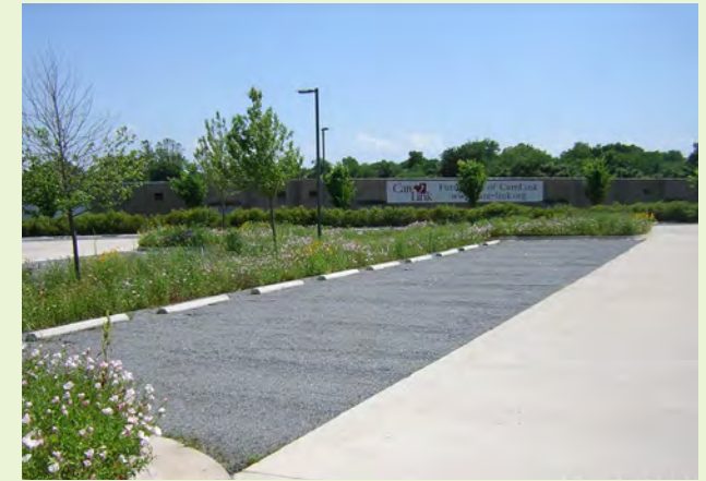
▲ A parking lot utilizing reinforced gravel paving within the parking lot stall area. This parking lot also has a vegetated swale to accept any potential overflow from the reinforced gravel area.
