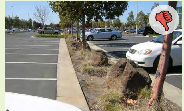
▲ Failed pedestrian circulation within a parking lot. Due to poor design, people have trampled this stormwater planter to the point where the landscape cannot grow.
