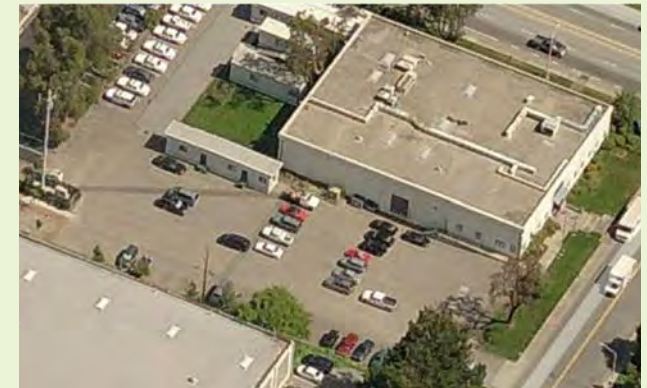
▲ The Brisbane City Hall site prior to retrofitting with a new parking lot and building landscape space was very inefficient in its layout.
