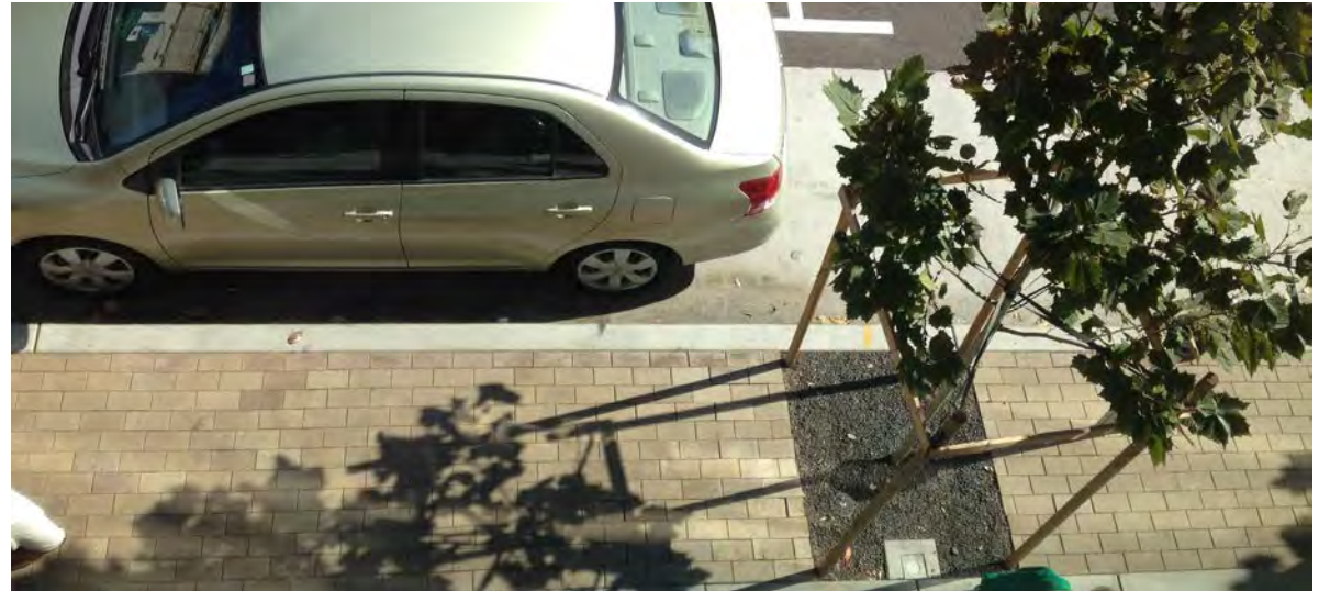
▲ Stormwater trees can be linked together with pervious pavement, modular suspended pavement, and other techniques to expand runoff storage capacity.
