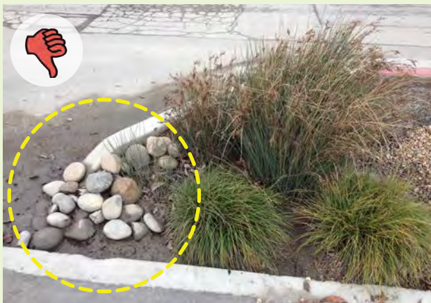
▲ River rock used to minimize erosion creates pockets of sediment accumulation that is difficult to remove.
