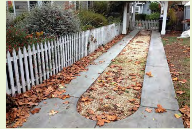
▲ EXAMPLE: A partial concrete/reinforced gravel driveway in a low-density residential setting.
