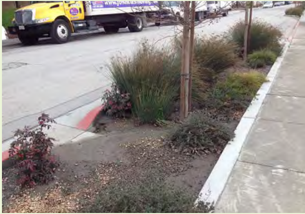
▲ Street sediment takes over this landscape on a regular basis without adequate prevention and maintenance.
