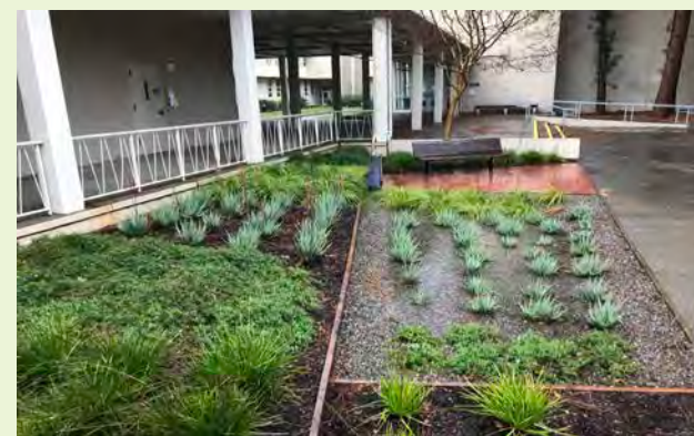
▲ This rain garden project that captures roof runoff at the UC Davis campus was built for under $3,500 and minimized the use of expensive materials.
