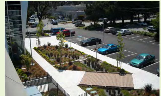
▲ After the retrofit, the Brisbane City Hall replaces under-utilized asphalt with a new rain garden without losing any parking spaces.
