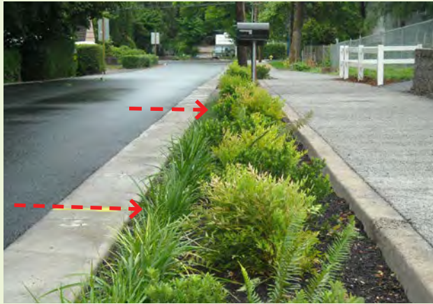
▲ This flush condition allows stormwater runoff to enter, evenly distributed, within a rural street green gutter system.
