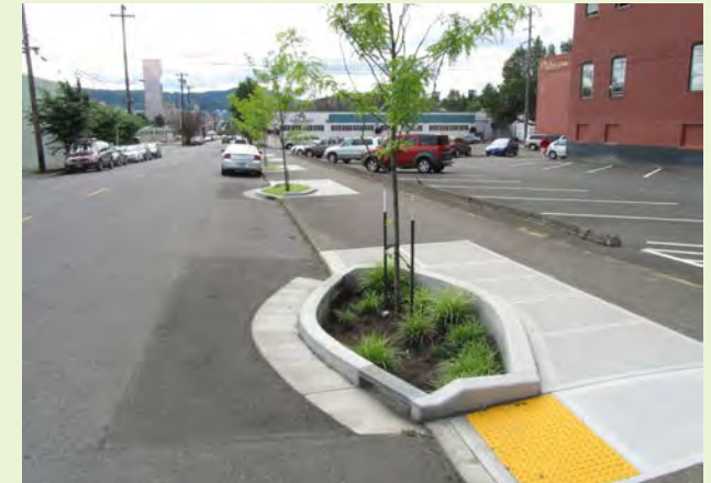
▲ Organic shaped tree well filters adjacent to accessible ramp completed as part of a retrofit project.
