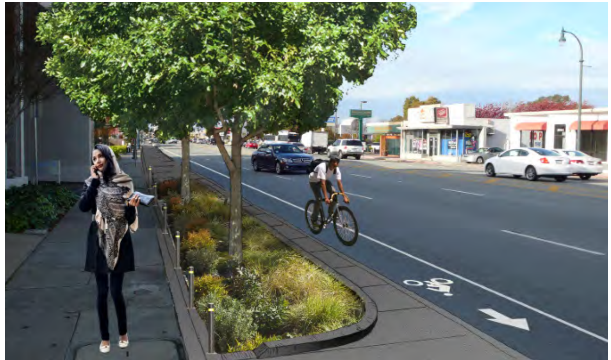
▲ RETROFIT OPPORTUNITY: The same street retrofitted with a stormwater curb extension in the parking zone. In this example a low-profile railing has also been added to the streetscape to keep people from entering the planter.
