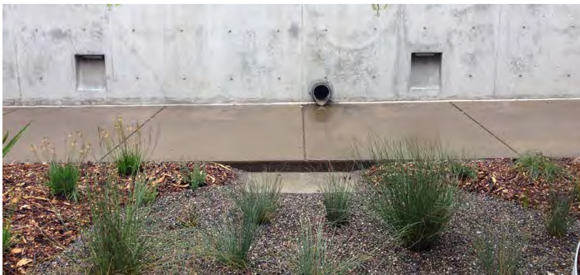
▲ This rain garden was strategically placed to capture the roof runoff from an existing roof downspout already integrated into the wall of the building.
