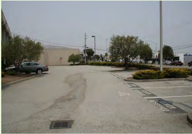
▲ EXISTING: A typical parking lot in San Mateo County that directs stormwater runoff inward towards an area drain.
