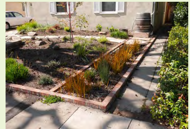
▲ EXAMPLE: An example residential stormwater planter that captures roof runoff first into a rain barrel and an excess runoff is directed to a stormwater planter.
