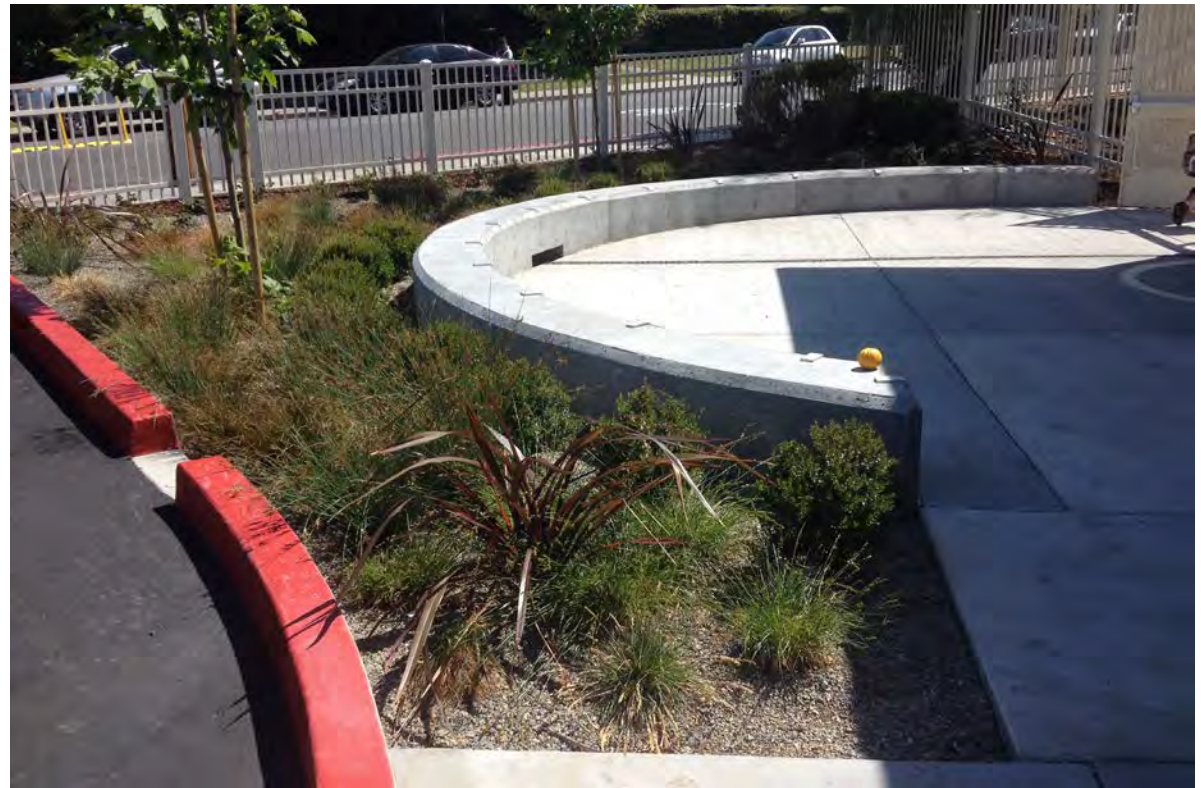
▲ A rain garden capturing surface and roof runoff at Laurel Elementary in San Mateo County is integrated into a student drop off zone.
