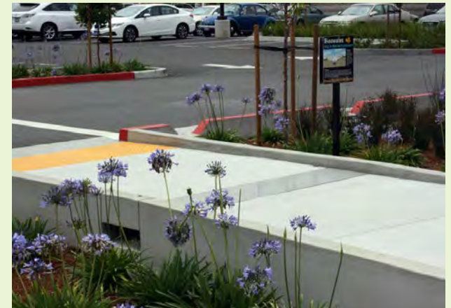
▲ Bridging structures allow for direct pedestrian access across linear green infrastructure measures.
