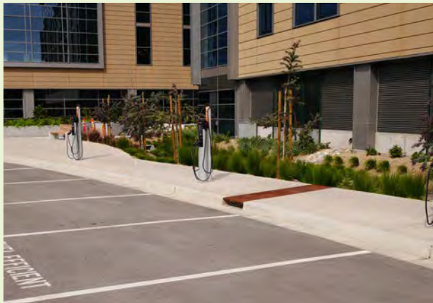
▲ This site development installed a rain garden to manage both building and parking lot runoff.
