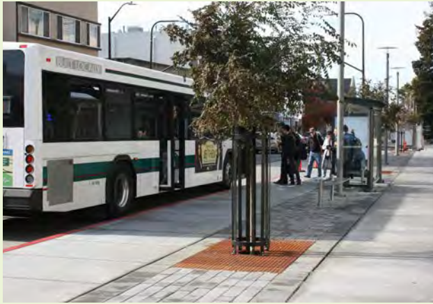
▲ Tree well filters are linked with pervious pavement and tree trench along with modular suspended pavement support cells to accommodate and treat runoff.
