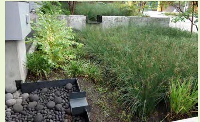
▲ Overflow systems can be staggered and combined between green infrastructure components. As one area overflows, it can spill into an adjacent treatment measure, and ultimately into an adequately sized overflow structure or outlet.
