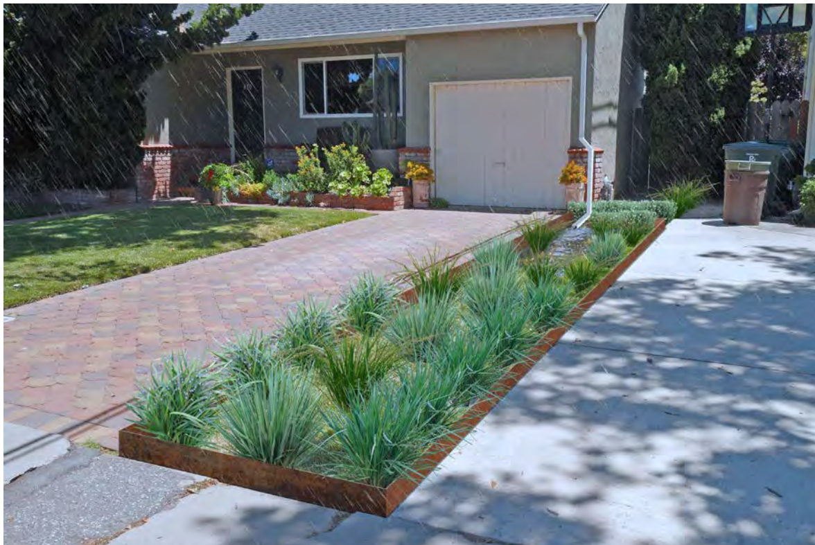
▲ RETROFIT OPPORTUNITY: The same residential landscape that converts a grass areas into a stormwater planter with drought-tolerant landscaping.
