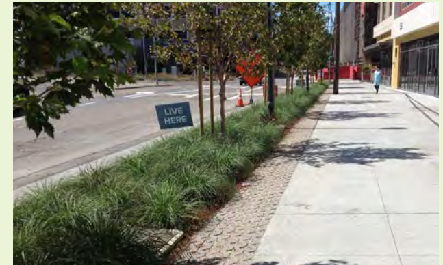
▲ This new streetscape planting features trees in addition to a strip of pervious pavement that allows for greater root volume.
