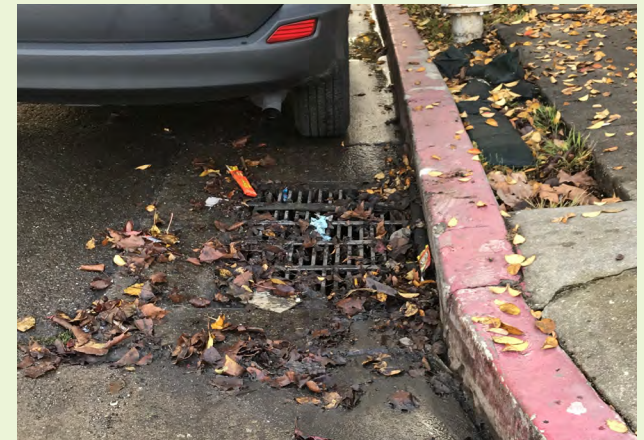
▲ Sediment, trash, and oils regularly collect in the street and flow into storm drain systems or water bodies.
