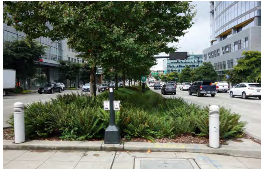
▲ Stormwater planters can effectively be located in street medians.
