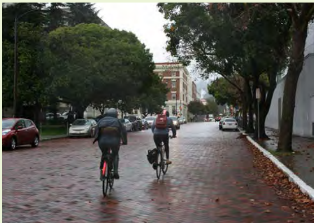
▲ This road is made of permeable pavers that can be easily biked on.
