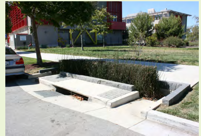
▲ Certain street projects, such as this new street, are required to meet C.3 provisions of the MRP.
