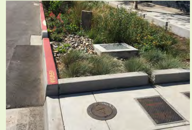
▲ Utilities located next to this green infrastructure facility are located outside the primary pedestrian crossing location. Designers should consider replacing utility covers and boxes in poor condition when designing retrofit projects.
