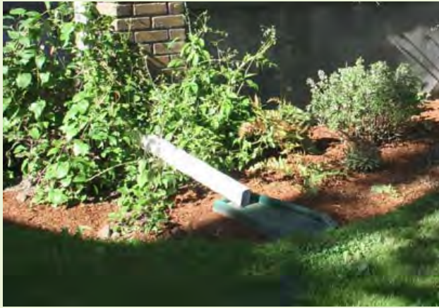
▲ A simple residential downspout disconnection directs roof runoff into a front yard.
