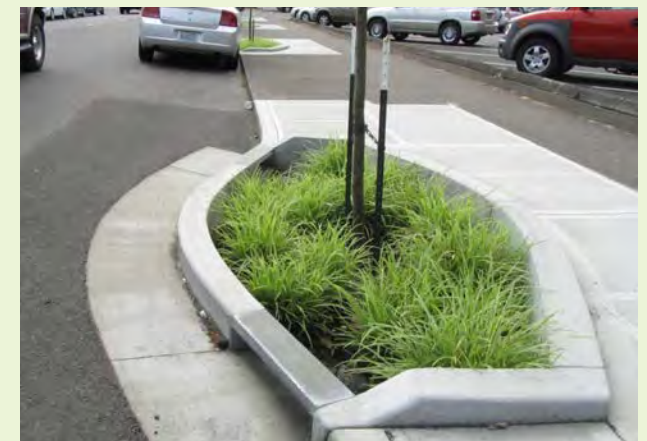
▲ Inlet/outlet is integrated into the curved curb.
