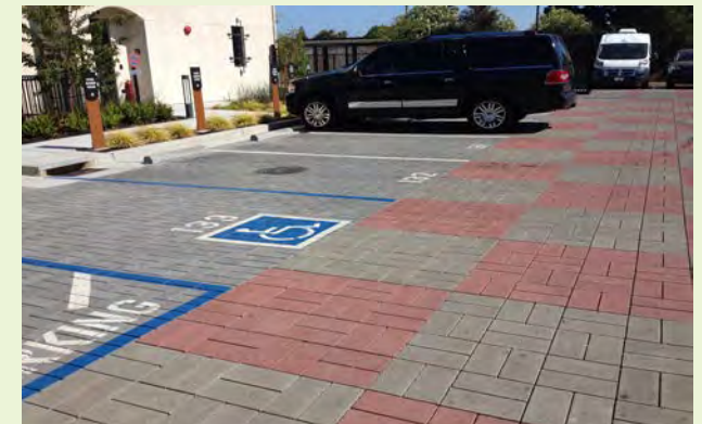
▲ A new development along El Camino Real in San Mateo County features permeable pavers throughout the parking lot.
