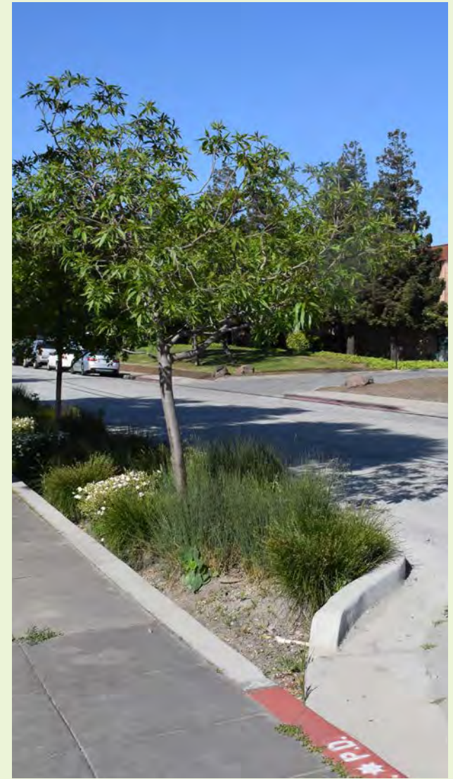
▲ Curb extensions with gaps allows stormwater runoff to enter the treatment measure.
