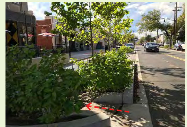
▲ This curb cut with side wings retains the side slope soil grade within a street stormwater curb extension project.
