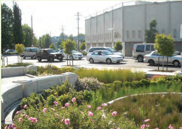
▲ Retaining walls double as weirs to expand the capacity of the stormwater facility and to retain and slow the runoff.
