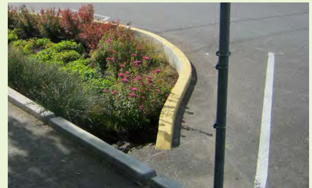
▲ The striping of this parking lot next to a stormwater planter allows for a 3-foot egress zone between the parking stall stripe and the landscape area. This protects both people and the landscape.
