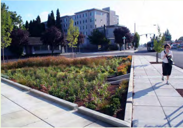
▲ A perimeter concrete curb was installed around this urban rain garden to help protect both pedestrians and the stormwater facility.
