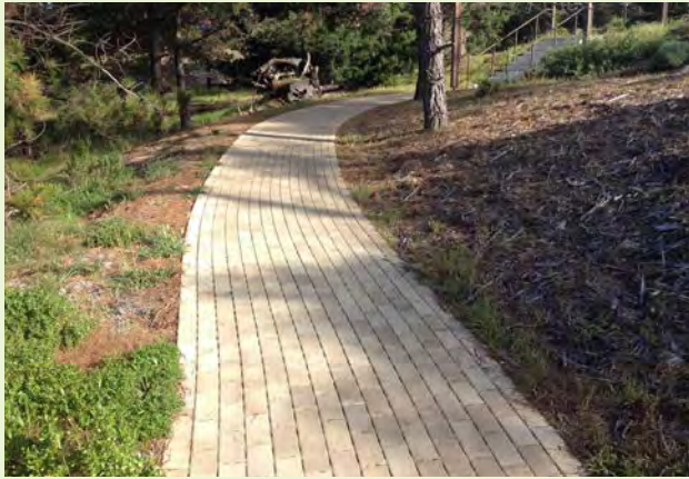
▲ Permeable pavers can accommodate meandering walkways and slopes to meet ADA compliance.
