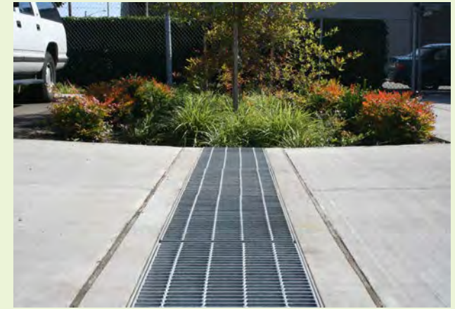
▲ This trench drain example connects two stormwater facilities within an industrial parking lot site.
