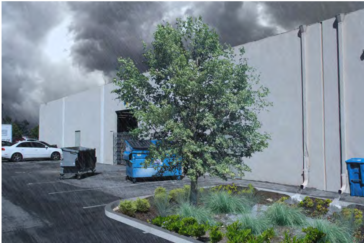
▲ RETROFIT OPPORTUNITY: The same industrial building site redirects a series of downspouts into a new stormwater planter. These stormwater planters can help add much-needed trees into industrial building sites.
