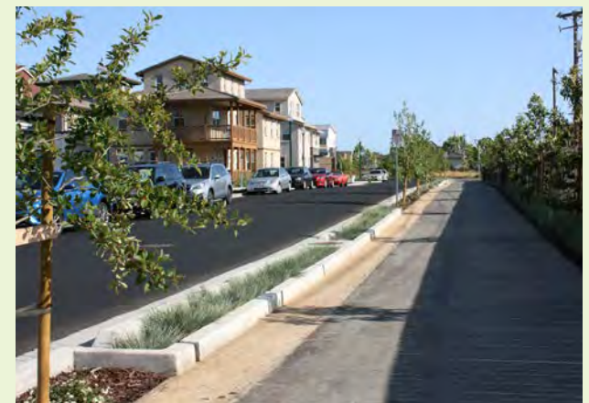
▲ Green gutter with notched curb edging collects and treats runoff from multi-use trail and street.
