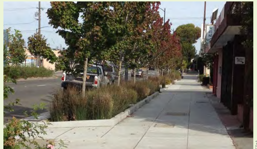
▲ Stormwater planters along this major arterial pick up runoff from the street through trench drains and curb cuts along the sidewalk.
