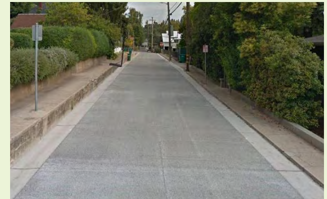
▲ This pervious concrete sidewalk is being retrofitted along El Camino Real in South San Francisco.
