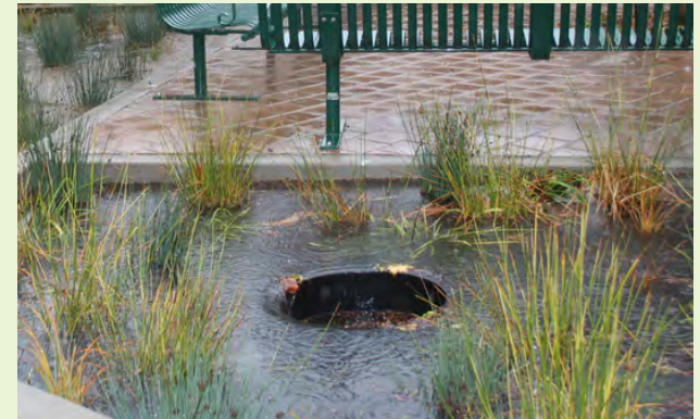
▲ This HDPE weir surrounds an inlet that is flush with the soil grade. The weir dictates the water level.
