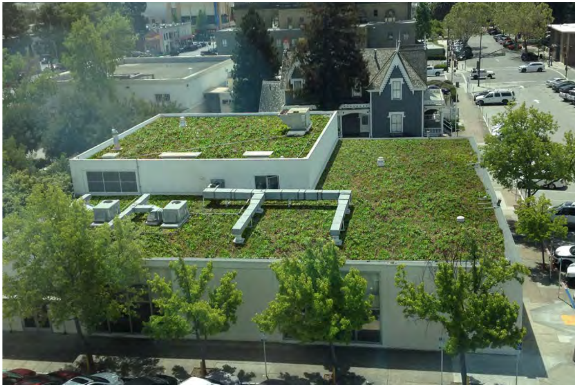
▲ RETROFIT OPPORTUNITY: The same commercial/office building rooftop with a light-weight extensive green roof application.
