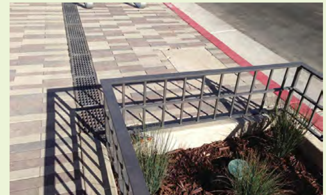
▲ Where there is significant drop in vertical grade, stormwater planters can use raised edges and/or perimeter low railings to allow pedestrians to detect the drop in grade.
