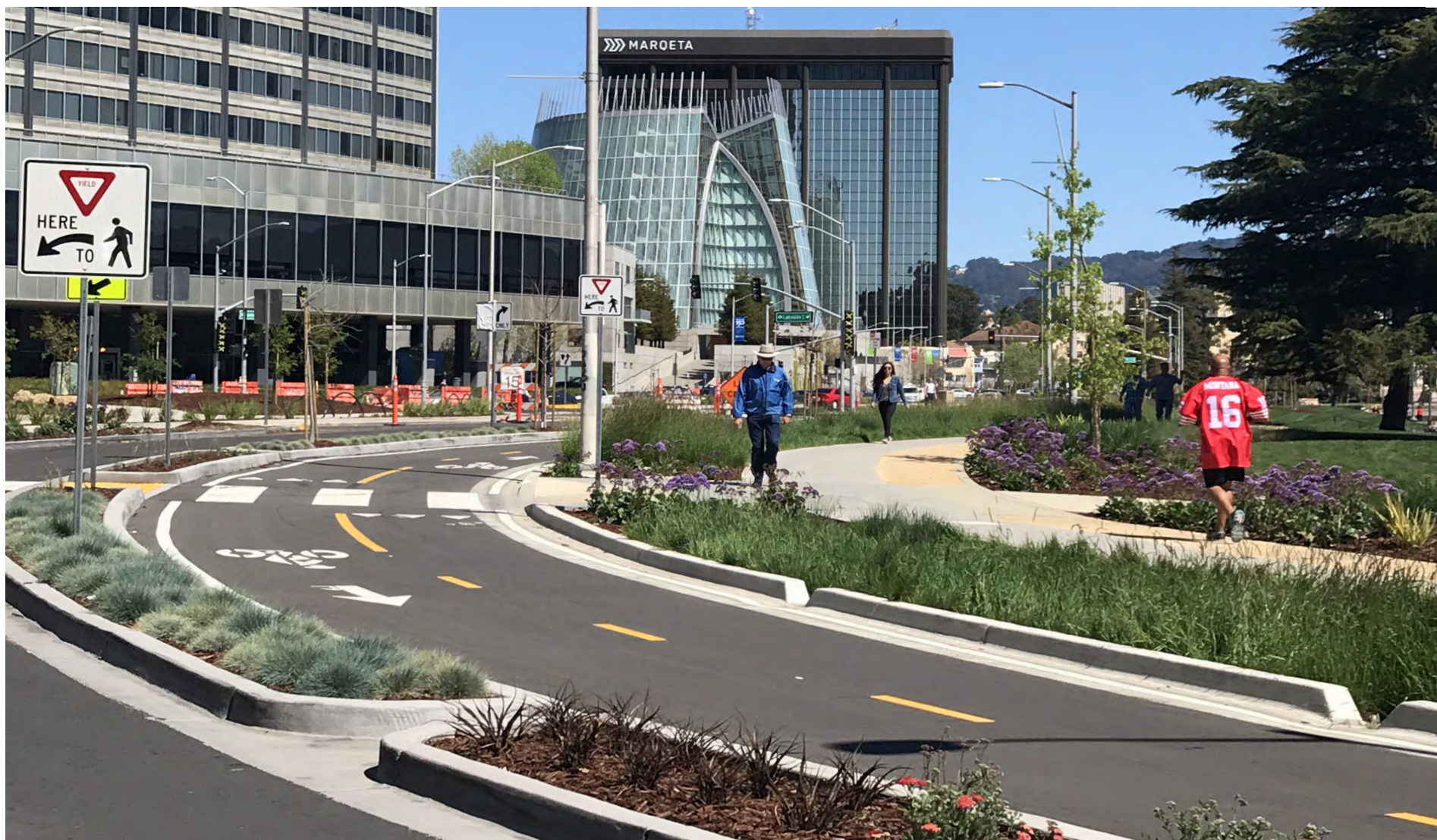
▲ A sustainable street retrofit in Oakland that integrates stormwater planters with improved pedestrian and bicycle (cycle track) facilities. Two-way vehicle traffic is located to (and off) the photograph to the left. Stormwater runoff flows from vehicle lanes through notches in a landscape buffer across the cycle track and into the stormwater planters on the opposite side of the street.
