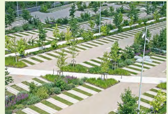
▲ This large parking lot distributes the stormwater landscape evenly throughout the parking lot.
