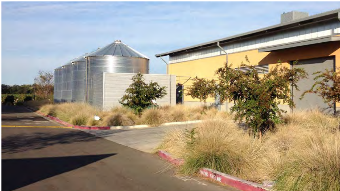
▲ A series of large cisterns stores water at the University of California, Davis.
