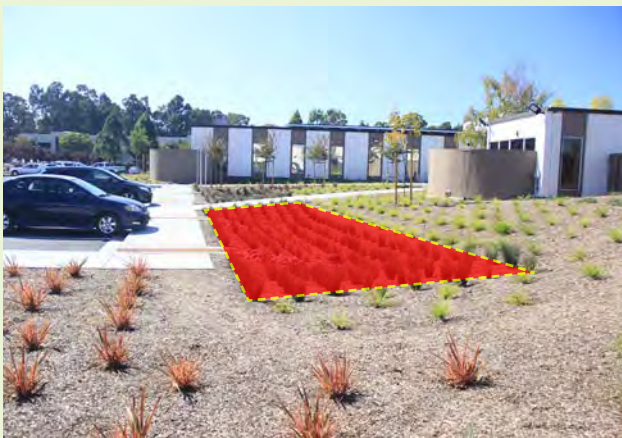
▲ Same project site, same issue of wasted landscape space that could be utilized for additional stormwater management. Only the red shaded portion is graded to accept runoff.
