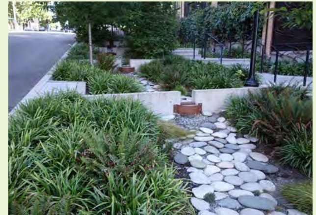
▲ The redevelopment of the adjacent multi-family project provided an opportunity for this green infrastructure measure to treat runoff from both public and private areas.
