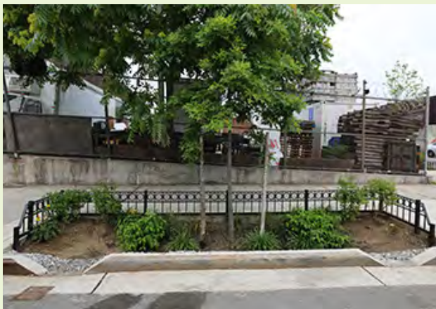
▲ This stormwater tree has two inlet/outlets which allows excess runoff to flow out of the planter and down the gutter to drop into an inlet.
