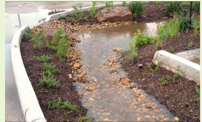
▲ Smaller rock at the flow line of a vegetated swale reduces to potential of erosion.
