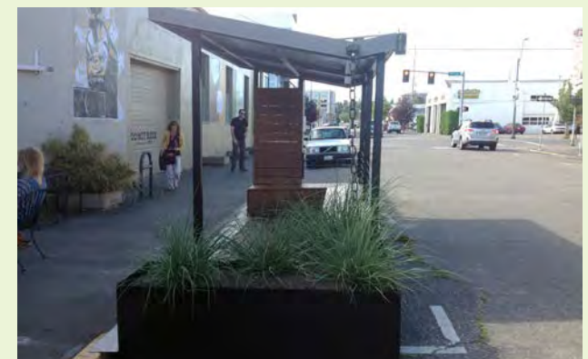
▲ A downtown temporary parklet's roof captures runoff directs it to a raised planter.
