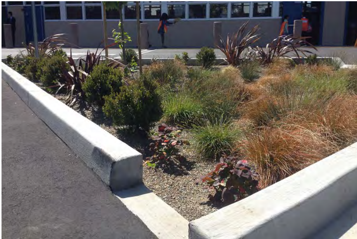
▲ Also at Laurel Elementary, a triangular parking lot rain garden island captures roof and surface runoff. Any overflow from this rain garden is re-captured within perimeter stormwater planters.
