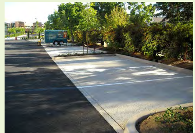
▲ EXAMPLE: This new parking lot utilizes pervious concrete within the parking lot's parking stalls.
