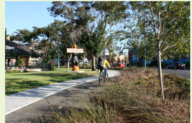
▲ EXAMPLE: Raised two-way cycle track and adjacent sidewalk separated from street by landscaping and stormwater attenuation.
