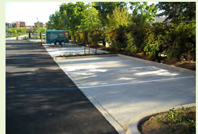
▲ Pervious concrete allows for stormwater management and its light color helps reflect heat rather than absorb it.
