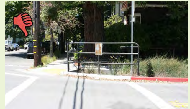
▲ Do not terminate crosswalks into green infrastructure facilities. This vertical walled stormwater planter was retrofitted to add a guardrail to keep people from entering the facility from the crosswalk.
