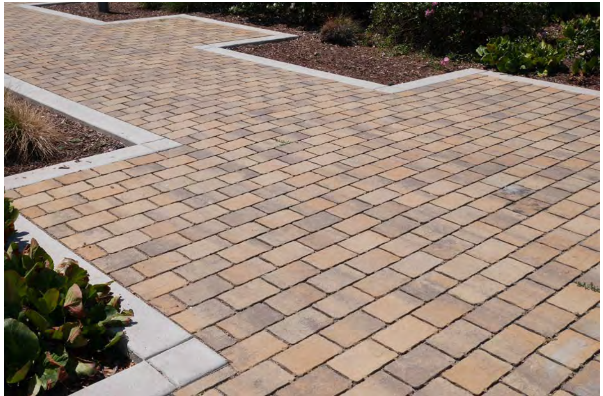
▲ EXAMPLE: This high-density residential apartment complex uses pervious pavers throughout all of its walkways. This paving material choice also provides some visual appeal over standard concrete.
