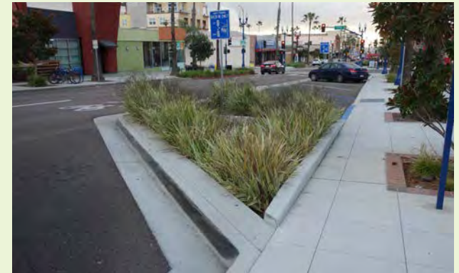
▲ Plants should be selected and placed to not impair the visibility of pedestrians and cyclists to drivers while still providing an attractive appearance to the community.
