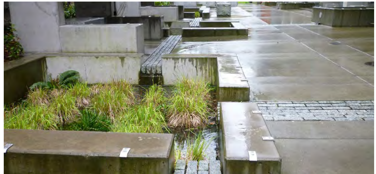
▲ This plaza space in Portland, Oregon directs roof runoff via a series of granite paver channels allowing water to flow through the joints of the pavers until it reaches the landscape.
