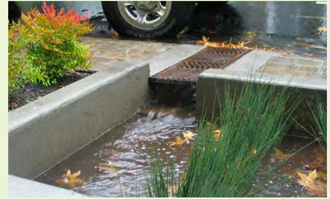
▲ A recessed concrete forebay at the end of a trench drain channel helps dissipate energy as water flows into the landscape.
