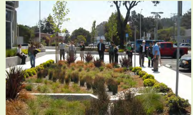
▲ This rectangular rain garden area receives runoff from both a parking lot and the building's rooftop.
