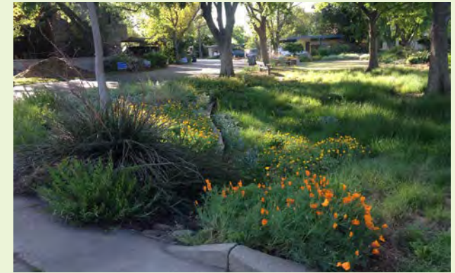
▲ A rain garden in Village Homes accepts street and site runoff.
