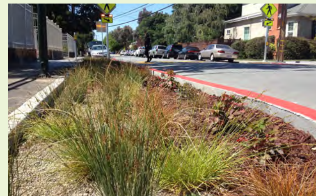
▲ This green street uses pea gravel mulch in the flow path of water and organic mulch on upland side slopes.
