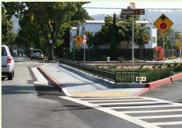
▲ An offset and angled intersection was retrofitted to include an extensive rain garden. Storm drain pipes from two streets outfall into the rain garden, which set the depth of the rain garden.
