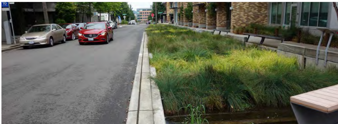
▲ Stormwater planter design, configuration, and location can vary depending upon the context and need for pedestrian circulation.
