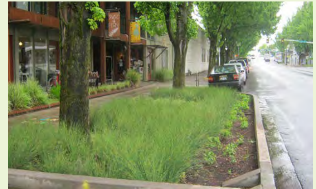
▲ This stormwater curb extension had enough horizontal space to gently transition in grade between the mature trees and the finish grade of the facility.
