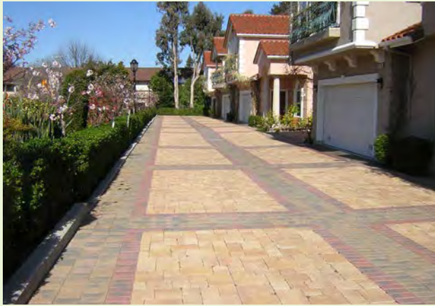
▲ EXAMPLE: Pervious pavers in a common shared driveway in San Mateo County.
