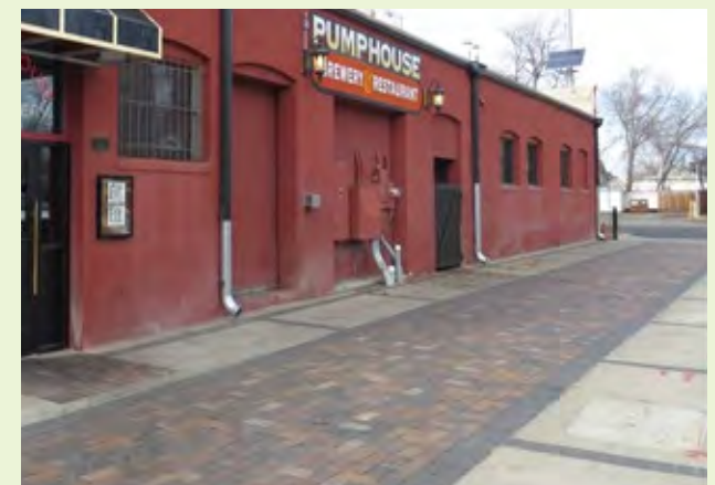
▲ EXAMPLE: Different types, colors, and textures of pervious pavements can add interest and aid in defining primary vehicle travel ways and other spaces such as primary pedestrian areas and loading.
