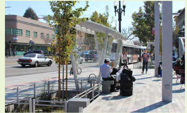
▲ Low fences and light bollard seats can be used to prevent people from entering green infrastructure facilities and to protect the function of the utility.
