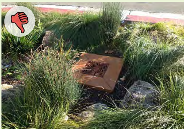
▲ Conversely, this stormwater curb extension has no check dams and is graded to retain little stormwater. As a result, most of the runoff simply enters the inlet without any ponding of water.
