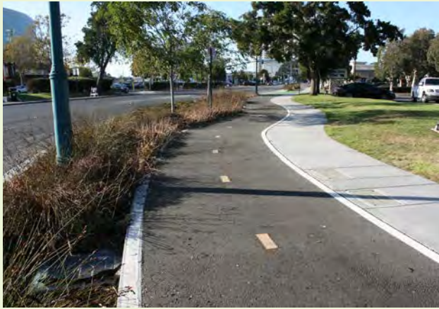
▲ A stormwater planter separates both bicycle and pedestrian circulation from vehicular traffic.
