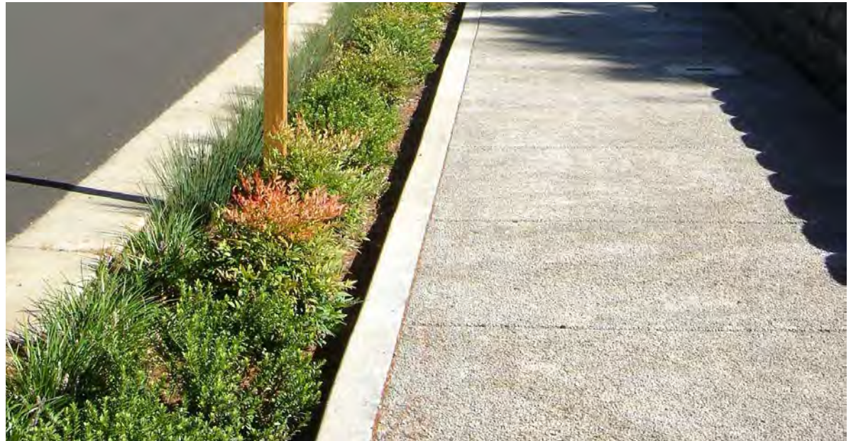
▲ This narrow green gutter on a rural residential street features a “curbless” condition allowing street runoff to sheet flow into the landscape.
