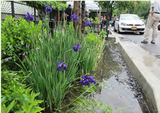
▲ Stormwater trees can have one or two inlets/outlets depending upon the amount of runoff to be captured and the grading and drainage design.
