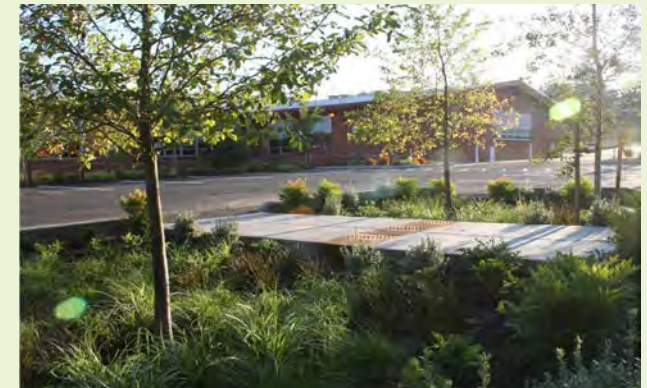
▲ This parking lot used to be completely paved. The new parking lot features a 2,000 square foot rain garden.
