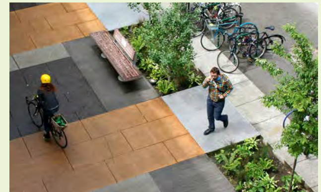
▲ A “curbless” green street features a drop in grade less than 4 inches and has multiple steel bridges that allow pedestrians to cross over the stormwater planter system.
