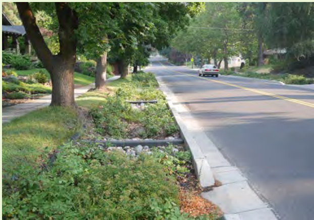
▲ This vegetated swale retrofit in Spokane, Washington preserves existing street trees and features check dams to slow water down as it moves through the landscape system.
