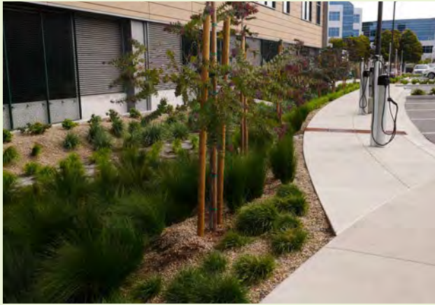
▲ This vegetated swale in San Mateo County captures both parking lot and building rooftop runoff.
