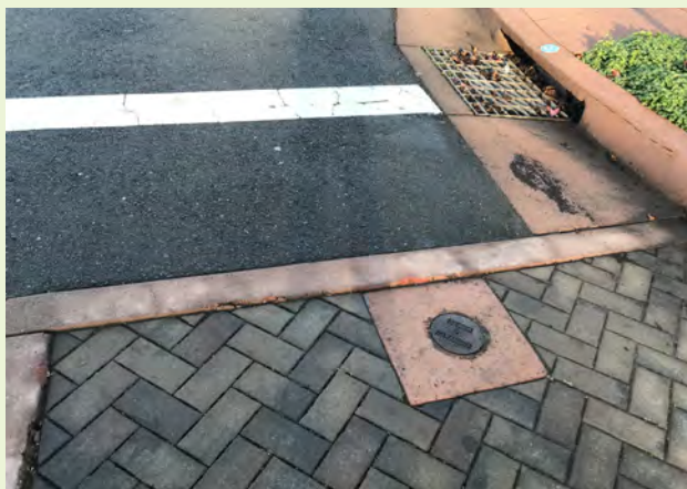
▲ This pervious paver parking lane contains a clean out and is located downstream of a stormwater facility and upstream of a drop inlet, which manages runoff that does not infiltrate into the paver system.
