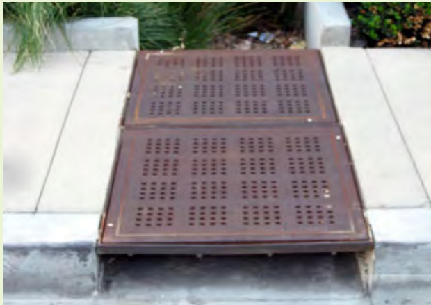
▲ Detail of trench drain directing runoff from the street to the stormwater planter set back from the on-street parking lane.
