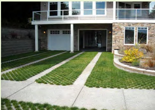
▲ Grass paving installed in a residential driveway.
