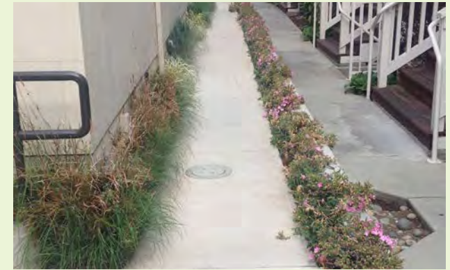
▲ A 12" wide green gutter accepts runoff from a building pathway.
