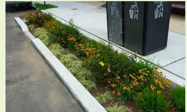
▲ A green gutter in Philadelphia accepts street runoff.
