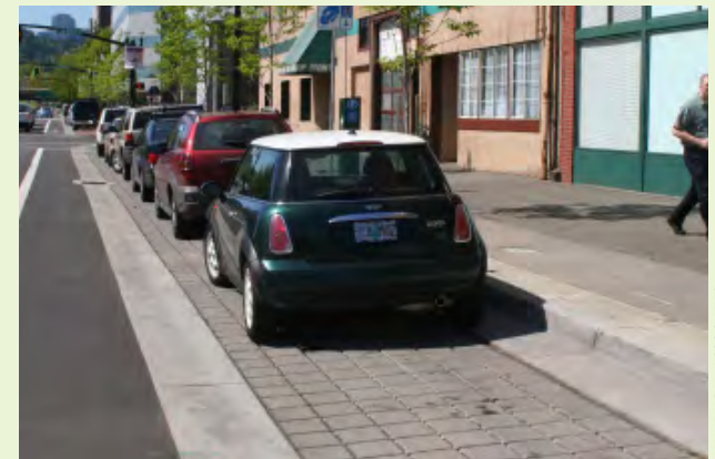
▲ EXAMPLE: This urban street uses pervious paving in its parking lane and could have been further refined with stormwater curb extensions.
