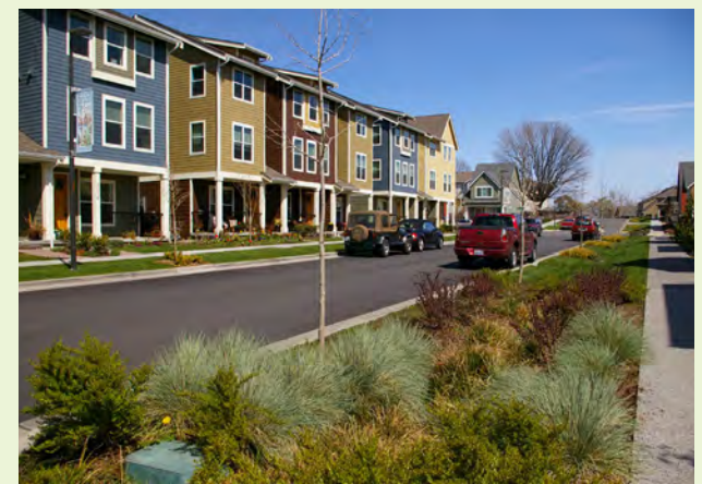
▲ Vegetated swale provides a buffer to pedestrians walking along the street from vehicle traffic. Periodic pedestrian bridge crossings could be provided to improve this design.
