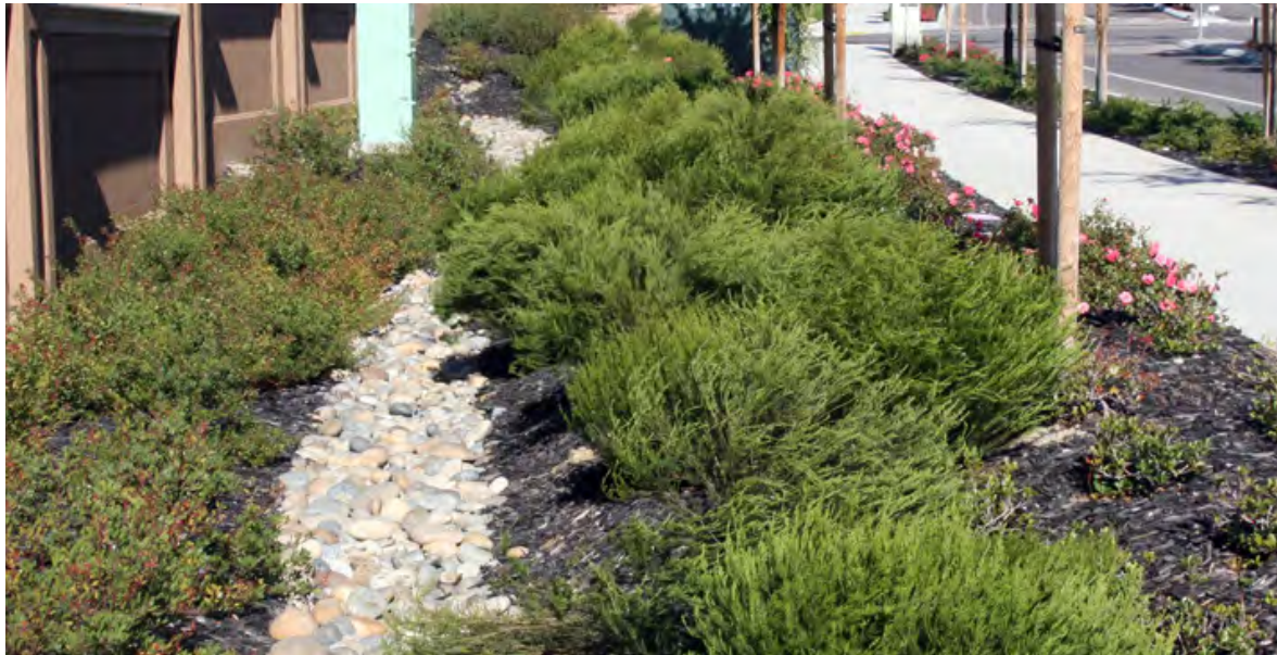
▲ Infiltration trench placed behind sidewalk within the right of way.
