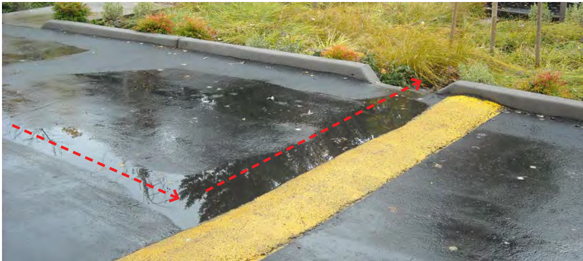
▲ This asphalt speed bump redirects stormwater into a rain garden curb cut during storm events. Without the speed bump in place, runoff would bypass the curb cut and create a missed opportunity for stormwater treatment.
