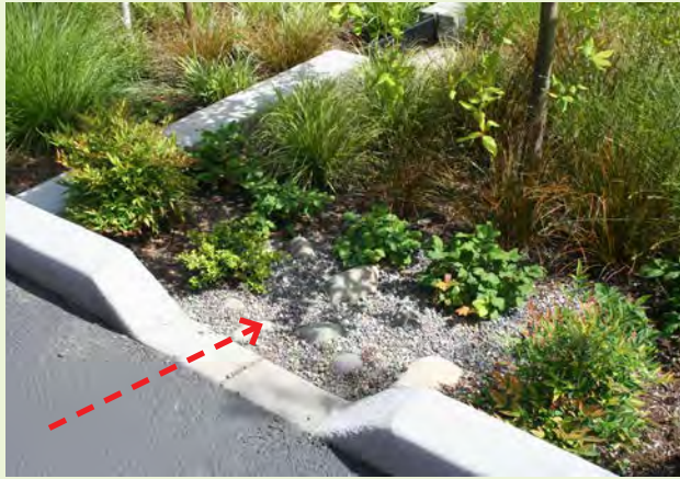
▲ A standard curb cut allows stormwater runoff to enter a parking lot rain garden. This curb cut has 45 degree chamfered sides.
