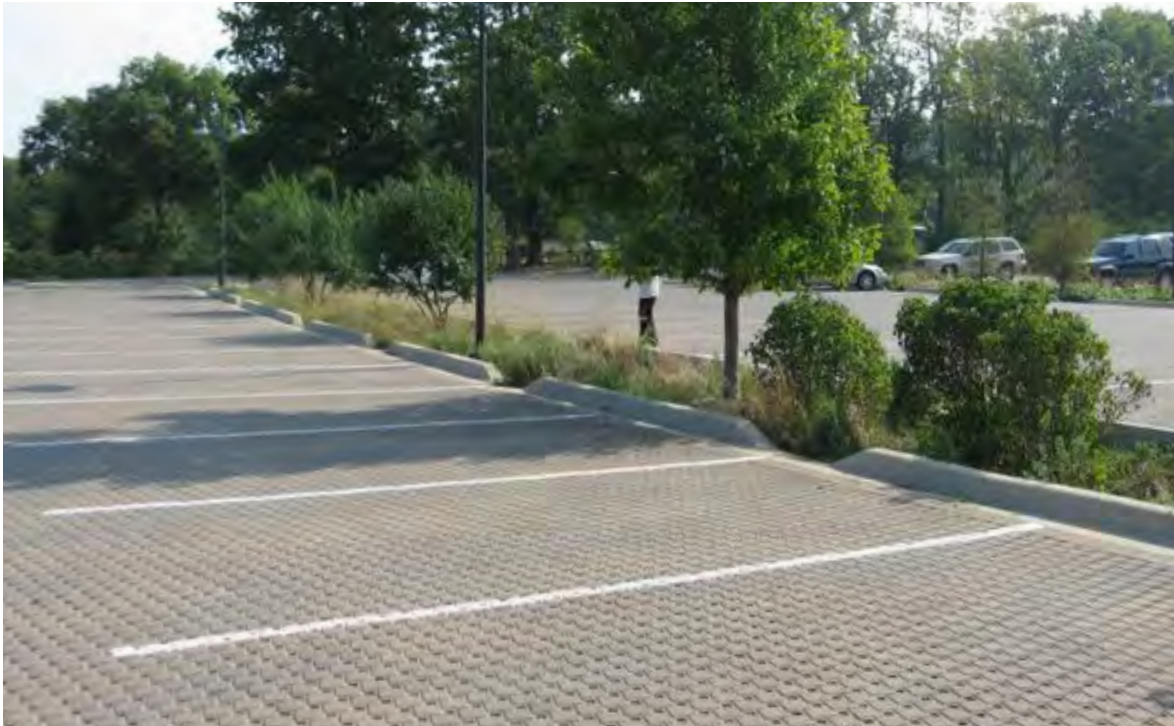
▲ Permeable pavers within a parking lot application. Any overflow from the pervious pavement system drains into a vegetated swale.
