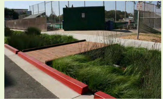
▲ Pedestrian bridges allow convenient crossing of recessed green infrastructure measures. This crossing is not ADA accessible at the street side.
