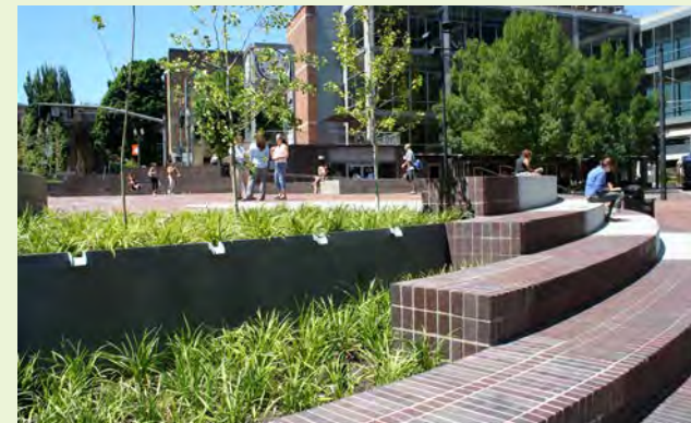
▲ A metal weir separates a drop in grade from one stormwater planter to the next. Scuppers along the weir allows for overflow to occur at controlled points.
