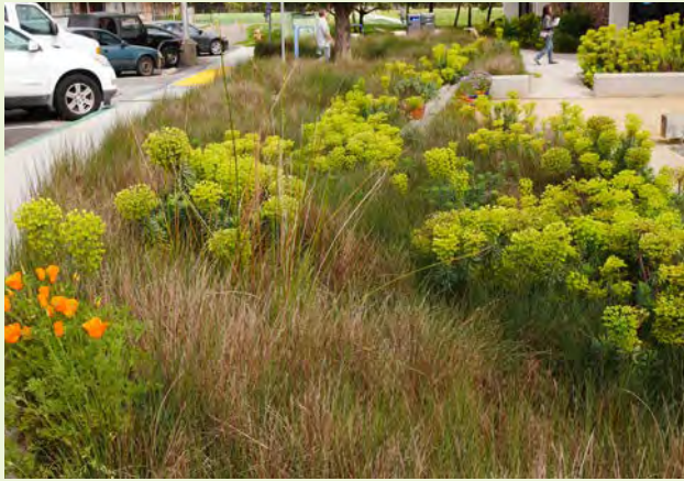
▲ This rain garden at the Serramonte Library front entrance accepts runoff from a large parking lot.
