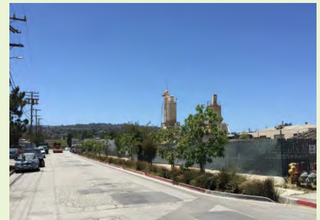
▲ EXAMPLE: This industrial street placed stormwater curb extensions in a parking lane to collect and treat runoff.
