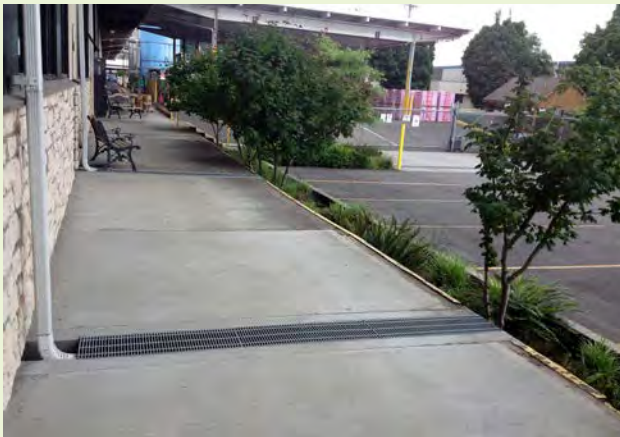
▲ EXAMPLE: An example industrial stormwater planter captures roof and sidewalk runoff via a trench drain.
