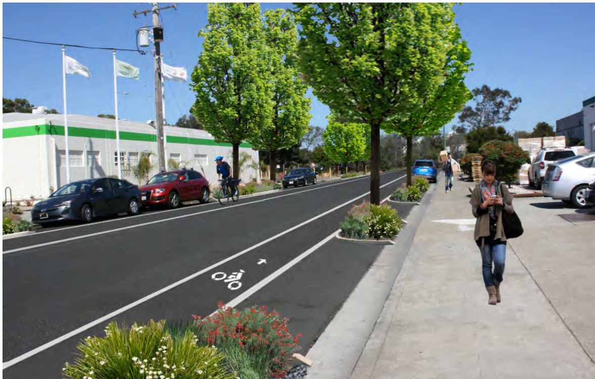
▲ RETROFIT OPPORTUNITY: The same industrial street retrofitted with stormwater planters in the parking lane of the street, as well bike lanes added.
