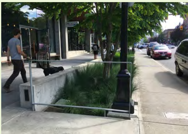
▲ Step out area between stormwater planters and parking allows for convenient entry for pedestrians into and out of vehicles. Intermittent walkways between the step out area and sidewalk allows convenient access to and access to destinations.
