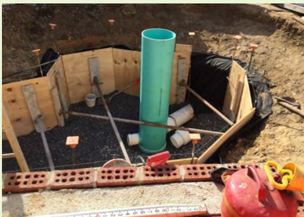
▲ The use of underdrains is important in places with poor infiltration and other conditions.
