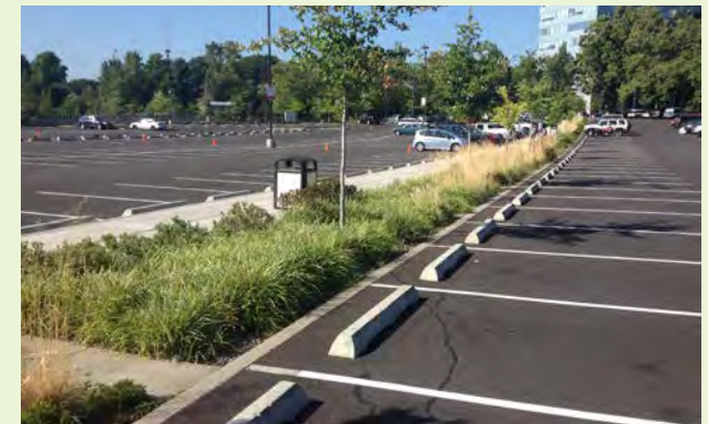
▲ A vegetated swale within a large parking lot. Notice that there is pedestrian pathway along on side of the vegetated swale to facilitate better site circulation.
