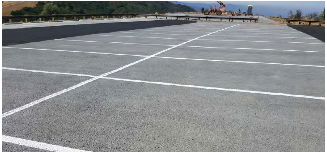
▲ Pervious pavements, such as the pervious concrete installed in this expansive parking lot, can be used to infiltrate stormwater, reduce runoff from the site, and improve water quality.
