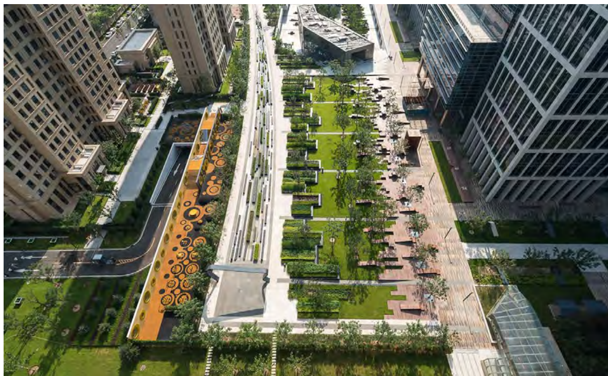
▲ This project in China shows the potential to green entire city blocks while still creating a beautiful balance between pedestrian space and landscape space. This project manages all of its stormwater runoff on site.
