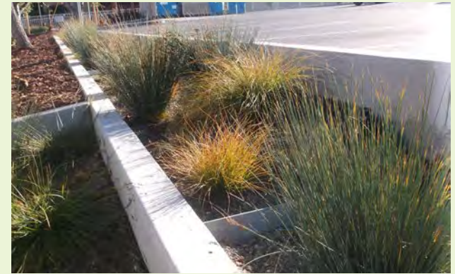
▲ This stormwater planter has several metal weirs placed along the flow path of water to encourage infiltration.
