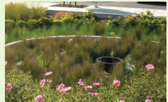
▲ A HDPE overflow weir surrounds a drain inlet that is flush with the soil surface. The weir dictates how much water is retained at any given time and can be replaced with a different height weir or removed completely.
