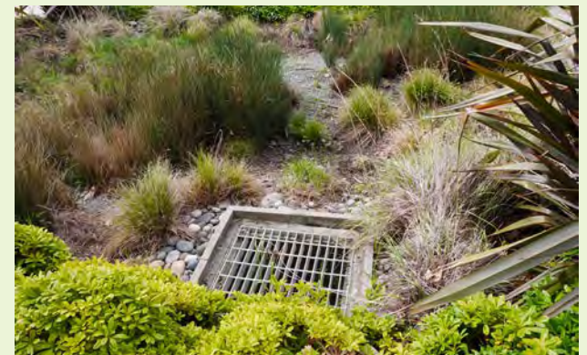
▲ Surrounding a flush inlet are raised bricks to create a simple raised weir effect and retains additional runoff.
