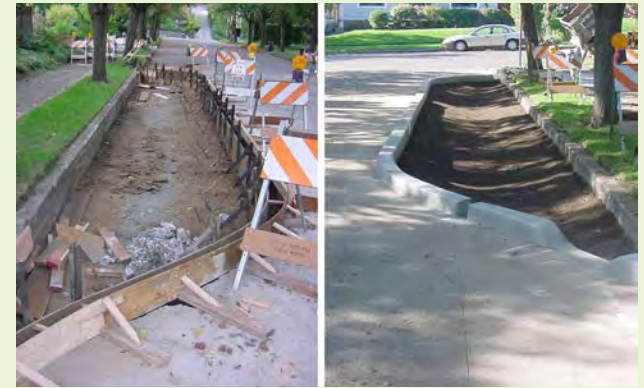
▲ Stormwater curb extensions constructed at the NE Siskiyou Green Street used the existing street curb to be the vertical transition in grade between mature trees and the finish grade of the facility.
