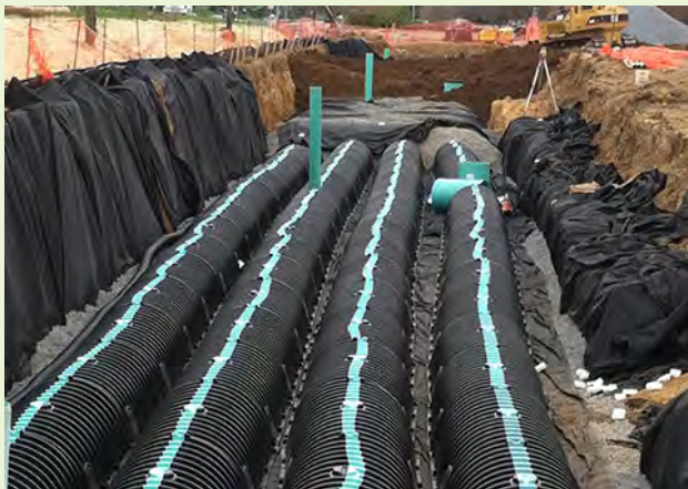
▲ Subsurface infiltration systems are useful in sites that are constrained for above ground green infrastructure measures.
