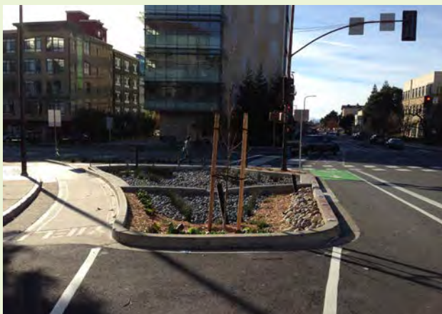
▲ This rain garden within a street separates a "free right" turn bike lane from through bike and vehicle lanes. The rain garden could have been extended toward the viewer to provide greater runoff treatment.
