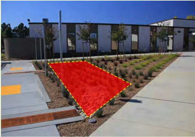
▲ This triangular space does not maximize the potential for stormwater management. Only the red shaded portion is graded to accept runoff.
