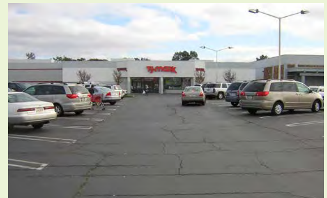
▲ A typical parking lot void of landscape space and completely impervious.
