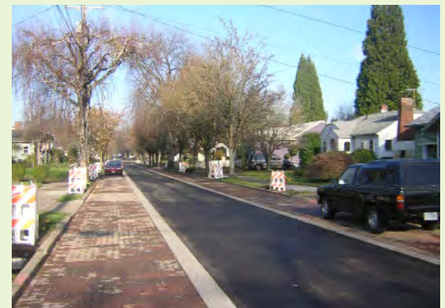
▲ EXAMPLE: A residential street is retrofitted with pervious paving.
