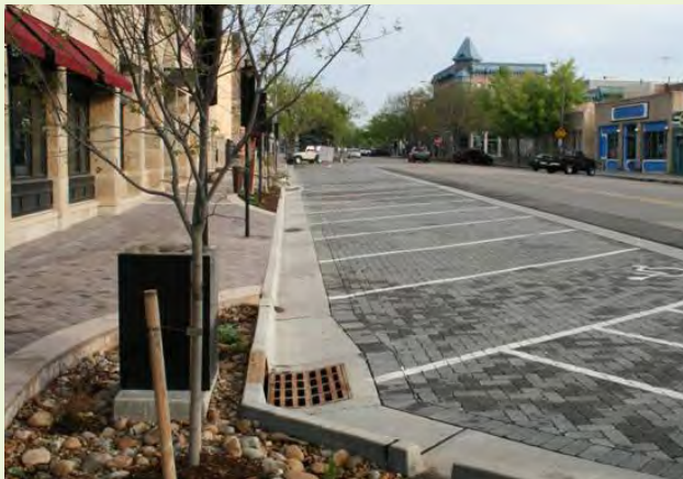
▲ Stakes and ties provide this newly planted tree with support while it acclimates to its new condition. An agreement between a developer and the city allowed multiple shared use green infrastructure measures to collect runoff from private and public areas.
