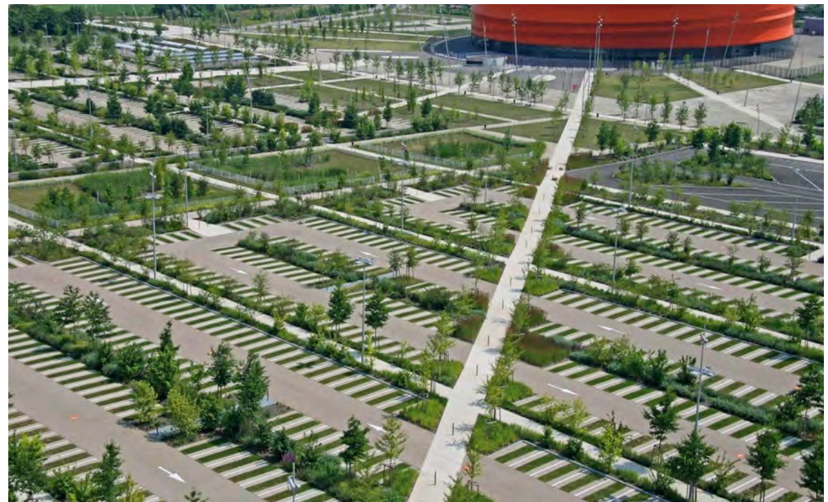
▲ This innovative parking lot example in Strasbourg, France boldly greens the parking lot with trees, pervious pavement, stormwater planters, and provides superb pedestrian circulation. This is an excellent example of balancing parking spaces with landscape and people space.
