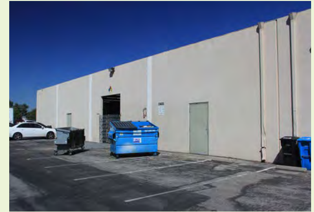
▲ EXISTING: A typical large-scale industrial building site in San Mateo County.
