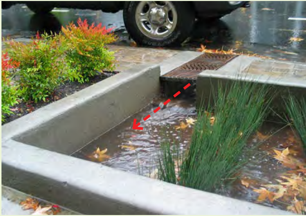
▲ A grated curb cut allows stormwater to pass under a pedestrian egress zone to the stormwater facility.
