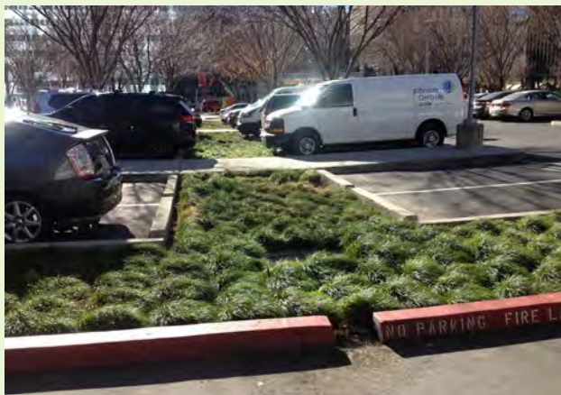
▲ A parking lot in Sacramento incorporates a vegetated swale and sites tree islands every two to three parking stalls to help shade asphalt surfaces.
