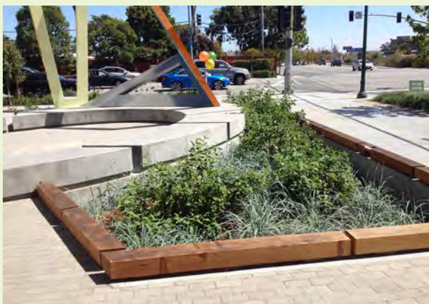
▲ EXAMPLE: An example plaza rain garden captures sidewalk runoff and features low-water plant communities.
