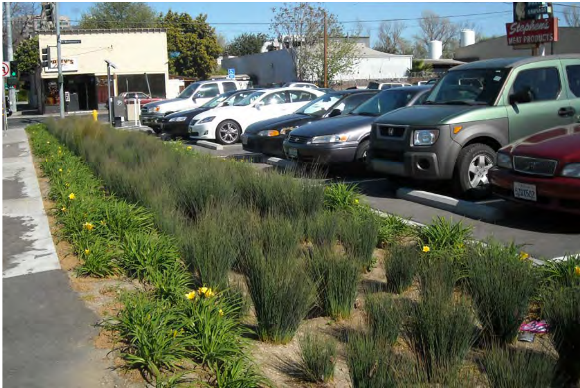
▲ This vegetated swale in Oakland, California was retrofitted within an existing parking lot.
