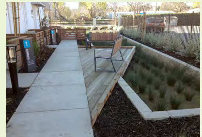
▲ EXAMPLE: An example high-density residential rain garden captures roof runoff and features a boardwalk overlook and seating area.
