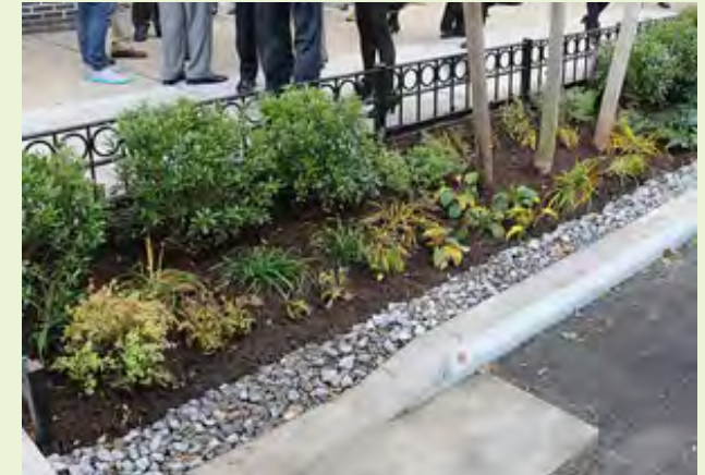
▲ The gravel band along the curb helps to dissipate stormwater runoff flows into the planter.
