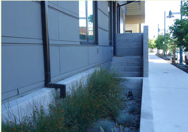
▲ Disconnected downspouts reduce runoff from entering the storm drain.
