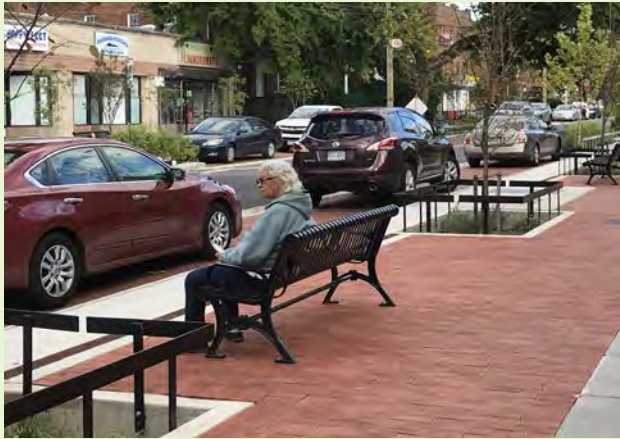
▲ Tree well filters linked by trench drain to can be edged with low curbs or railing and used with or without a tree grate.
