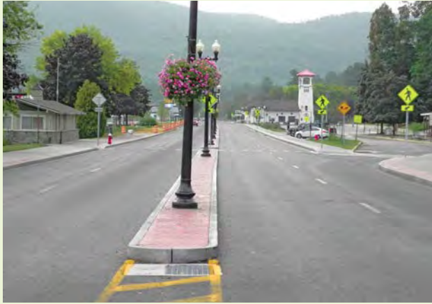
▲ Porous asphalt was used in this street's repaving.
