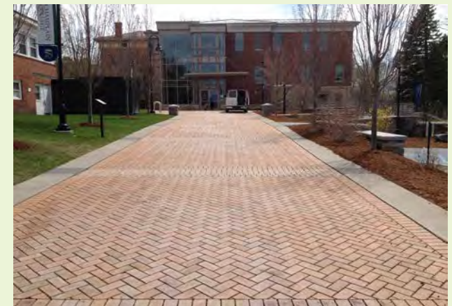
▲ EXAMPLE: An example of a school walkway using pervious pavers.
