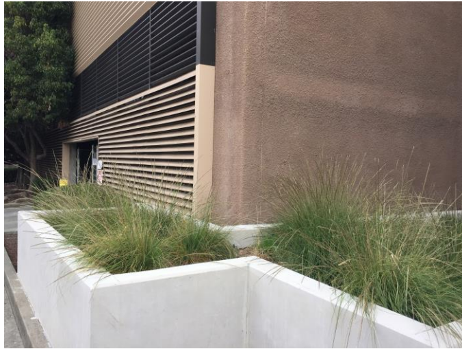
Figure 8-5: Flow through planter in Emeryville (Credit: EOA, Inc.)
