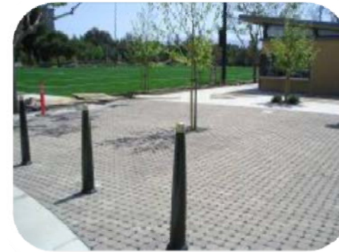
Permeable Interlocking Concrete Pavers
