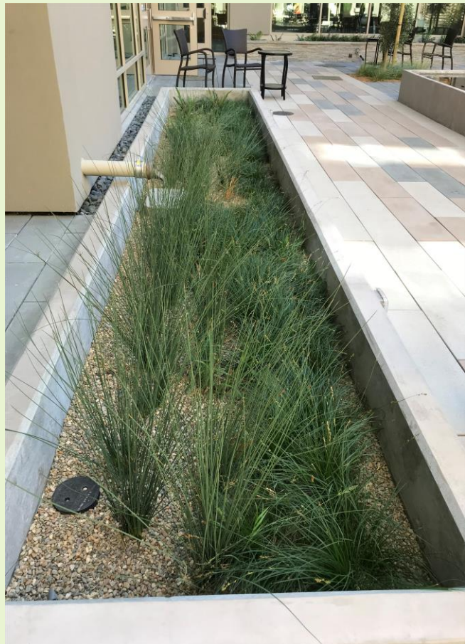
Figure 6-13: Flow-through planter with gravel rock mulch. (Credit: City of Burlingame)
