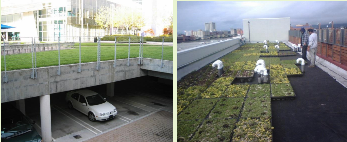
Figure 6-44: Parking Lot with Turf-Covered Intensive Green Roof, Google building, Mountain View; and Modular Extensive Green Roof installation, Emeryville. (Credit: EOA Inc.)
