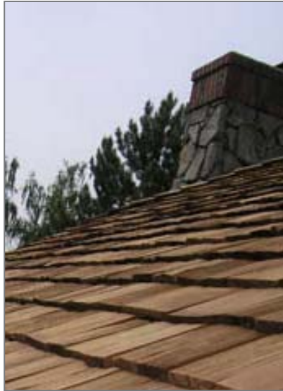
Wood shingle roof Courtesy of Gutter Glove
