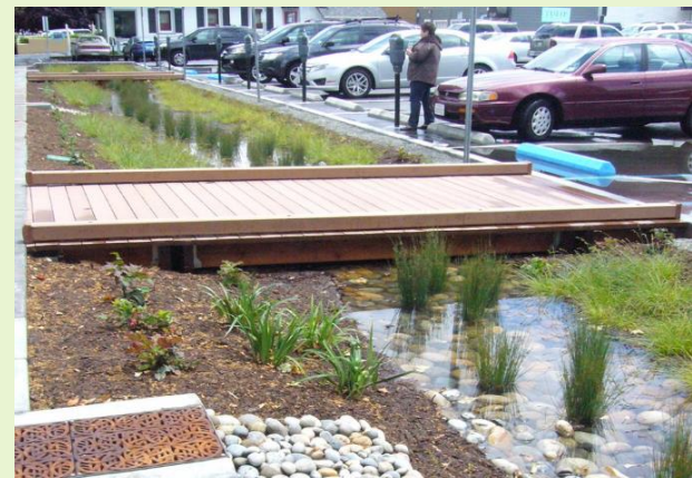
Figure 6-3: Bioretention area in a multi-family residential property in Redwood City (top; Credit: EOA, Inc.) and in a parking lot in Burlingame (bottom; Credit: SMCWPPP)
