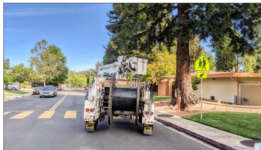
Red curb striping does not extend the full length of the intersection at Sharon Road and Eastridge Avenue. Drivers were observed stopping in the intersection and blocking the crosswalk.
