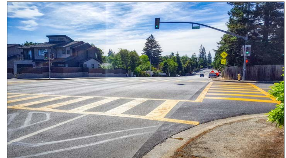
The crossings at Sharon Road and Alameda De Las Pulgas lack curb ramps. Pedestrian push buttons at Alameda / Sharon Road lack tactile directional indicators and are located on the same pole.
