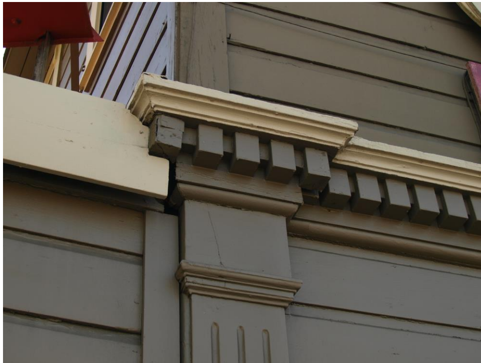
Detail of front façade, viewed facing west.
