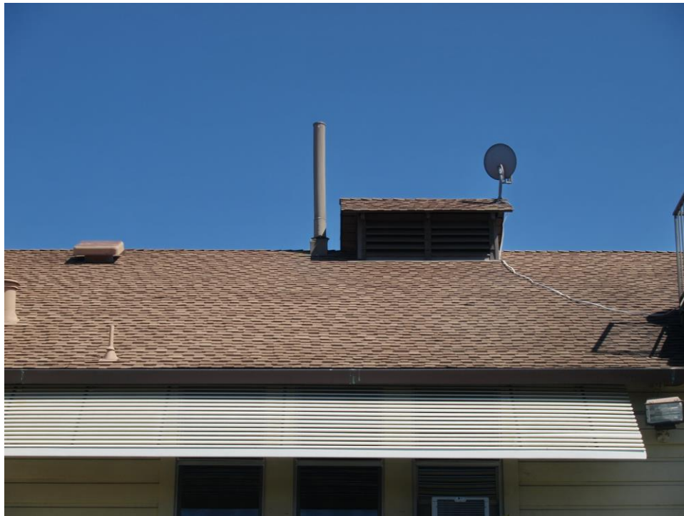
Roof detail with existing antenna, viewed facing southeast.
