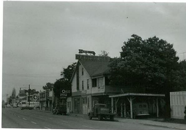
#2 Showing the Oasis building from the North
