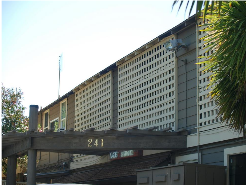
Detail view of lattice screen and entry trellis on side elevation, viewed facing west.
