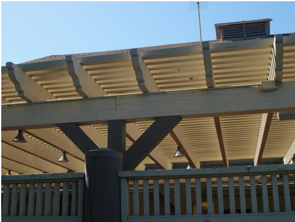
Detail of trellis, viewed facing northwest.
