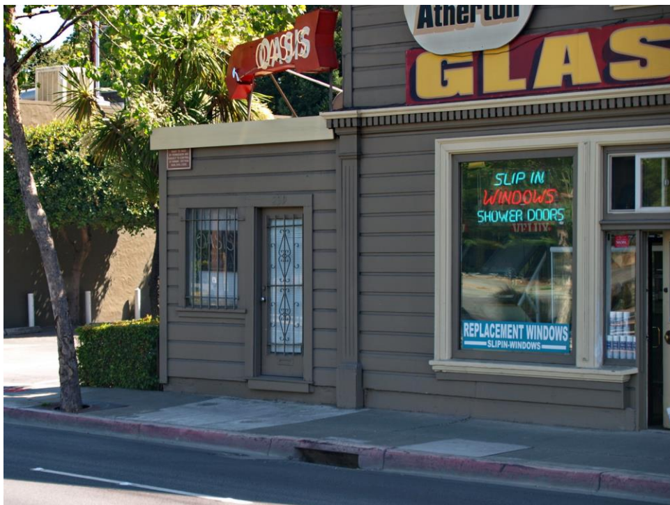
Detail of front façade at office extension, viewed facing south.
