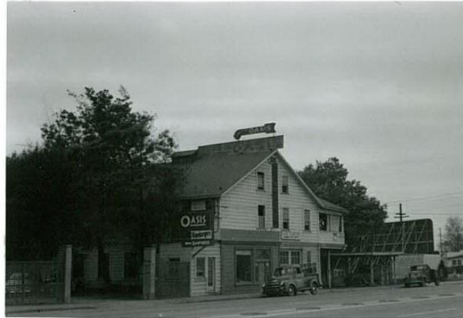
#1 Showing the Oasis building from the South More than 30ft. across driveway.
