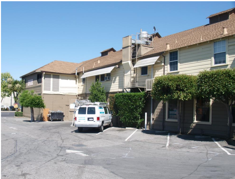
Side elevation from rear of site, viewed facing east.
