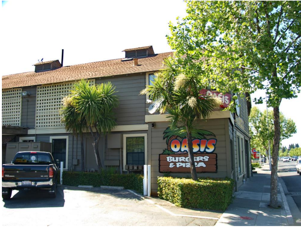
Side elevation at front, viewed facing northwest.
