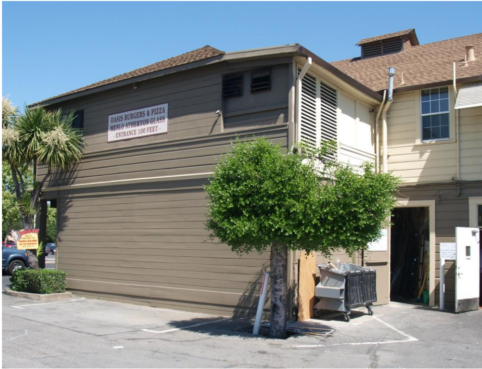
Front side wing, viewed facing east.
