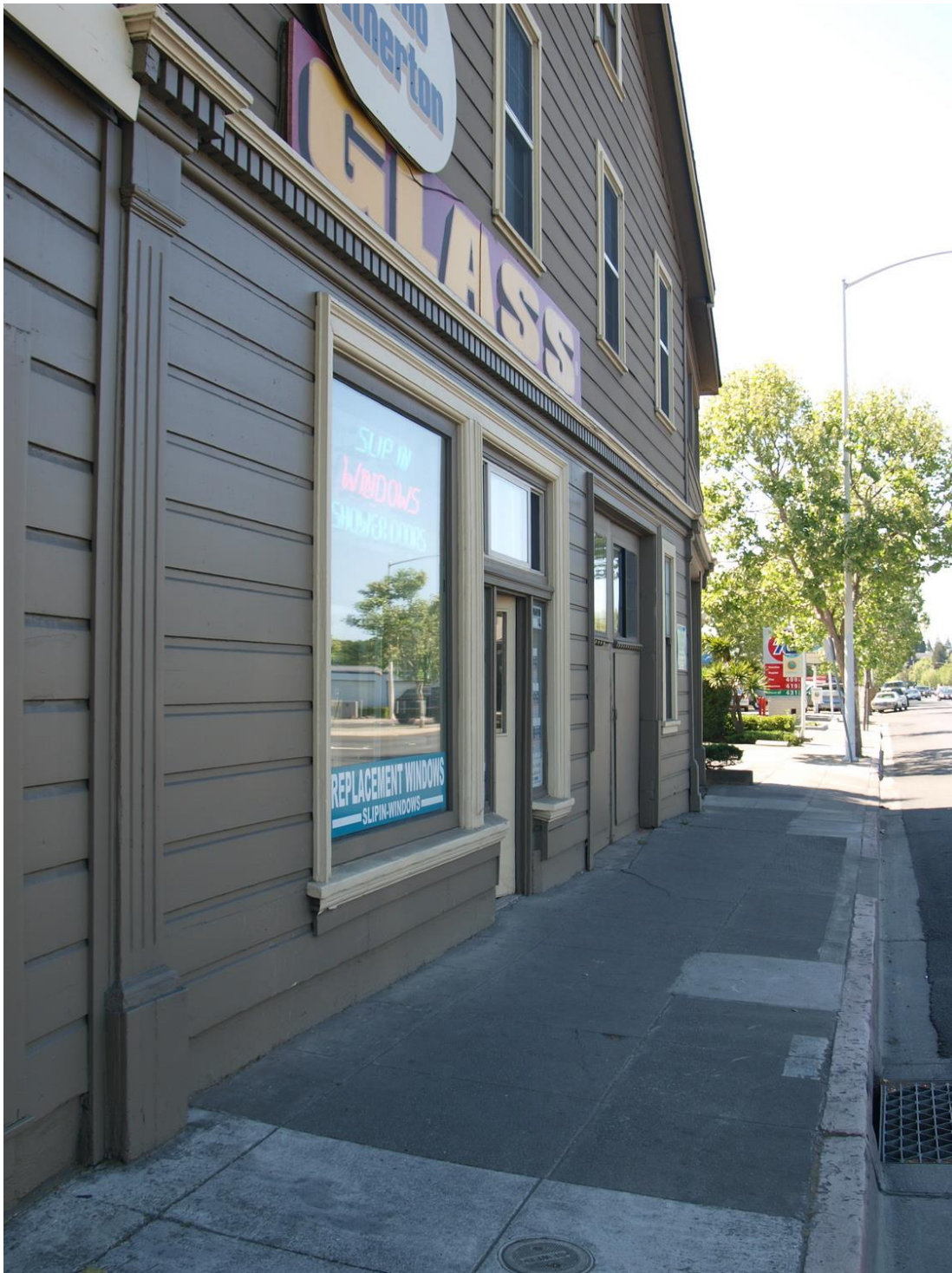
Front façade, viewed facing northwest.
