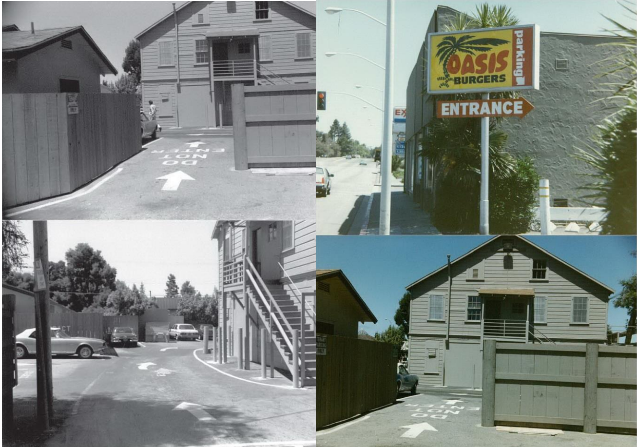
Photos of various elevations of subject property at 241 El Camino Real, Menlo Park, dated 1985. City of Menlo Park Planning File for Property at 241 El Camino Real, Planning Division, Department of Community Development.
