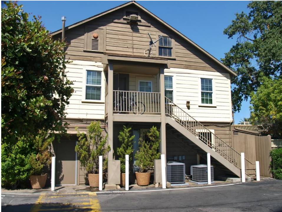
Rear elevation, viewed facing northeast.
