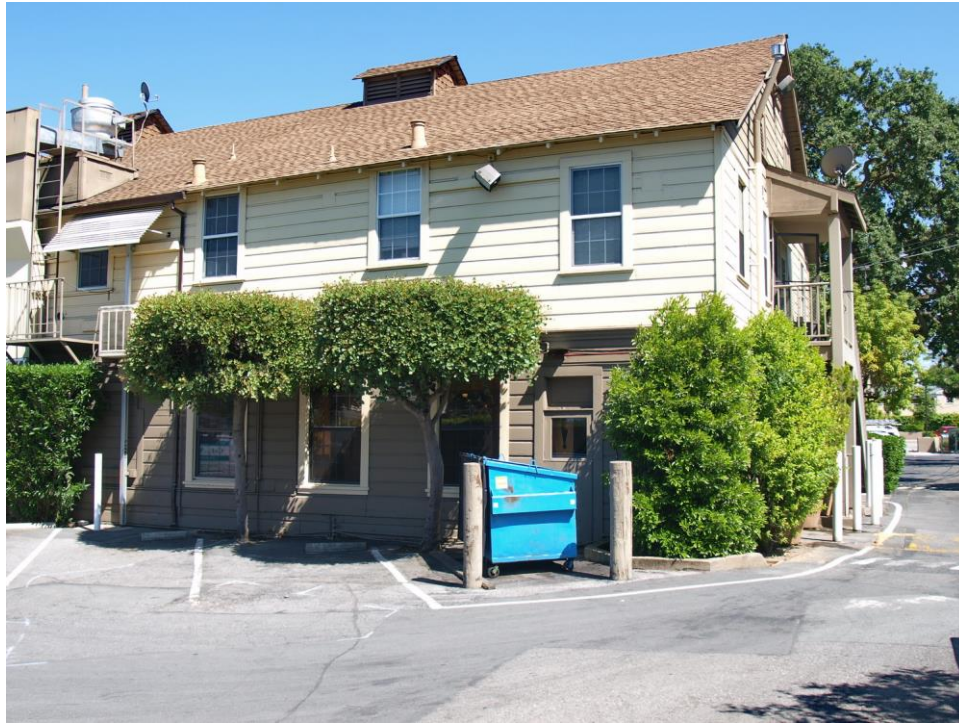
West (rear) corner of building, viewed facing southeast.
