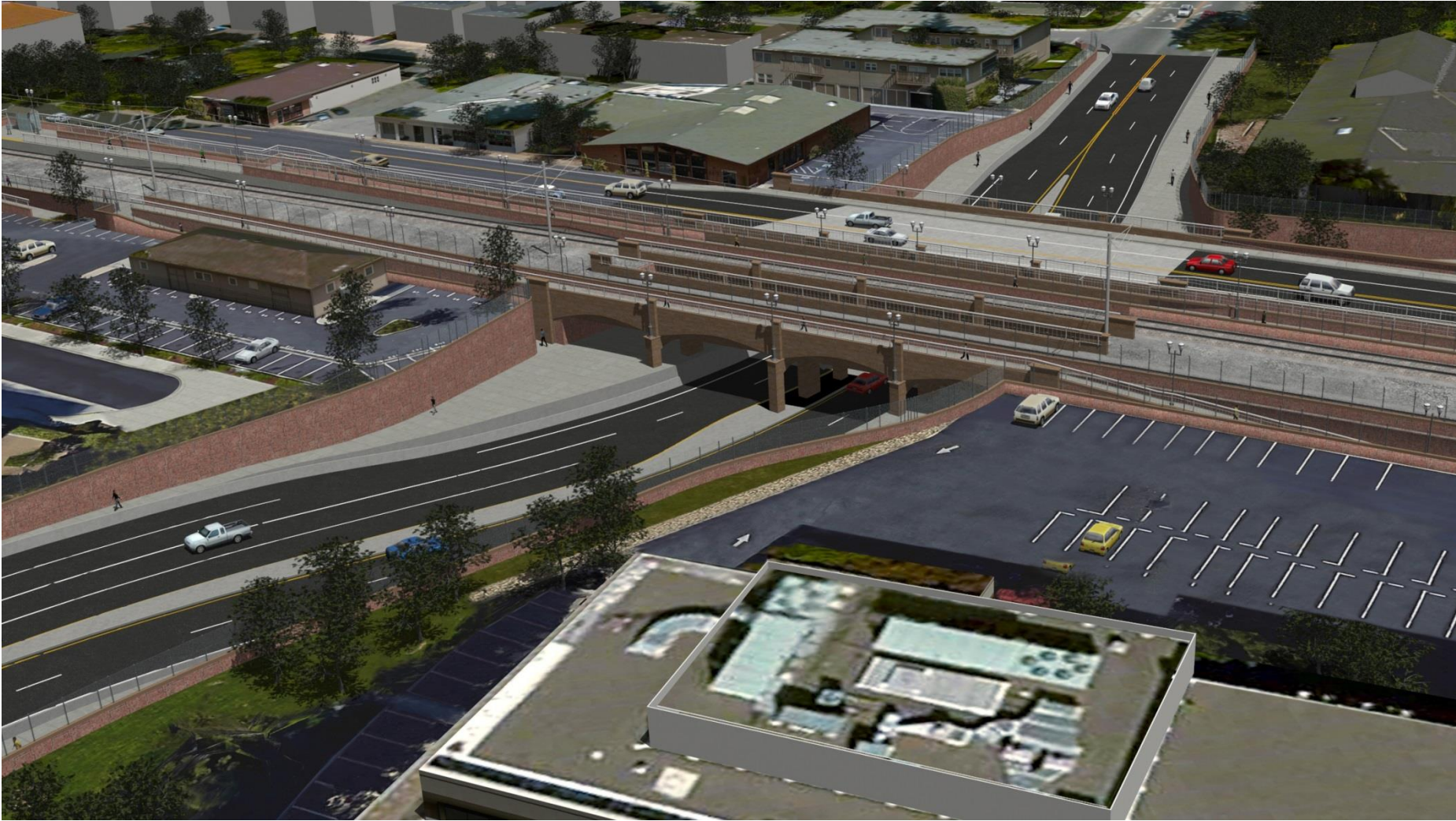
Ravenswood Avenue Railroad Crossing Project
