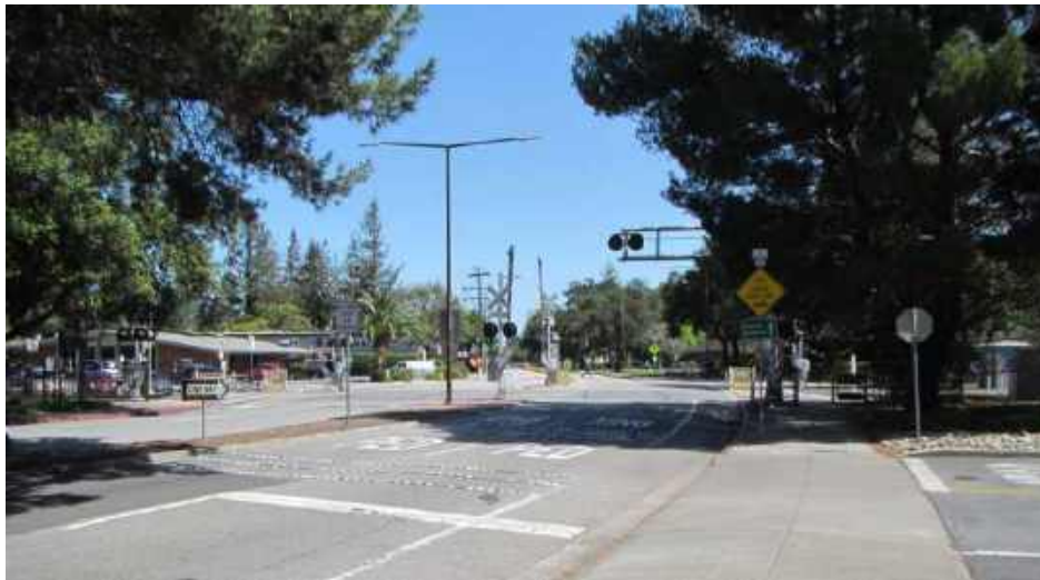
Figure 2. Ravenswood Avenue Rail Crossing, facing East
