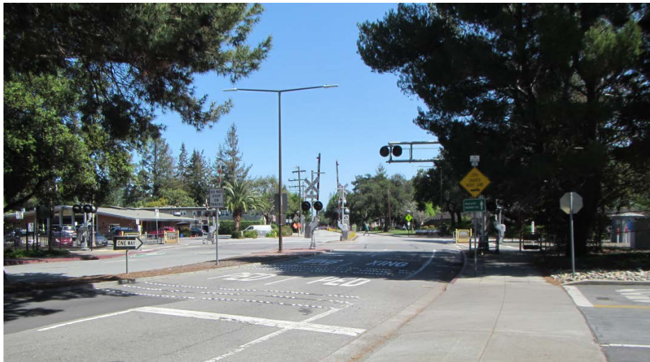
Figure 2. Ravenswood Avenue Rail Crossing, facing East
