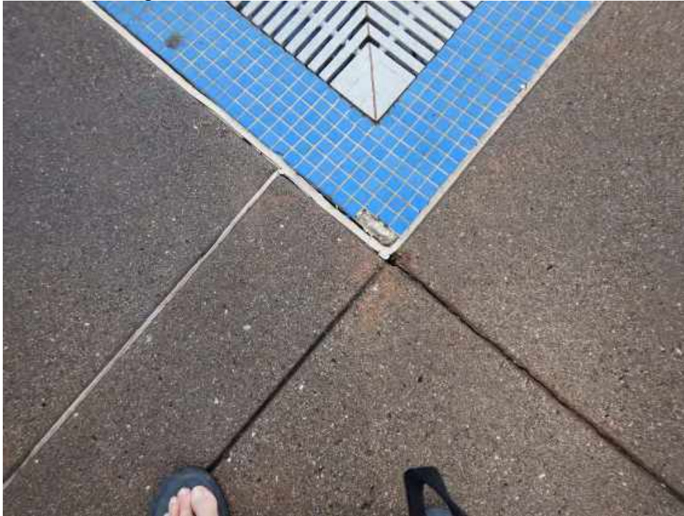
Photos 14 through 17 Perimeter Tiles
