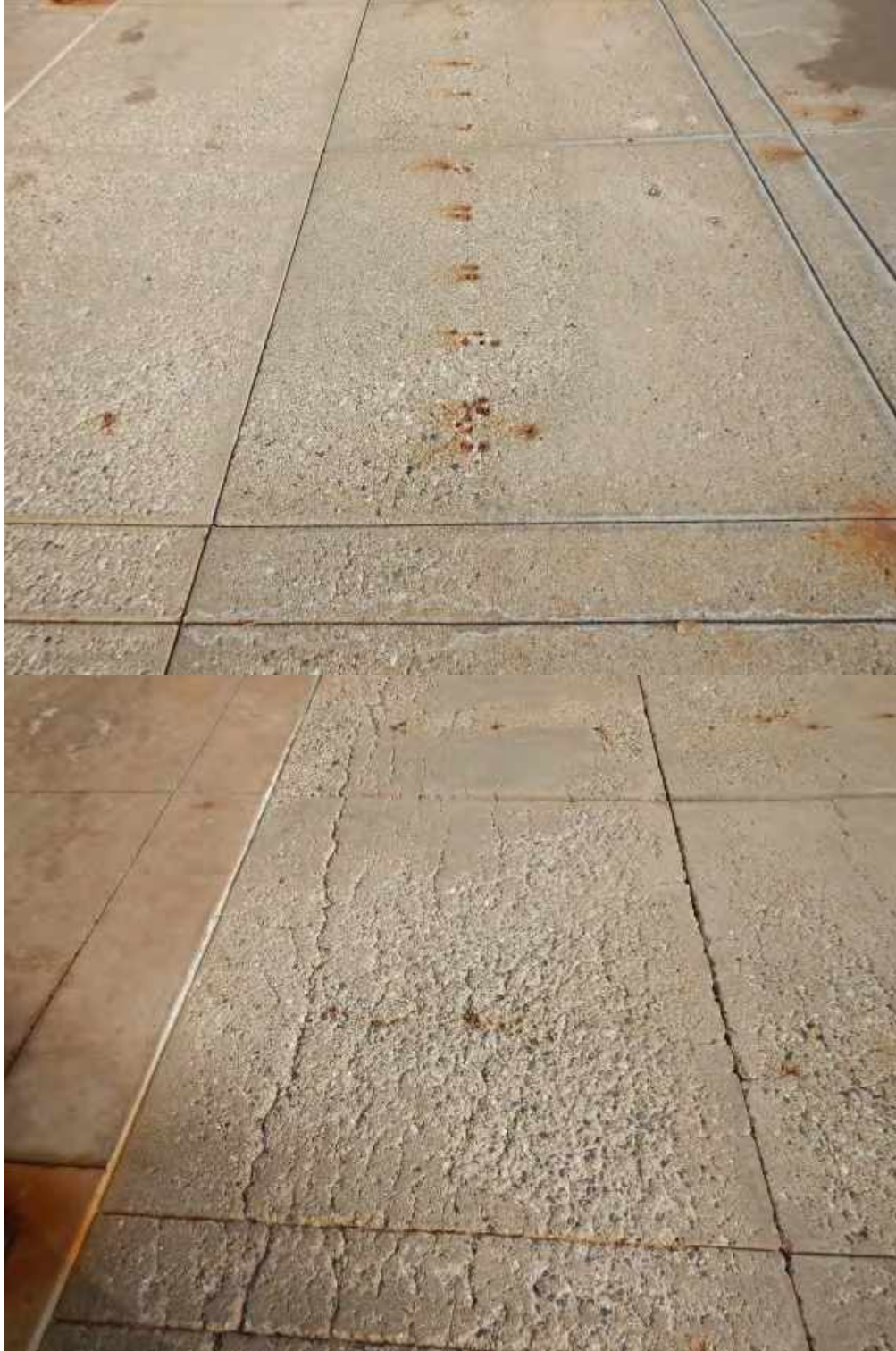
Photos 11 and 12 Expansion joint sealant
