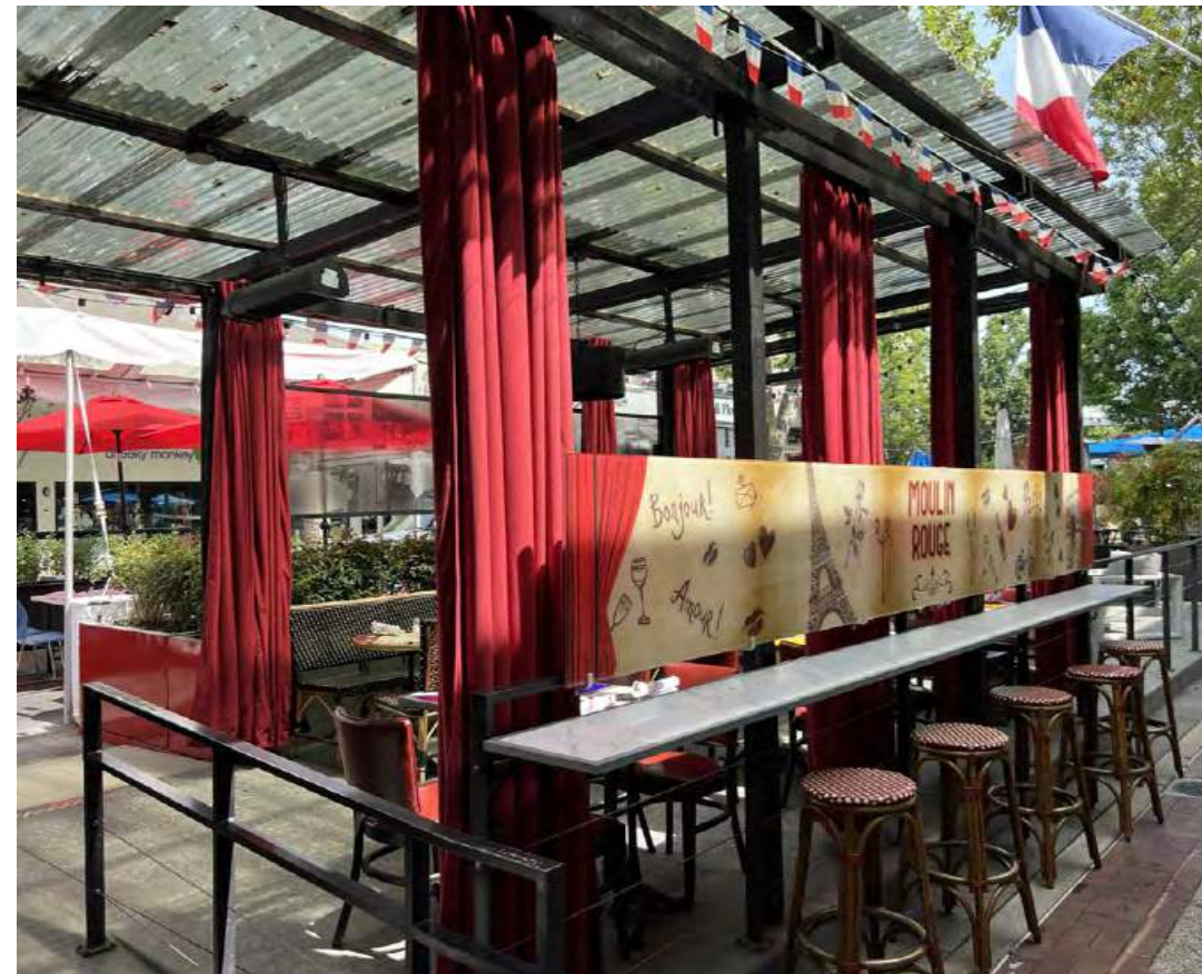
Photo of non-compliant items 1, 2, 3, 4 & 5.
