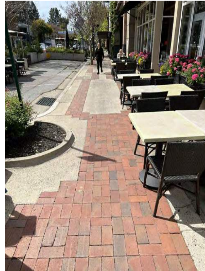
Photo of non-compliant item 5.
