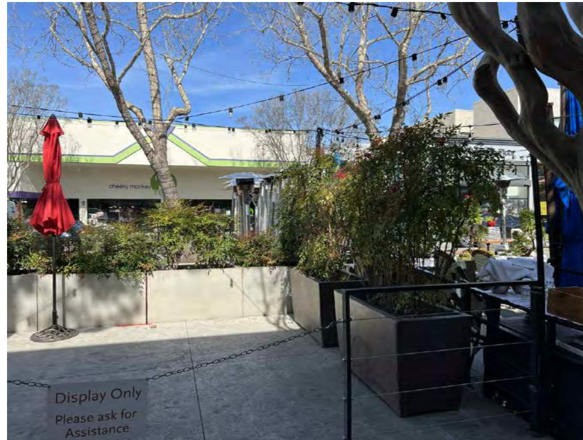
Photo of non-compliant items 1, 3, 4 & 5.
