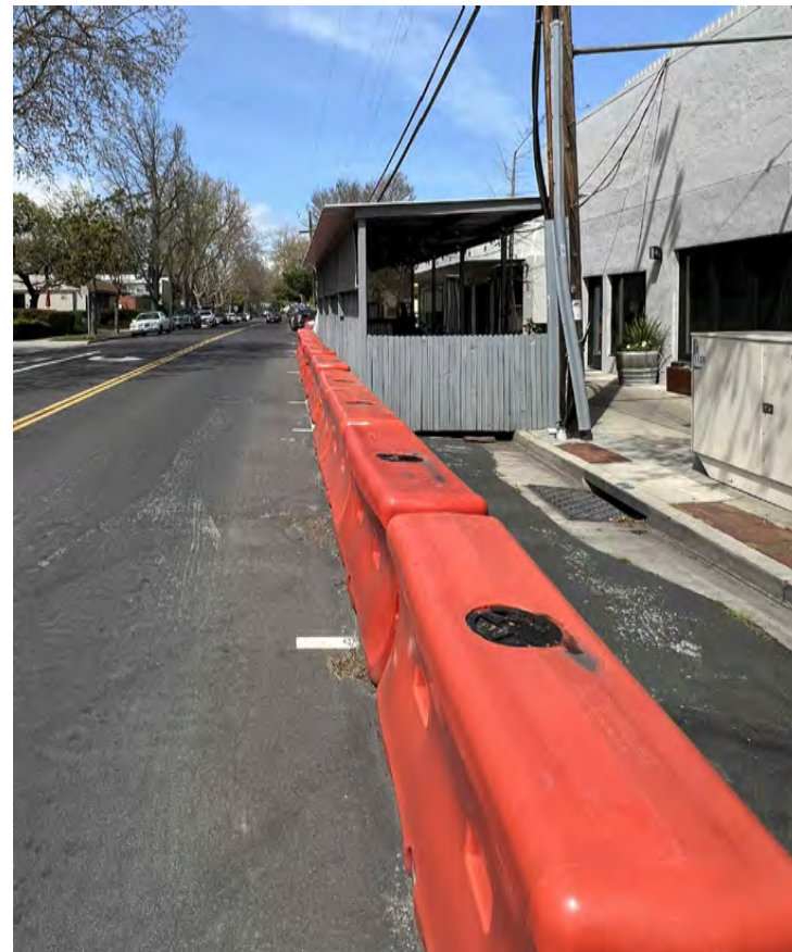
Photo of non-compliant items 1, 2, 3, 4, 5 & 7.
