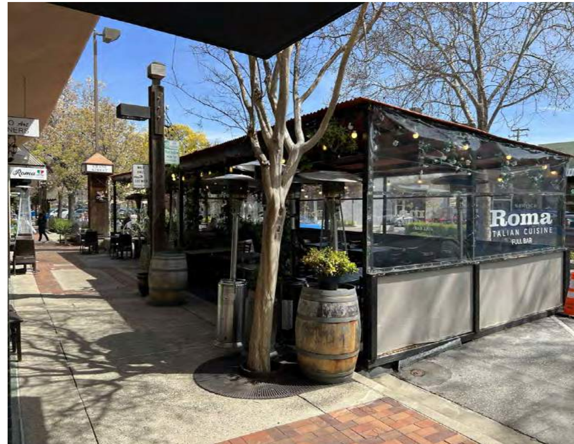
Photo of non-compliant items 3, 6 & 8.
