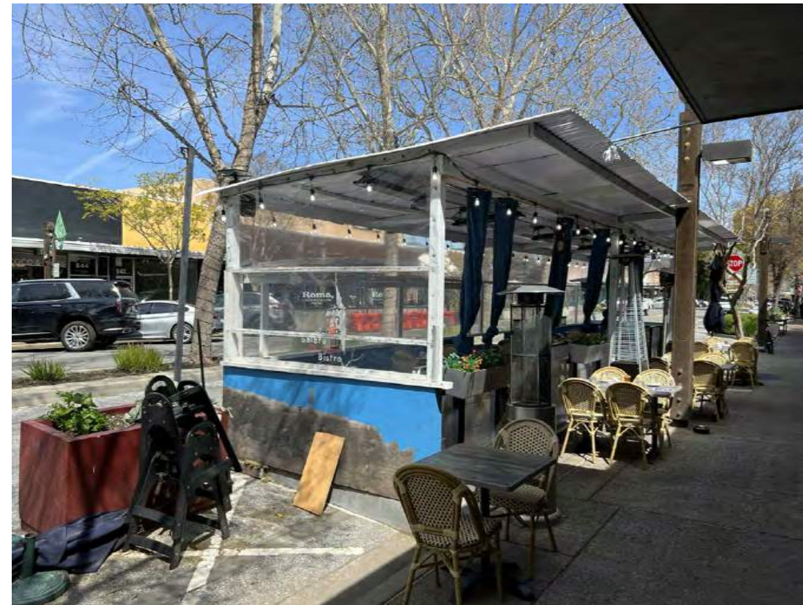
Photo of non-compliant items 4, 5, 6 & 7.
