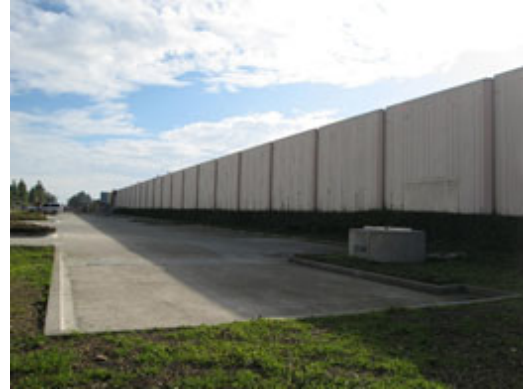
Rear (Easterly) Elevation of 1320 Willow Road
