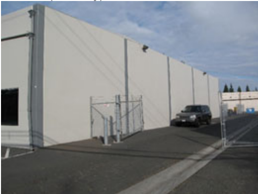
Side (Southerly) Elevation of 985 O'Brien Drive
