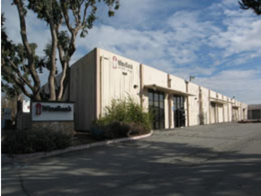
Front View of 1320 Willow Road
