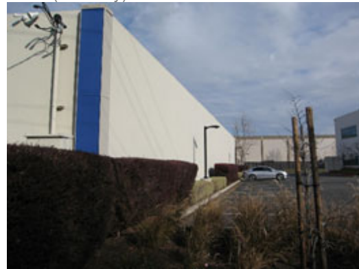
Side (Southerly) Elevation of 1001 O'Brien Drive
