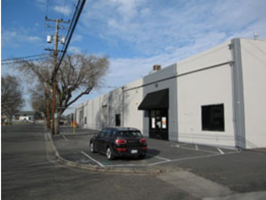
Front (Westerly) View of 985 O'Brien Drive
