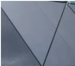
PAINTED ALUMINUM / COMPOSITE CLADDING
