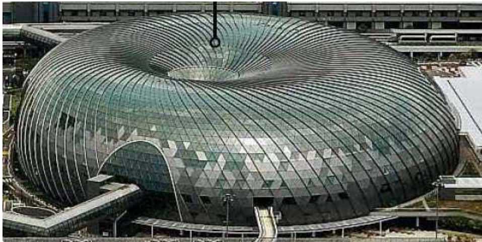
Figure 20. The Jewel Changi Airport building, which has a comparable design and exterior appearance to the proposed atrium. Although extensive vegetation is present inside this building, it is largely invisible from outside the atrium.
