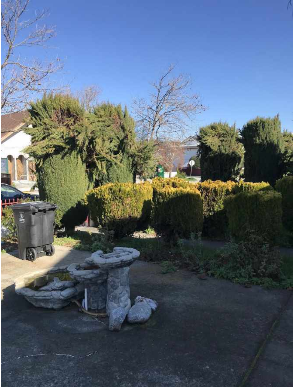
Photo 6. Site of new foundation for ADU, encompassing tree #13 (left) and three (3) small arborvitae.
