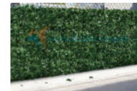
TEMPORARY 6' TALL CHAINLINK FENCING WITH DECORATIVE FENCE WRAP
