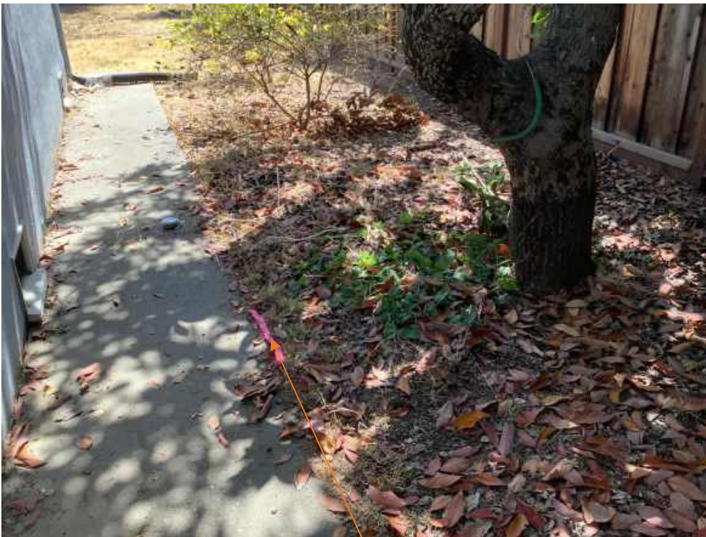
TREE # 3 (TAG # 5276): EXPECTED EXTENT OF EXCAVATION FOR FOUNDATION
