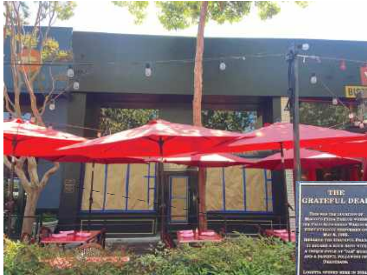
FULL FRONT FACADE
