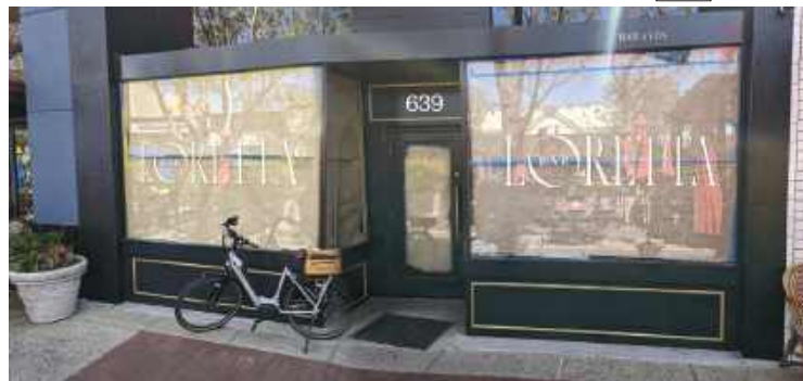
LOWER FRONT FACADE
