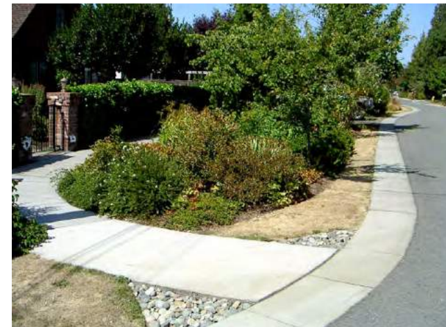
Sidepath in Seattle with Green Stormwater Infrastructure integrated.
