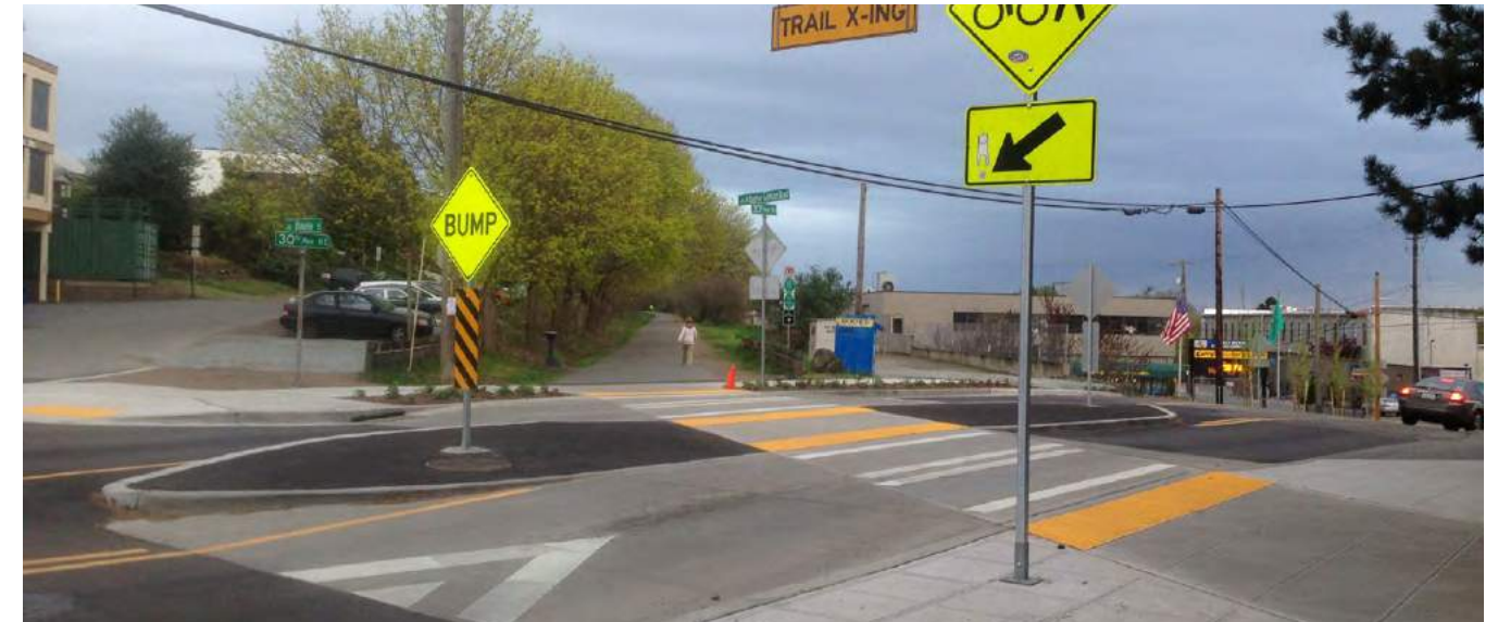
This raised path crossing encourages drivers to yield to pedestrians and allows bicyclists to cross traffic one lane at a time.
