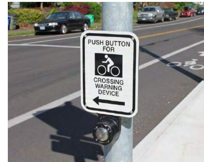
Bicycle push button actuators are positioned to allow bicycle riders in roadway to stop traffic on busy cross-streets.
