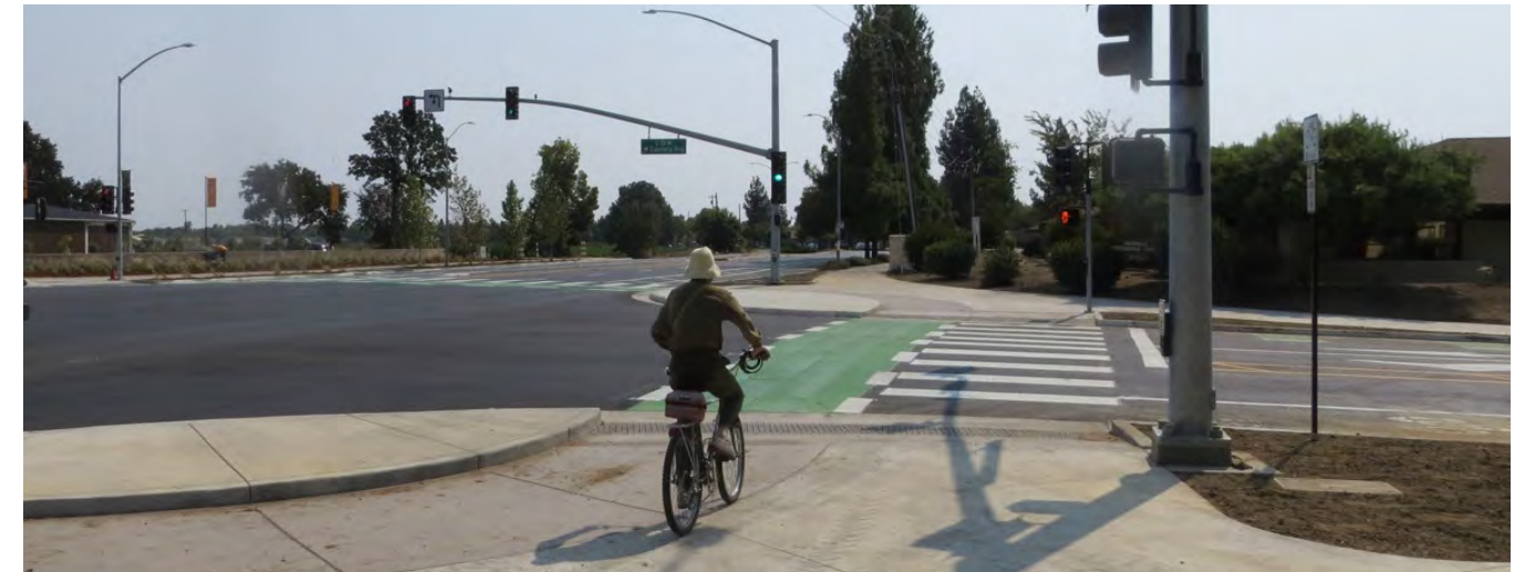
Protected intersections feature a corner safety island and intersection crossing markings, and can be used by bicyclists to queue for two-stage left turns.
