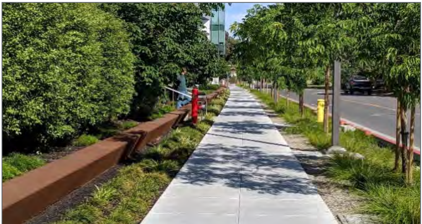
Green infrastructure, such as the bioswales along the Menlo Gateway site at Independence Drive, provides a cost effective approach to managing stormwater as part of roadway design.
