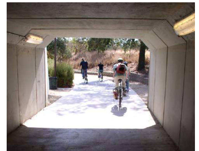
Grade-separated crossings help people walking or biking cross barriers such as freeways, railroads, and rivers.
