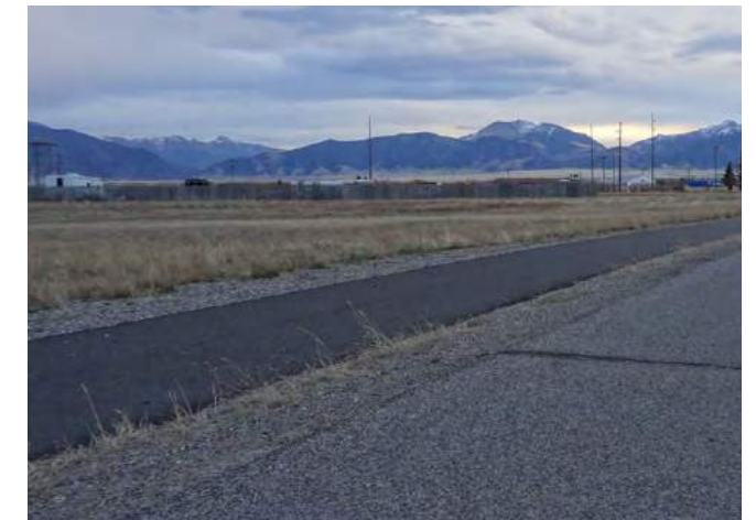
Sidepath with gravel separation.
