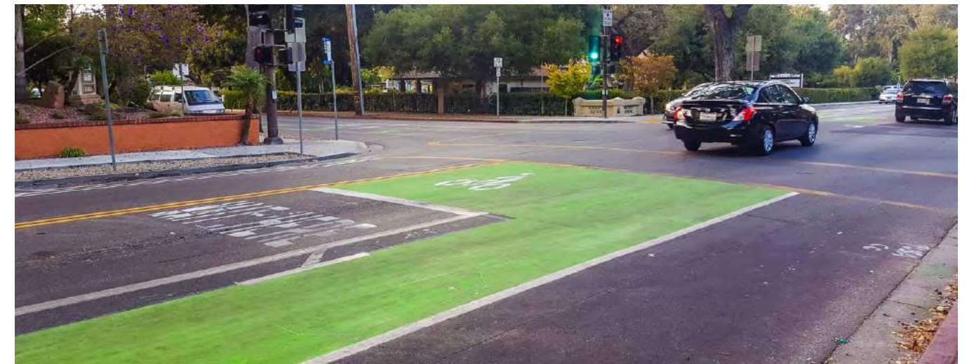
The use of colored pavement helps denote conflict zones where motorists crossing the bike lane must yield.
