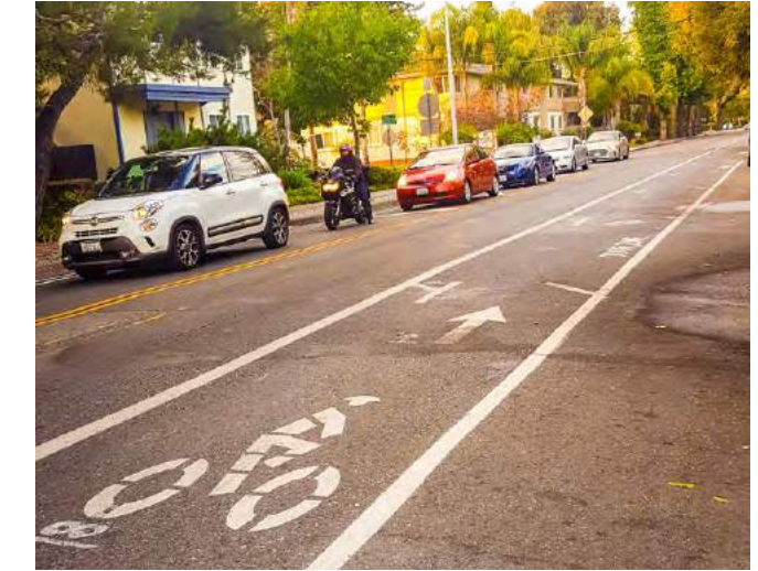
The use of pavement markings delineates space for cyclists to ride in a comfortable facility.
