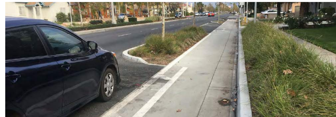
Street Level Separated Bikeways can be separated from the street with parking, planters, bollards or other design elements.
