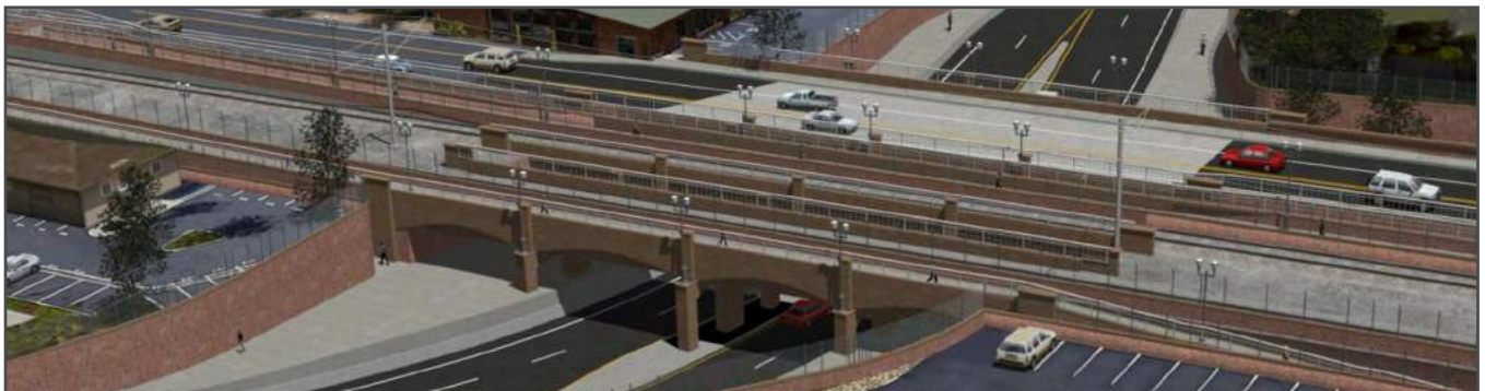
The City of Menlo Park supports replacing at-grade Caltrain crossings with grade-separated crossings at Ravenswood, Oak Grove and Glenwood Avenues. This visualization shows the proposed grade separation looking east along Ravenswood Avenue.
