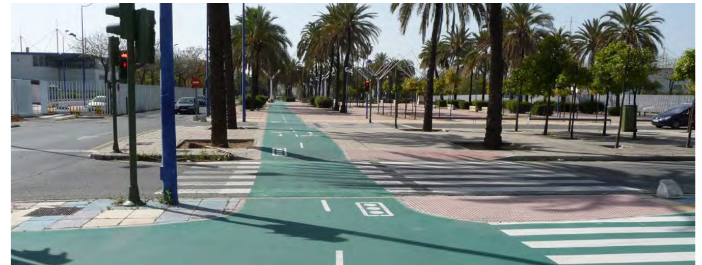
Raised separated bikeways are bicycle facilities that are vertically separated from motor vehicle traffic.
