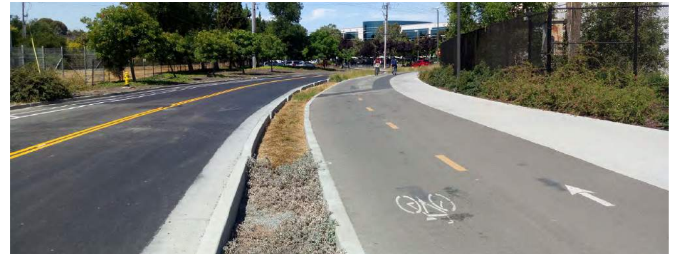
A two-way facility can accommodate cyclists in two directions of travel.
