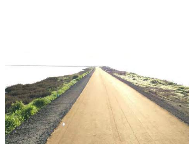
Decomposed granite on San Francisco Bay Trail as an alternative to paved paths.
