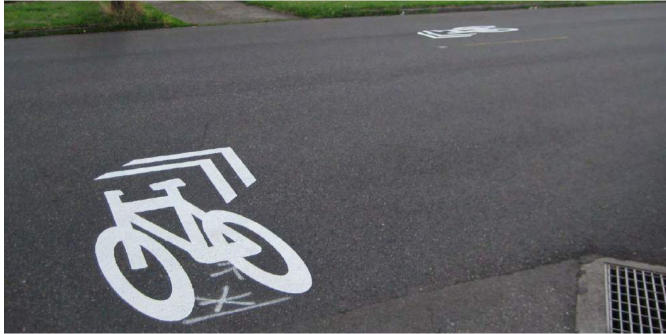
Some cities use pavement markings to indicate required turns or jogs along the bicycle route.
