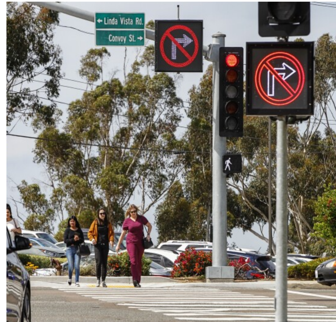
Blank out sign Used to restrict turning movement conflicts between turning vehicles and bicycles/pedestrians
