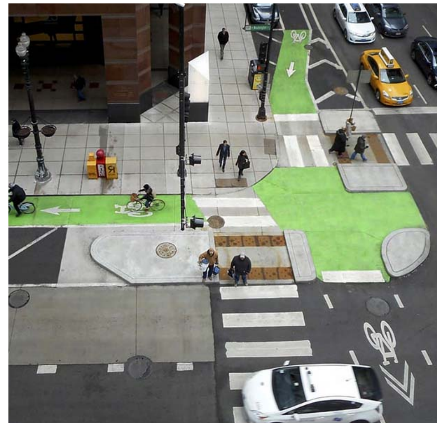
Protected Intersection Provides separate path of travel for bicyclists, improving visibility and reducing crossing distance
