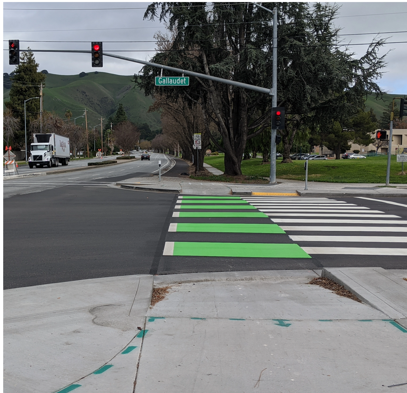
Intersection Crossing Marking Increases the visibility of bicyclists, raising awareness of potential conflict areas
