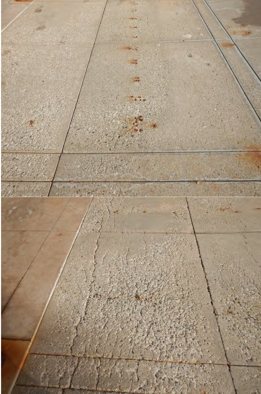
Photos 11 and 12 Expansion joint sealant
