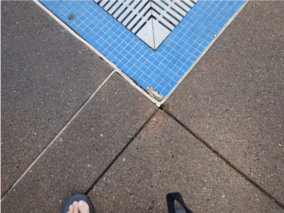
Photos 14 through 17 Perimeter Tiles
