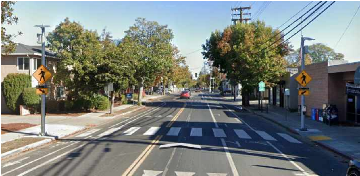
Rectangular rapid flashing beacons (Oak Grove Ave. – Menlo Park)
