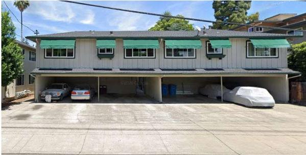
Figure 1 Example of a four-unit, soft-story building
