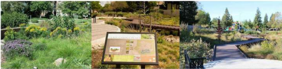
RAIN GARDEN/ STORM WATER TREATMENT
