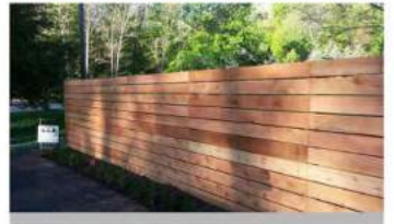
PERIMETER FENCE 72" TALL HORIZONTAL WOOD PLANKS
