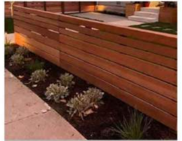
PATIO FENCE 42" TALL HORIZONTAL WOOD PLANKS
