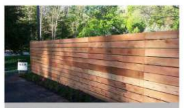
PERIMETER FENCE 72" TALL HORIZONTAL WOOD PLANKS
