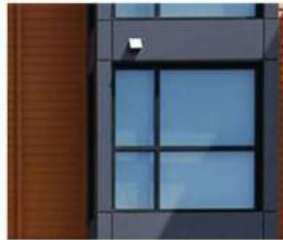
W1 VINYL WINDOW VPI QUALITY WINDOWS BLACK FRAME FINISH OR SIMILAR BY ALTERNATIVE MANUFACTURER
