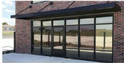
W2 STOREFRONT ALUMINIUM STOREFRONT BLACK FRAME FINISH
