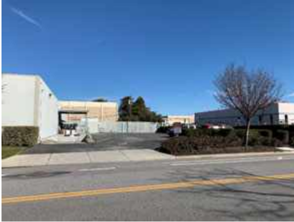
Photo 1. The project site consists of a commercial building surrounded by hardscape with narrow, interrupted areas of landscaping.
