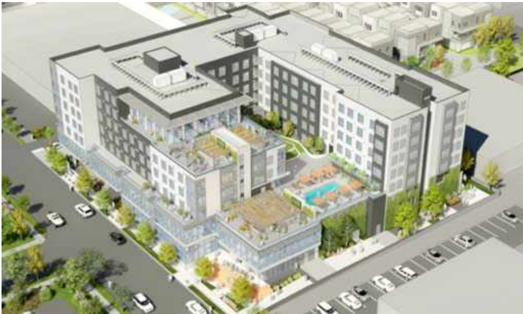
Figure 2. The proposed building incorporates opaque wall panels, overhangs, and window mullions. These features help the building appear as a solid structure to birds, and reduce the likelihood of collisions.
