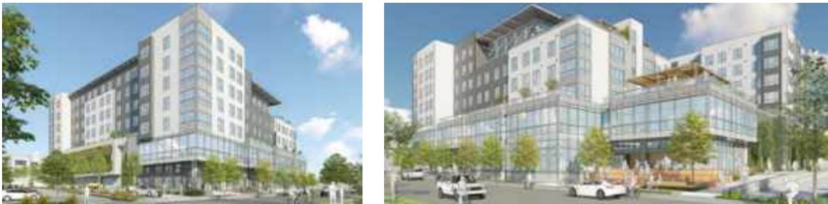
Figure 3. Southwest (left) and southeast (right) building perspectives. The facades of Levels 1 and 2 are predominantly glazed on the south façade and its adjacent corners. Freestanding glass railings are present on all rooftop terraces.
