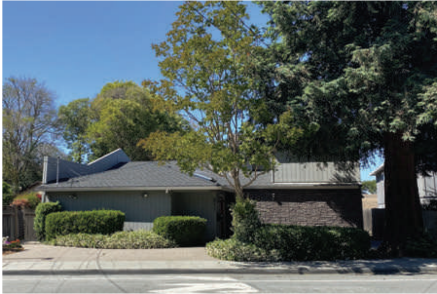
811 BAY ROAD, FRONT / SOUTH ELEVATION ⑥
