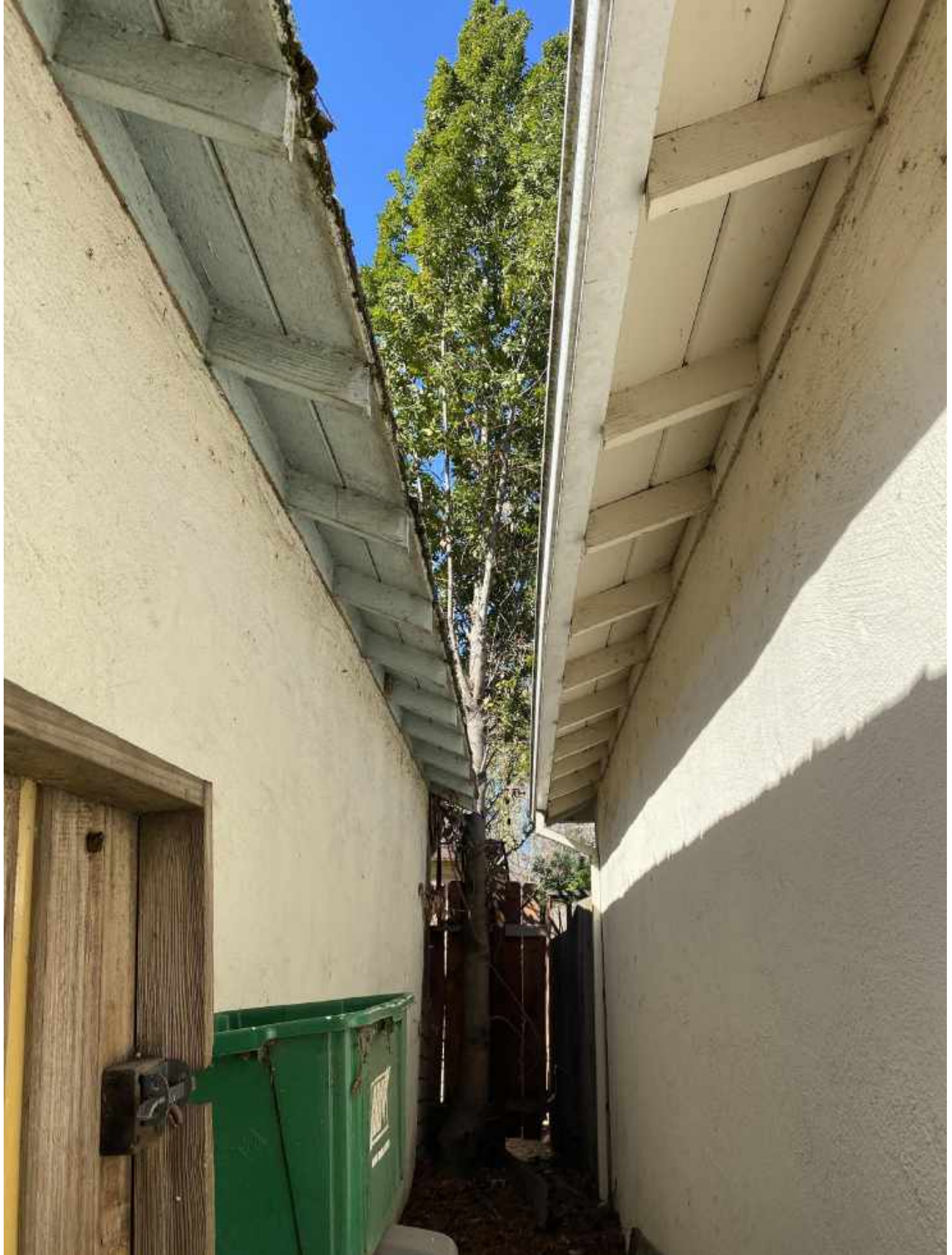
Photo 4. View of tree #3. Due to its poor location and potential impacts from demolition of the building on the left, removal is necessary.
