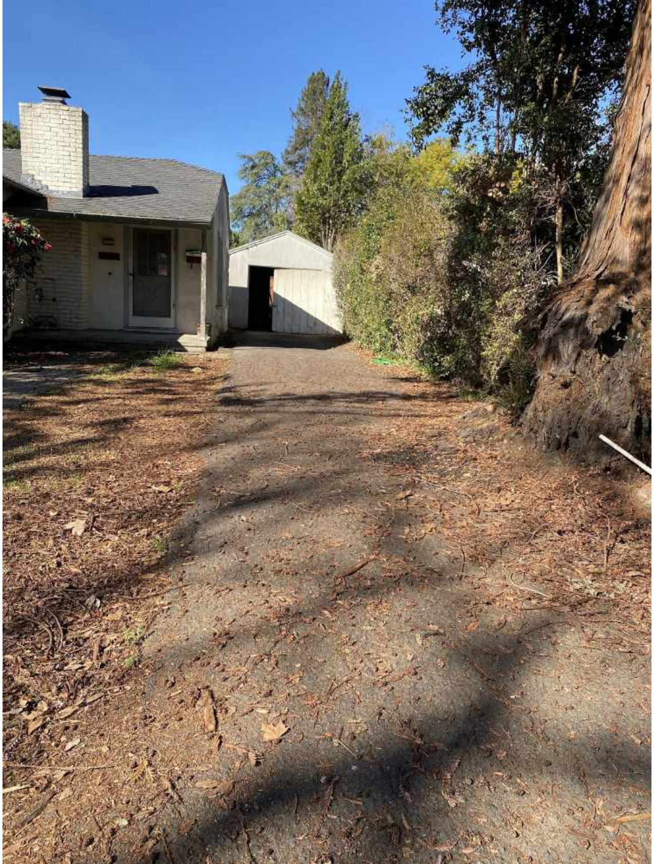
Photo 3. Shown of the right side of the photo, tree #1 has grown over the existing driveway. Care and attention to preconstruction planning are essential to reduce impacts to the TPZ of this tree.
