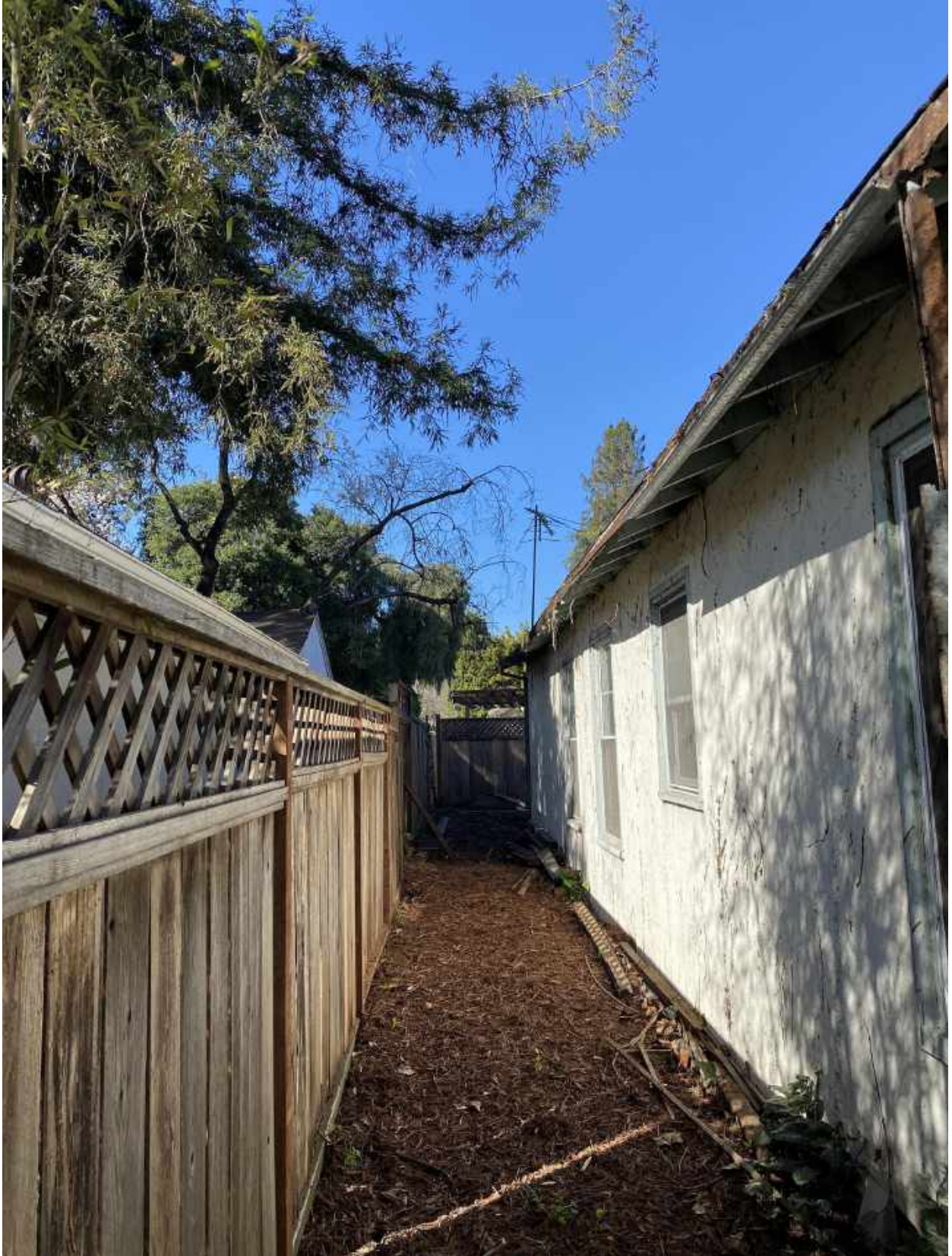
Photo 8. View along the south fence line. The canopy of tree #5 (seen in the background with leafless branches) overhangs the property fence. The portion of the canopy that overhangs the property line is dead. Pruning of deadwood is recommended.
