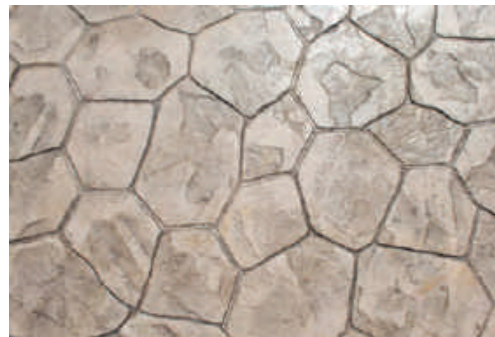
PAVEMENT NODE - STAMPED CONCRETE
