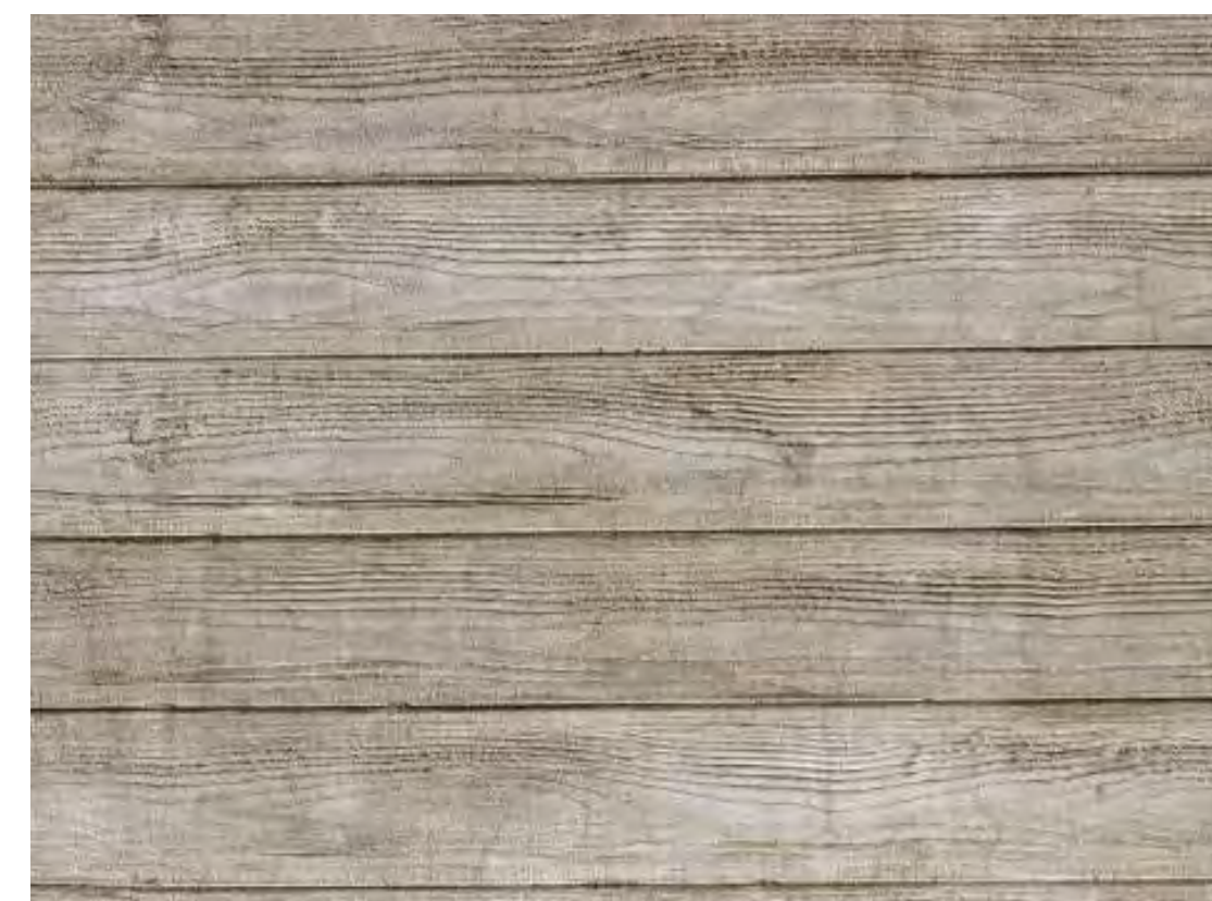
PAVEMENT NODE - STAMPED CONCRETE
