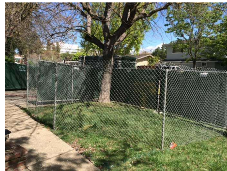
Figure 5: Example of Tree Protection Fencing
